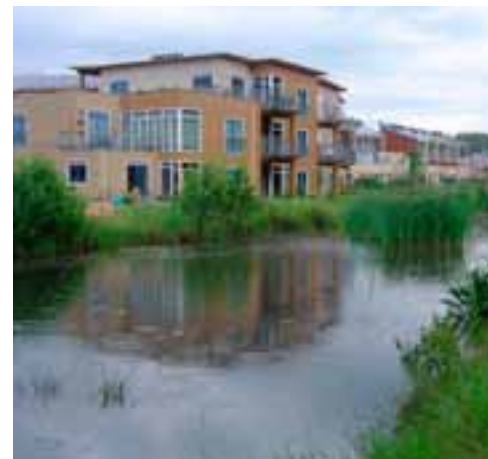
A constructed wetland created to collect the stormwater from the district and provide an amenity for the community
