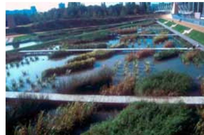
A constructed wetland created to collect the stormwater from the district and provide an amenity for the community
