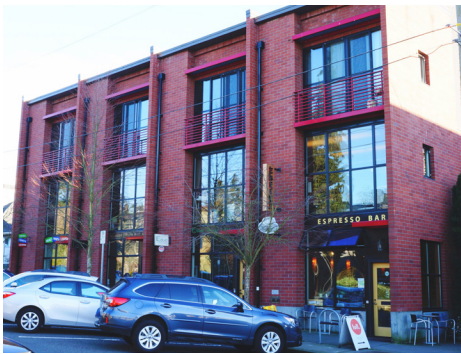
Live-work units designed for commercial uses at grade, with living spaces above.
