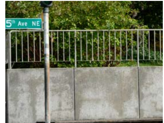
Retaining wall along 15th Avenue at 43rd Street.
