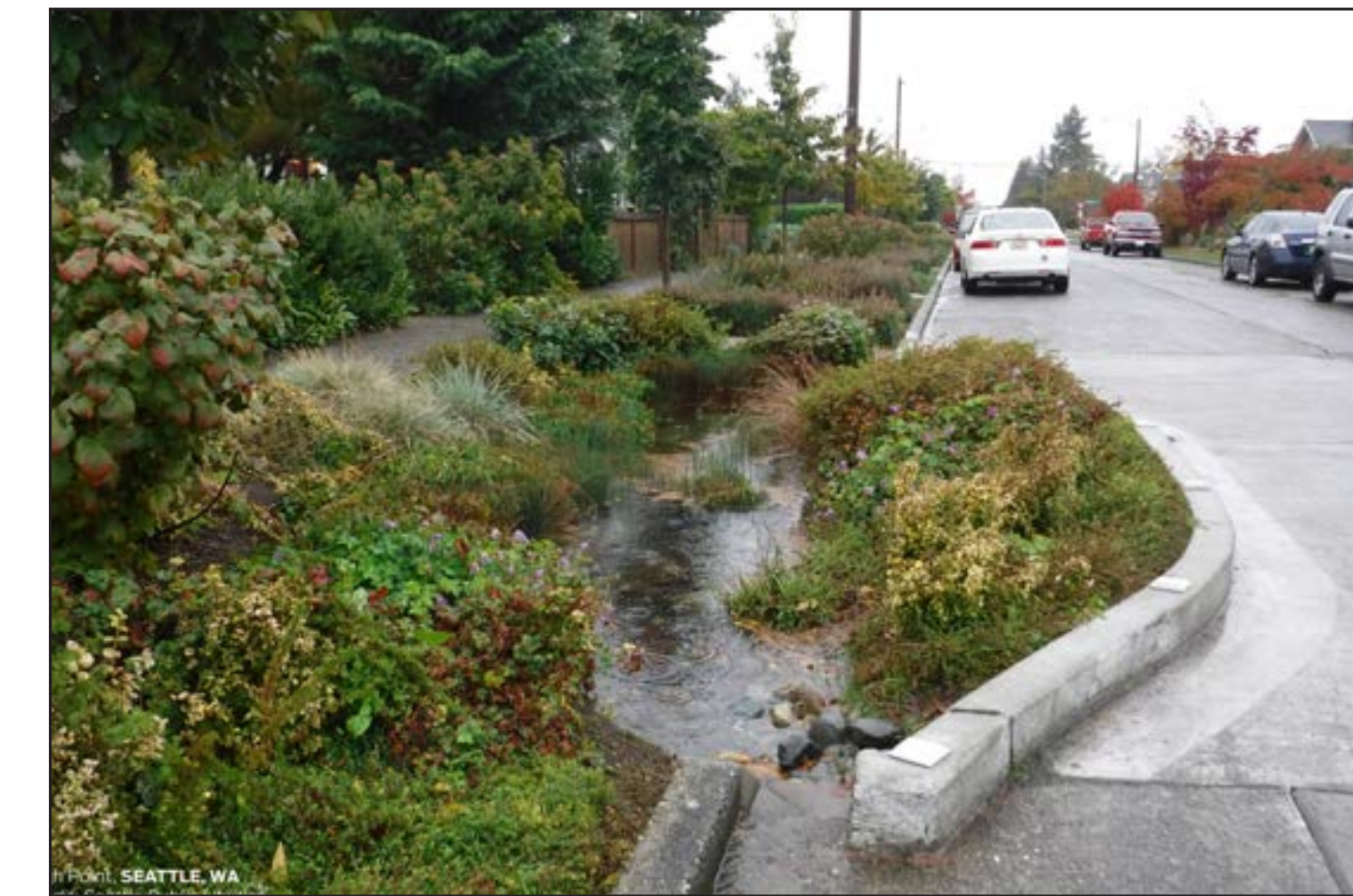
Green Stormwater Infrastructure at High Point
