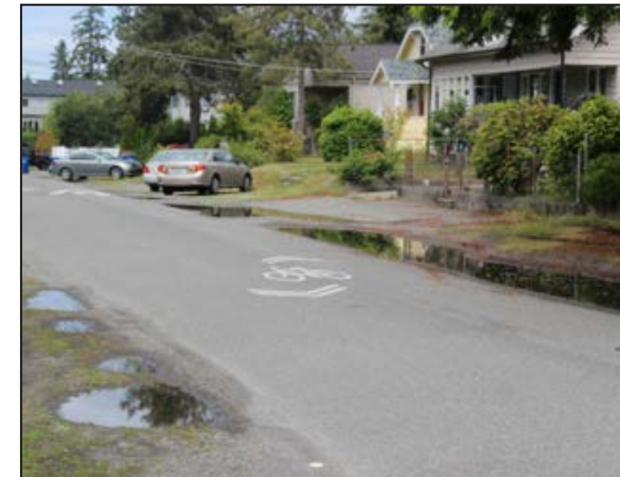
Drainage issues in Crown Hill
