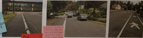
Traffic Calming Device Roadway features
