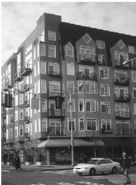
the roofline of this building adds to the structure's residential identity
