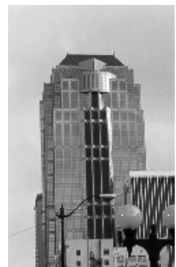
a sculpted form is carried up the building to the distinctive treatment of the rooftop
