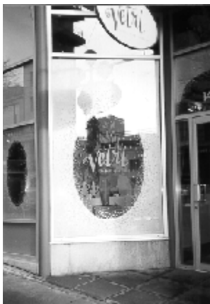
signage at the sidewalk level
