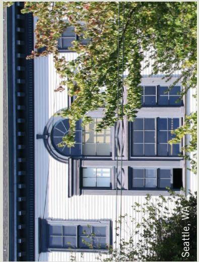
Cornice with brackets and dentil moldings, painted wood siding, contrasting wood trim, classical window composition with arch, keystone, and pilasters.
