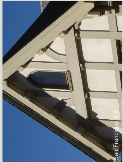
Steeply-pitched gable end with eaves supported by brackets and half-timber detailing.
