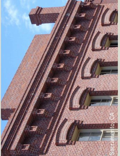
Clearly defined top with a continuous cornice and parapet, jack arches over vertical window openings, and corbeled brackets.
