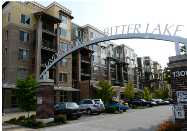
Linden Place includes 751 low-income senior and family apartments in two buildings
