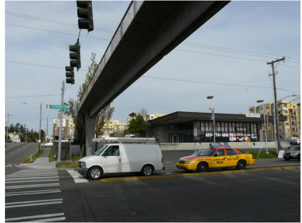
Figure 19 - Existing development at the northwest corner of Aurora and N 130th St.
