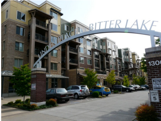
Figure 5 - This Development along Linden Place includes 391 low-income senior and family apartments in two buildings.
