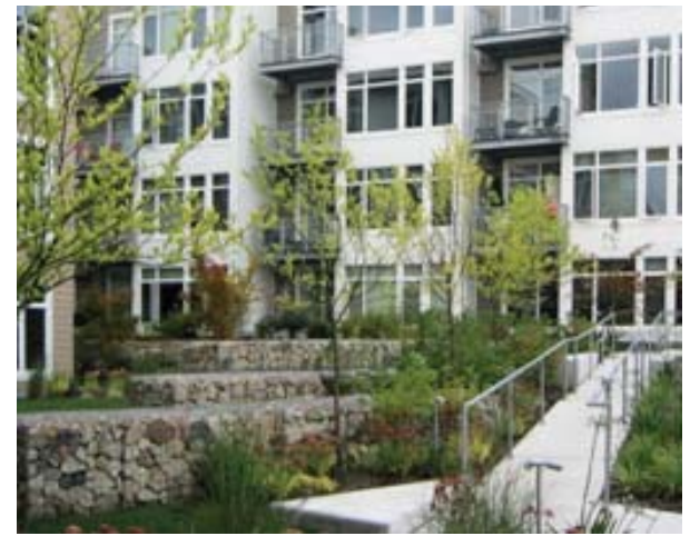
A residential courtyard
