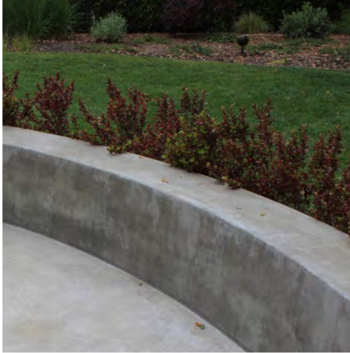
CONCRETE SEAT WALL
