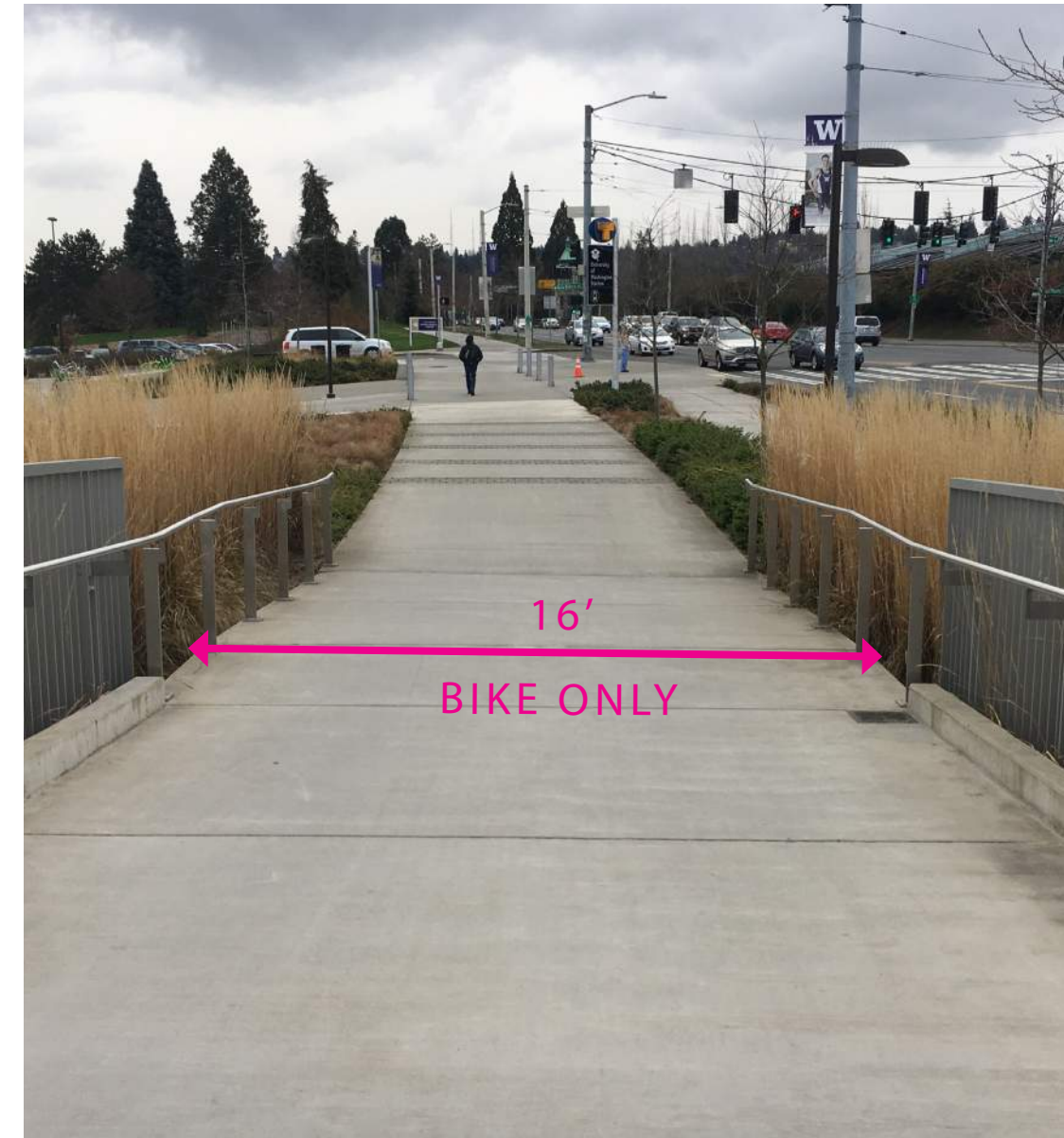
Bicycle Ramp at ST Station/Montlake Triangle
