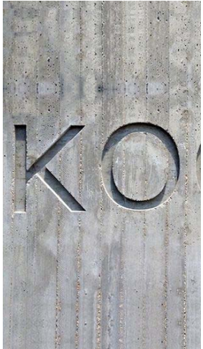
Articulated Concrete Formwork
