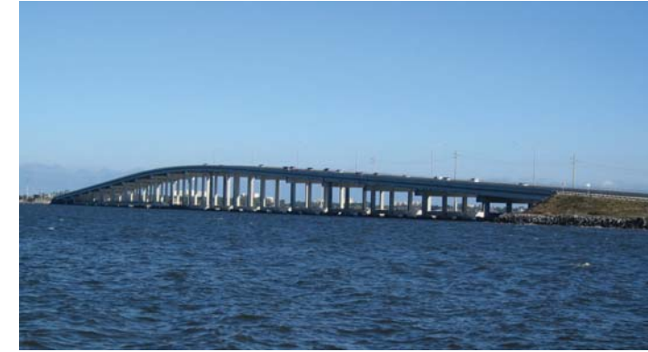
Eau Gallie Causeway Eau Gallie, Florida
