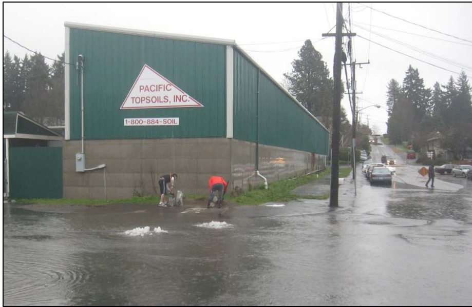
Stormwater surging out of inlets
