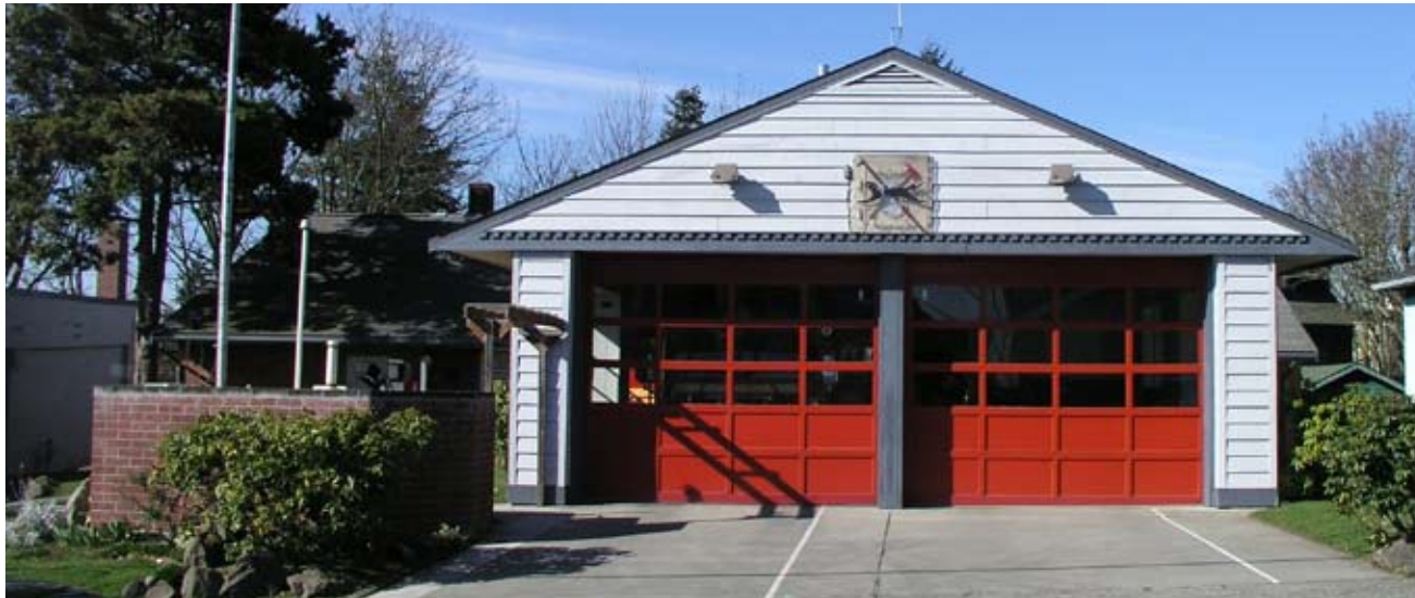
Fire Station 9 built circa 1952, a modern post-war design
