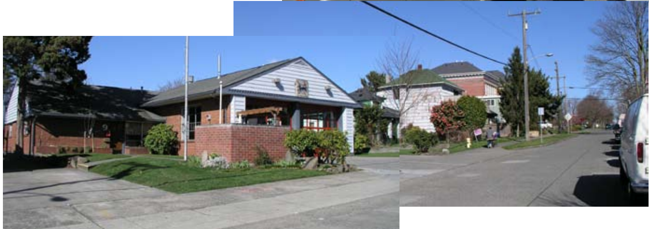
looking west to Fire Station 9 site & adjacent buildings
