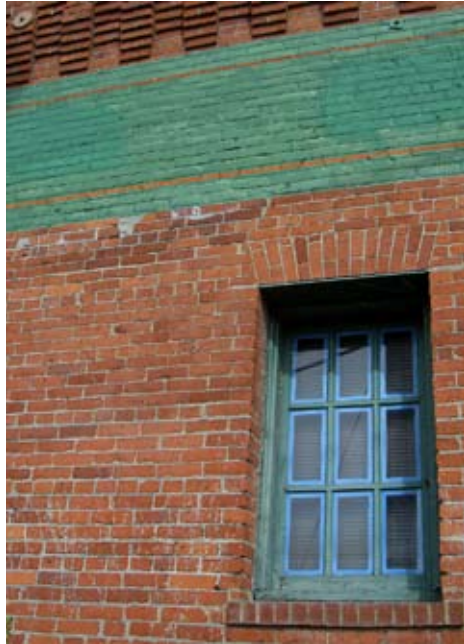
Brick coursing detail in Fremont commercial area
