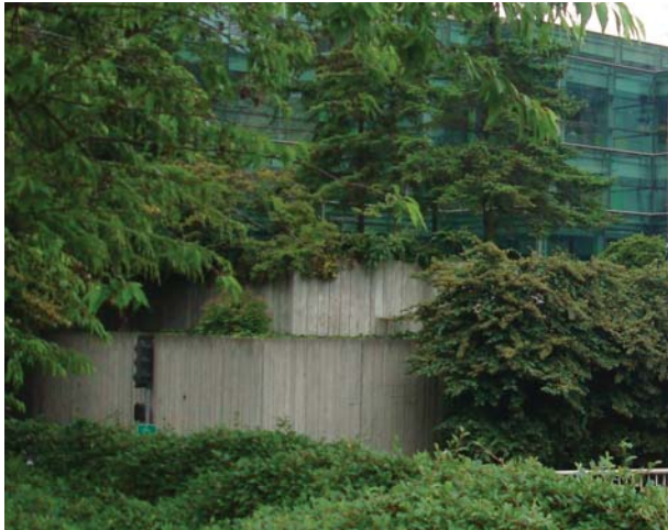
vegetated retaining walls
