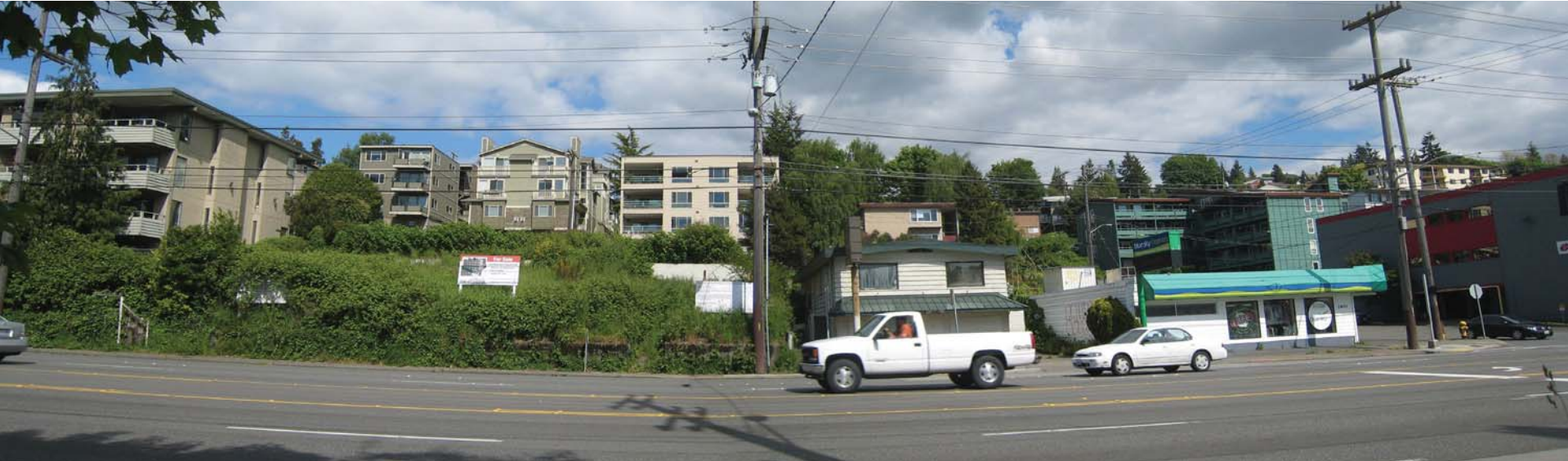
15th Ave West looking across to Fire Station 20 site
