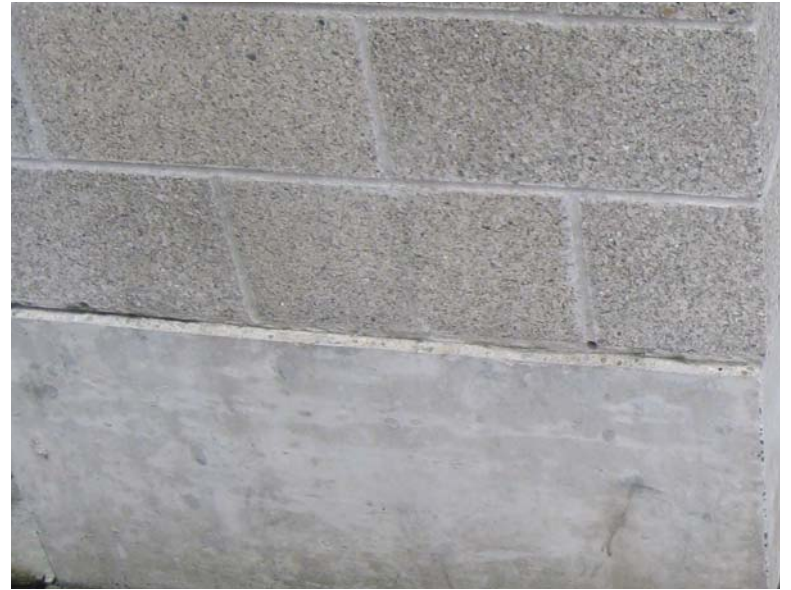
ground - face cmu with cast concrete below
