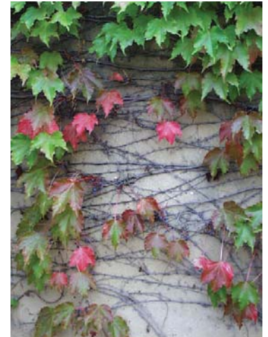
vegetated retaining walls
