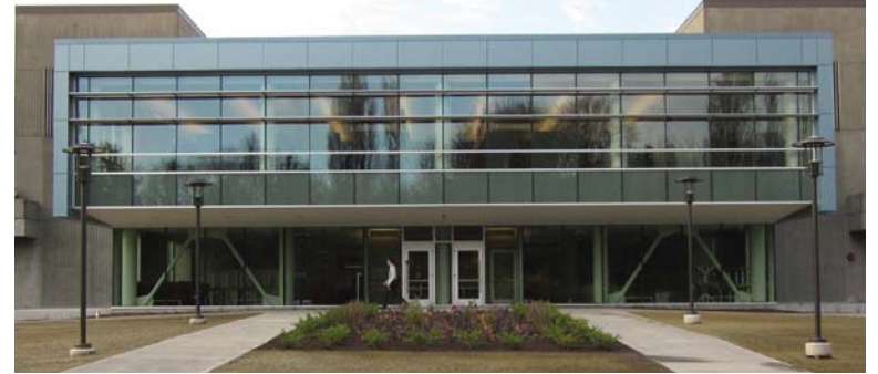
structural silicon glazed curtainwall lower spandrel panel
