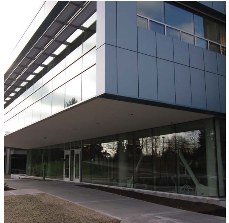
structural silicon glazed curtainwall with metal panel infill
