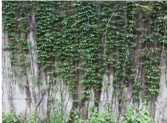
vegetated retaining walls
