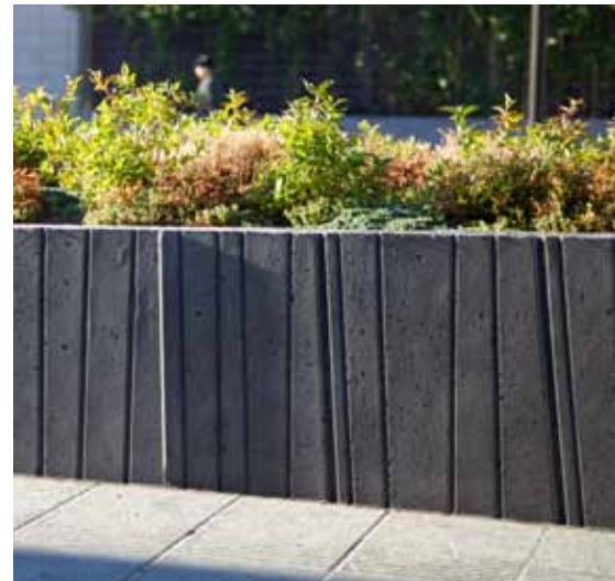
Dark concrete formliner walls around campus perimeter
