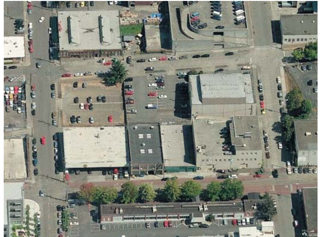
Aerial View from the West
