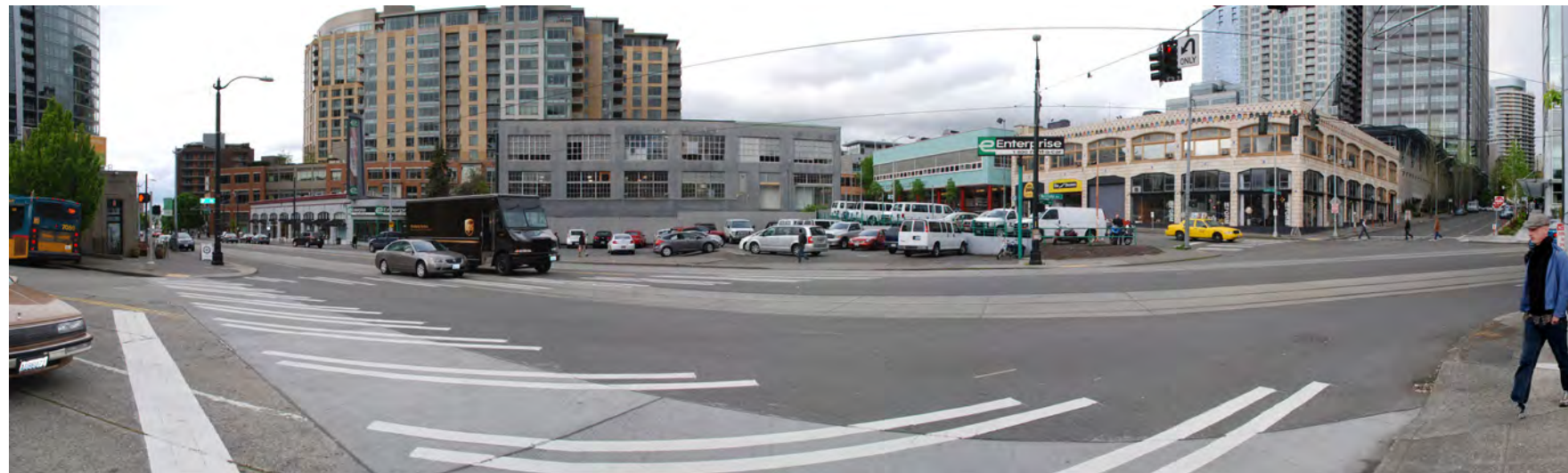
Existing Conditions @ 8th Ave, Lenora St and Westlake Ave
