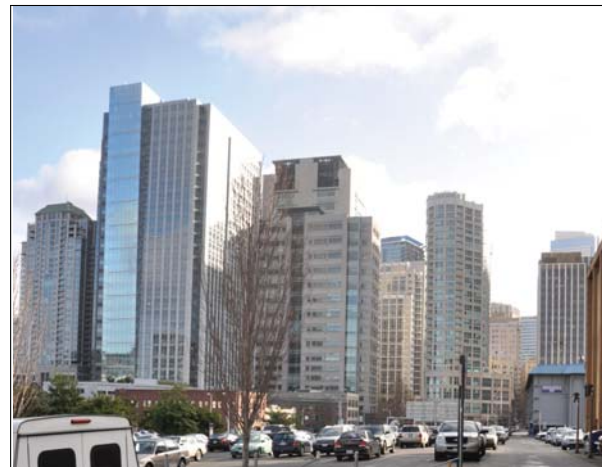
L to R: Cosmopolitan Condo Tower, West 8th office building, U.S. Federal Courthouse, 1700 7th Ave office building, Metropolitan Condo Tower • Variety in tower shape and surface expression • Stepped form
