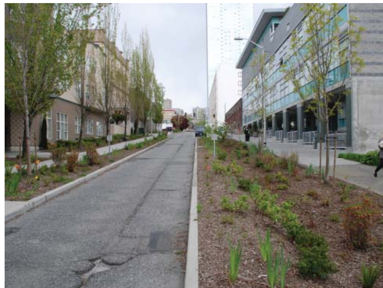
Terry Avenue Rain Gardens
