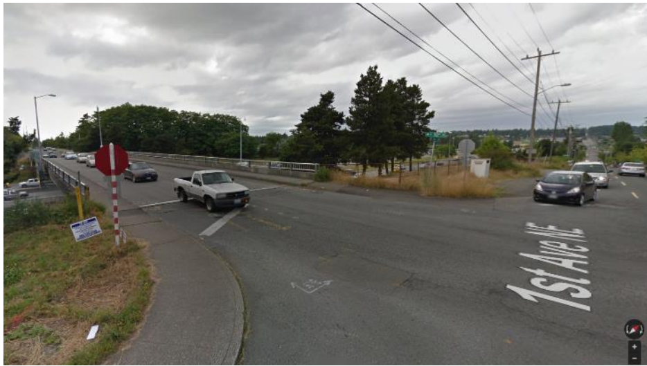
92 nd Street Overpass
