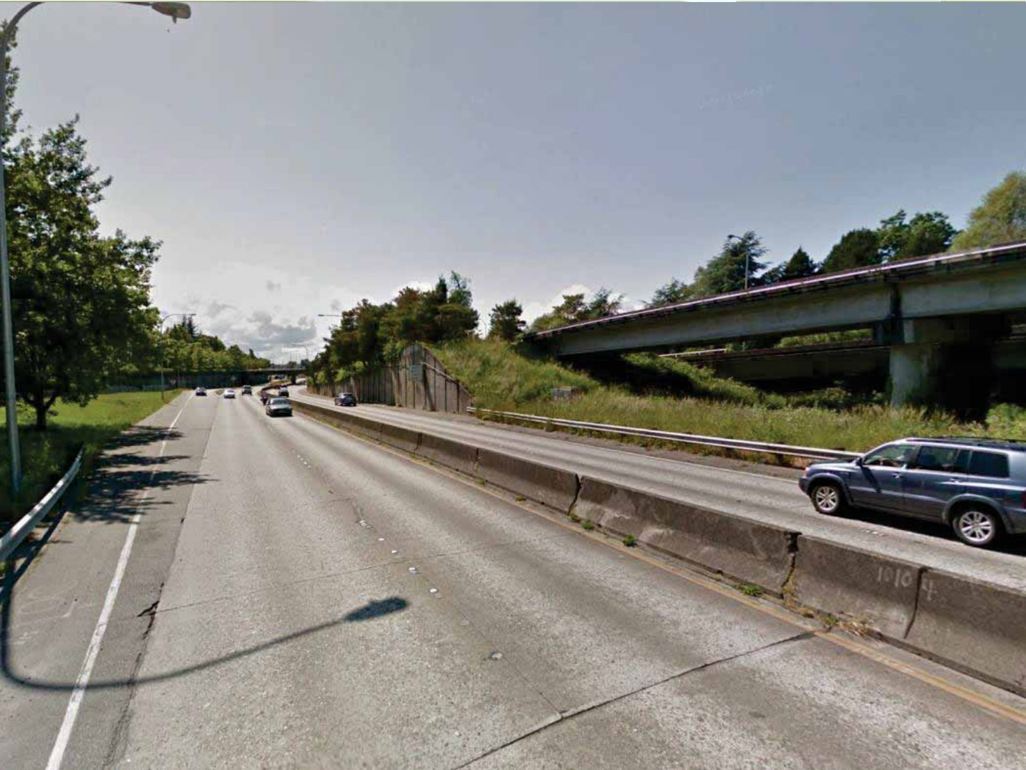
17. View of East Portal from Mainline (looking west)
