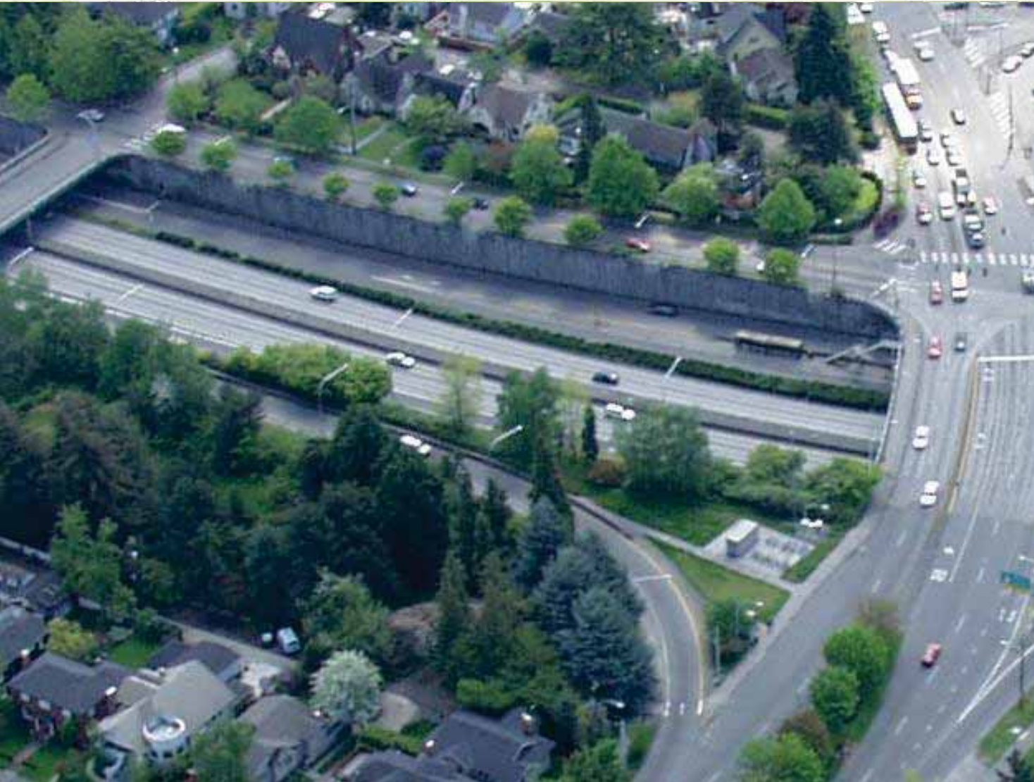
6. View of West Lid at Transit Plaza (looking southeast)
