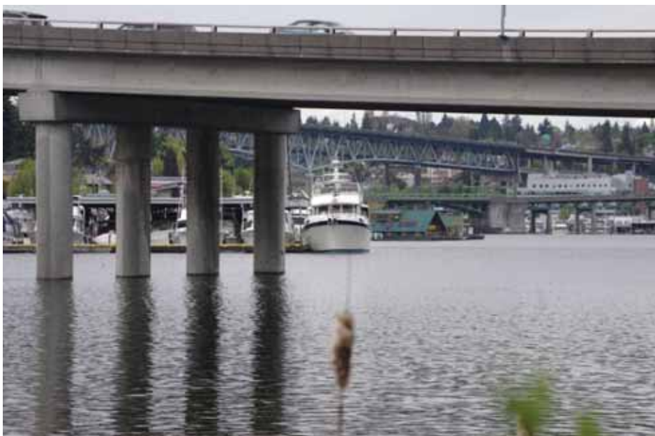
Portage Bay Bridge looking northwest from Montlake Playfield (I-5 Ship Canal and University Bridge in background)
