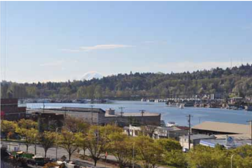
Portage Bay Bridge looking southeast from University Bridge
