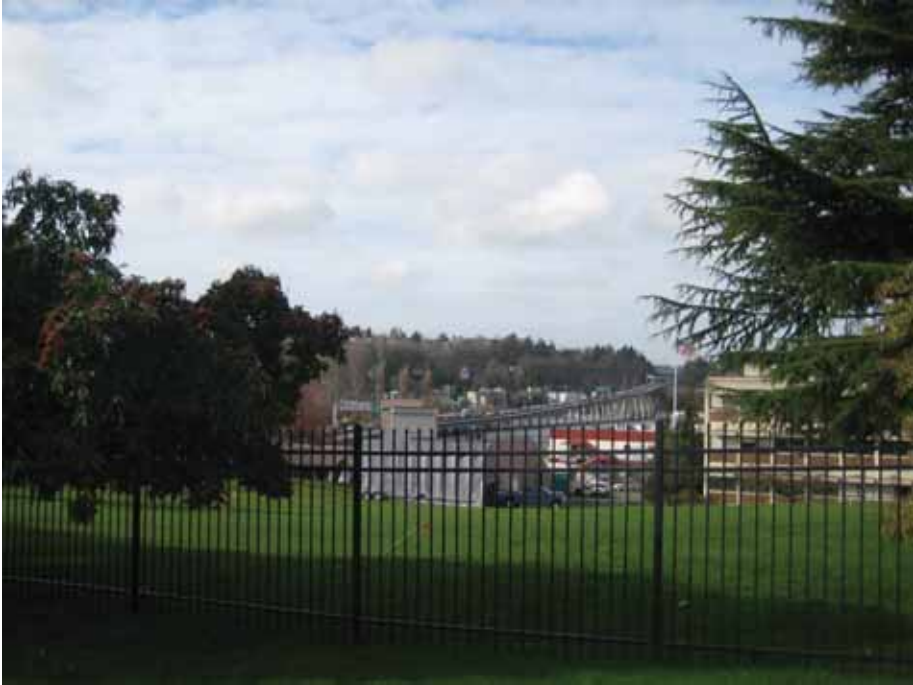
Portage Bay Bridge looking west from West Montlake Park
