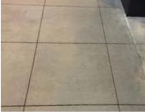
2x2 standard scoring on concrete sidewalks
