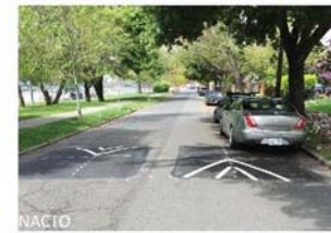
Speed humps installed on hills may include a cut for downhill bicyclists.
