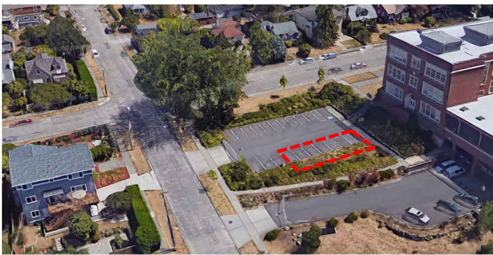
AERIAL VIEW FROM SW HINDS STREET LOOKING SE
