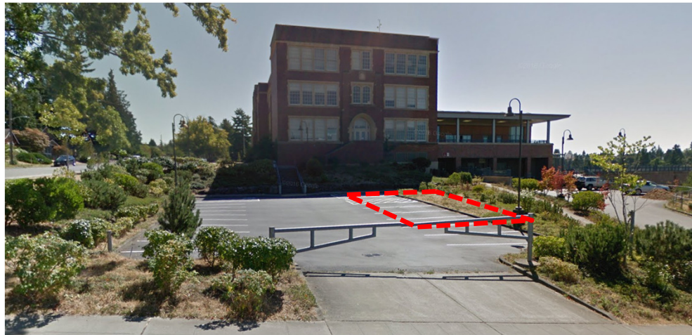
VIEW FROM SW HINDS STREET LOOKING S
