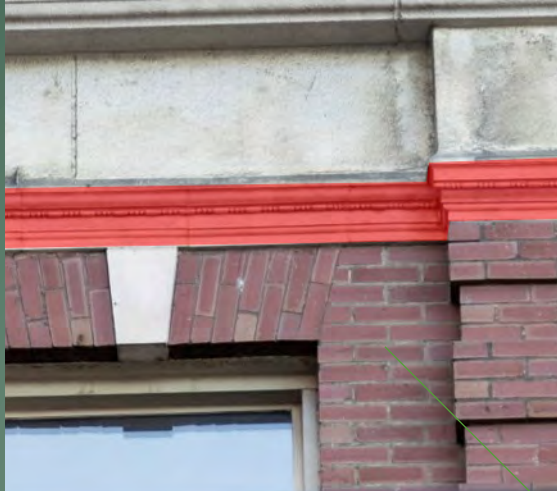
Jack arch, terra cotta key stone and band at cornice (shaded red)
