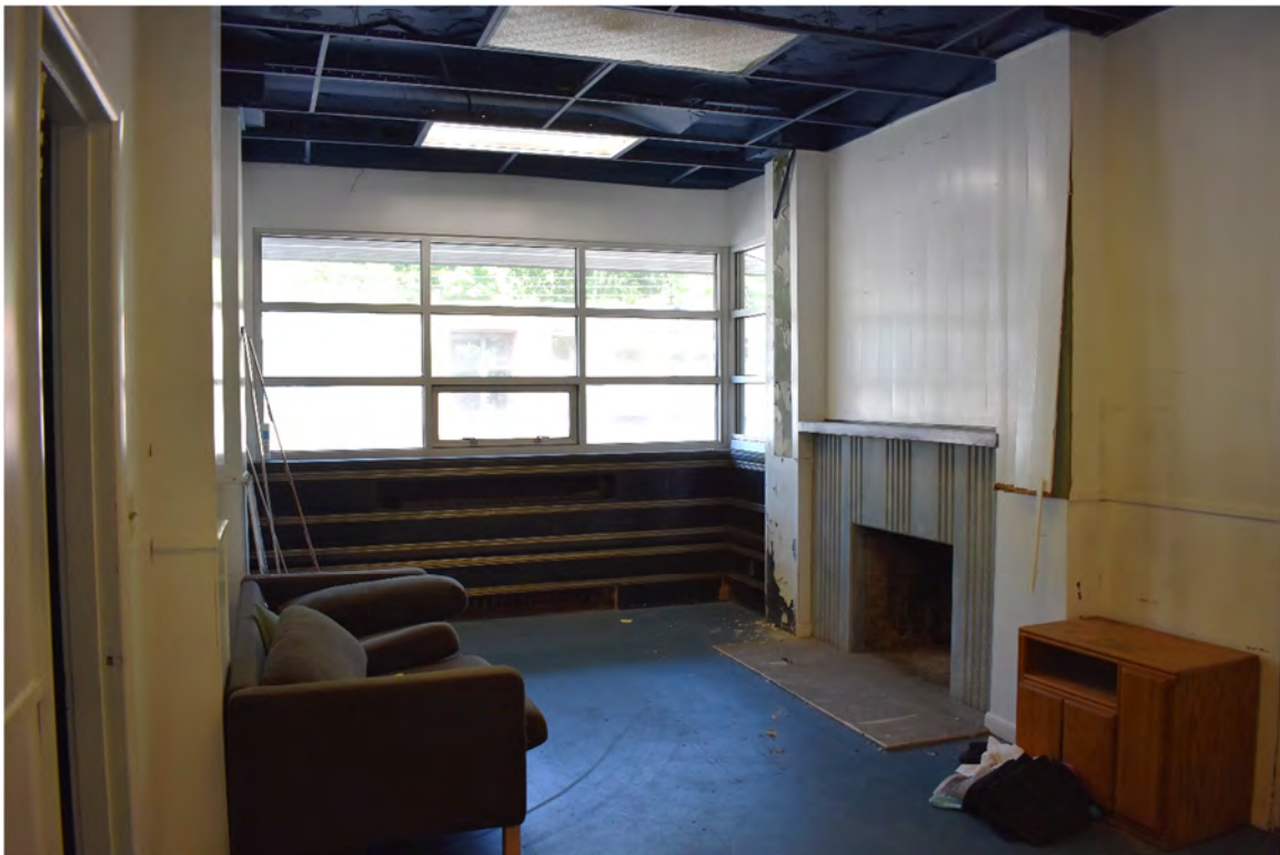
Fig. 37 – Interior, upper floor, office space along east wall. Originally built as the executive office. (May 2019)
