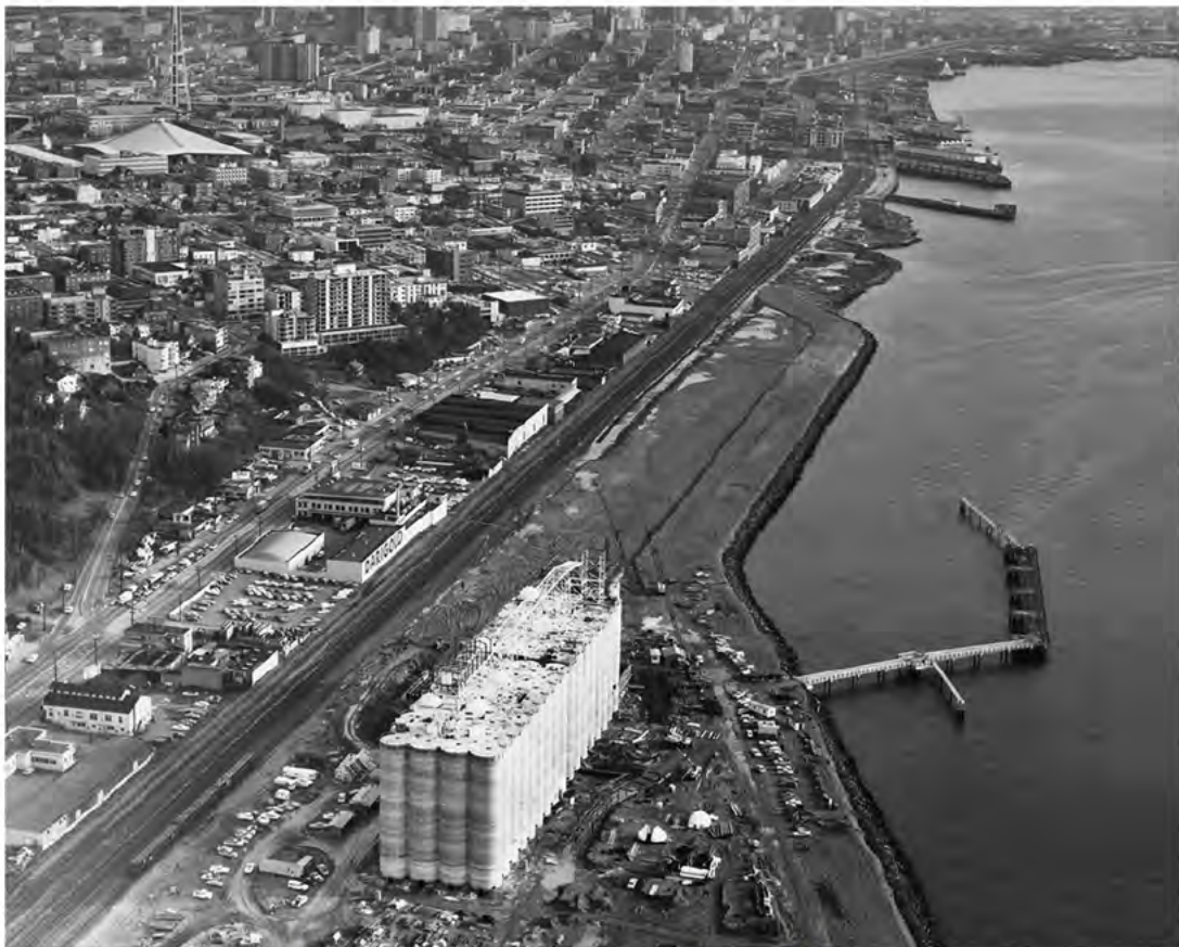
Fig. 78 – 1969 of Pier 86 grain elevator and terminal under construction. (SMA 63981)
