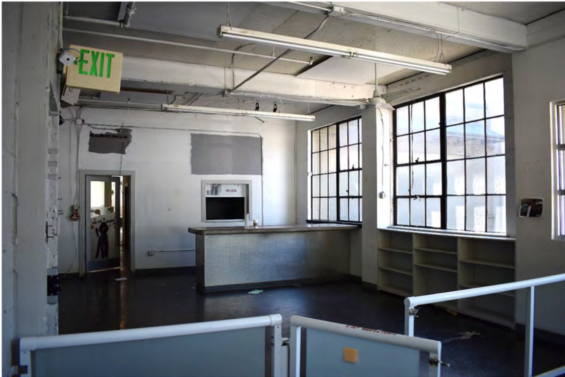
Fig. 31 – Interior, upper floor, reception desk area at northeast building corner. (May 2019) Windows face north and overlook the loading dock.
