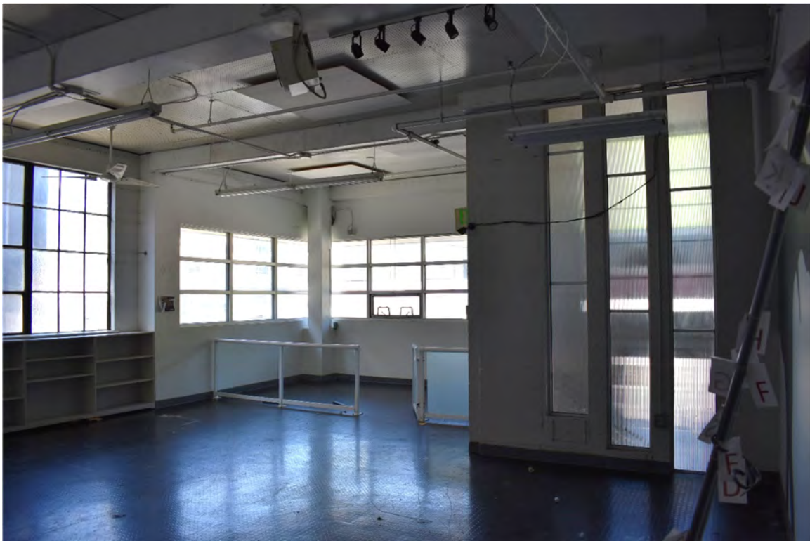
Fig. 29 – Interior, upper floor, reception desk area at northeast building corner. Note reights to tower entry vestibule at right. (May 2019)
