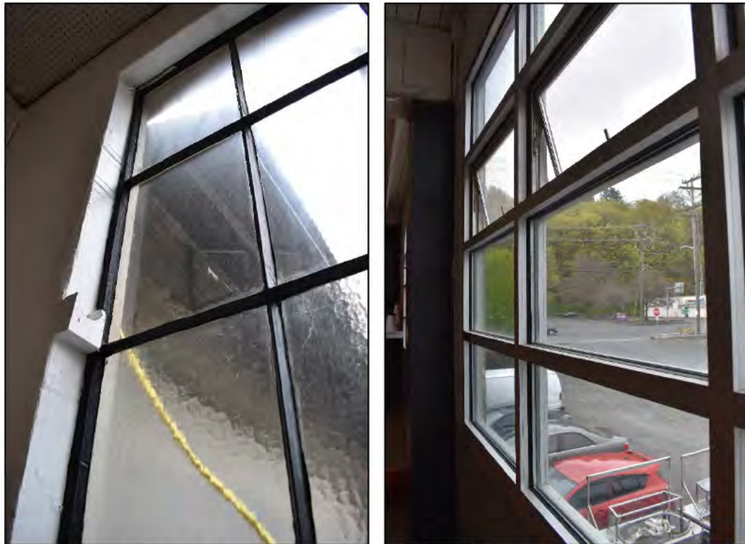
Fig. 33 – Interior, upper floor, detail of typical original (left) and non-original (right) windows.
