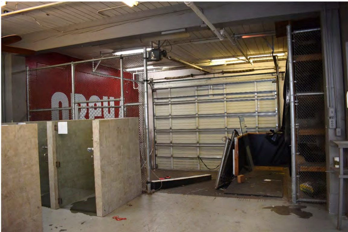
Fig. 41 – Interior, upper floor, at loading dock (note garage door). (May 2019) The garage door opens onto Elliott Avenue on the east building elevation.
