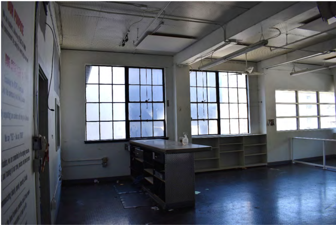
Fig. 30 – Interior, upper floor, reception desk area at northeast building corner. Note original windows at left and center, overlooking loading dock. (May 2019)
