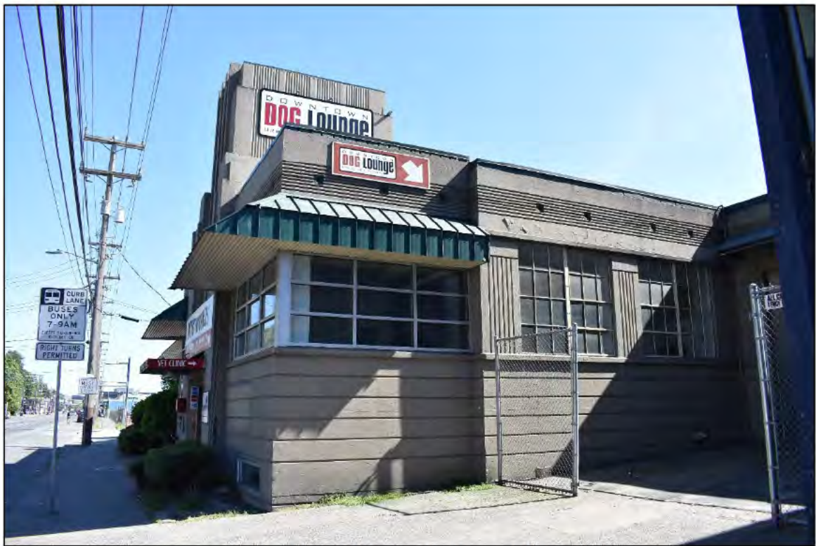
Fig. 14 – East and north elevations. (May 2019)
