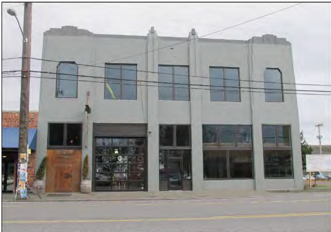
Fig. 129 – Marwood Electric Company (1930) at 1712 1 st Avenue South.
