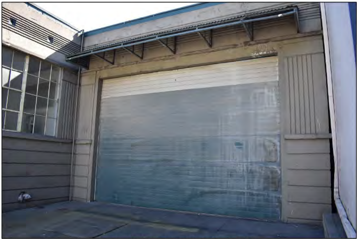
Fig. 16 – East elevation, detail of loading dock. Note original window on north elevation visible at left.
