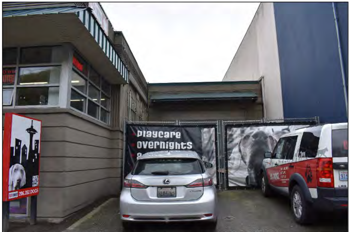
Fig. 15 – East and north elevations, detail of loading dock.
