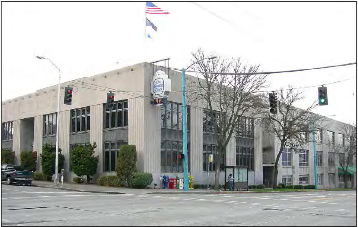
Fig. 132 – Seattle Times Office and Printing Plant (Robert Reamer, 1931, altered). The building is a Seattle landmark. (Joe Mabel)
