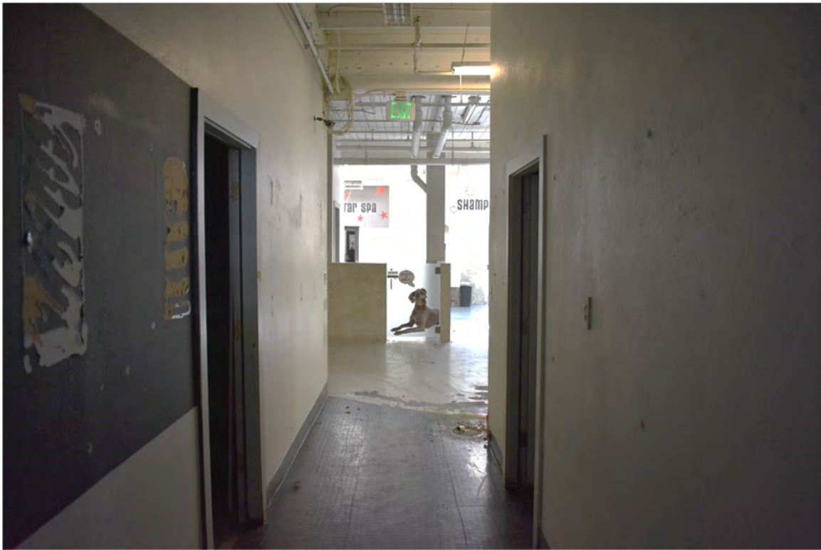
Fig. 40 – Interior, upper floor, interior corridor. (May 2019)
