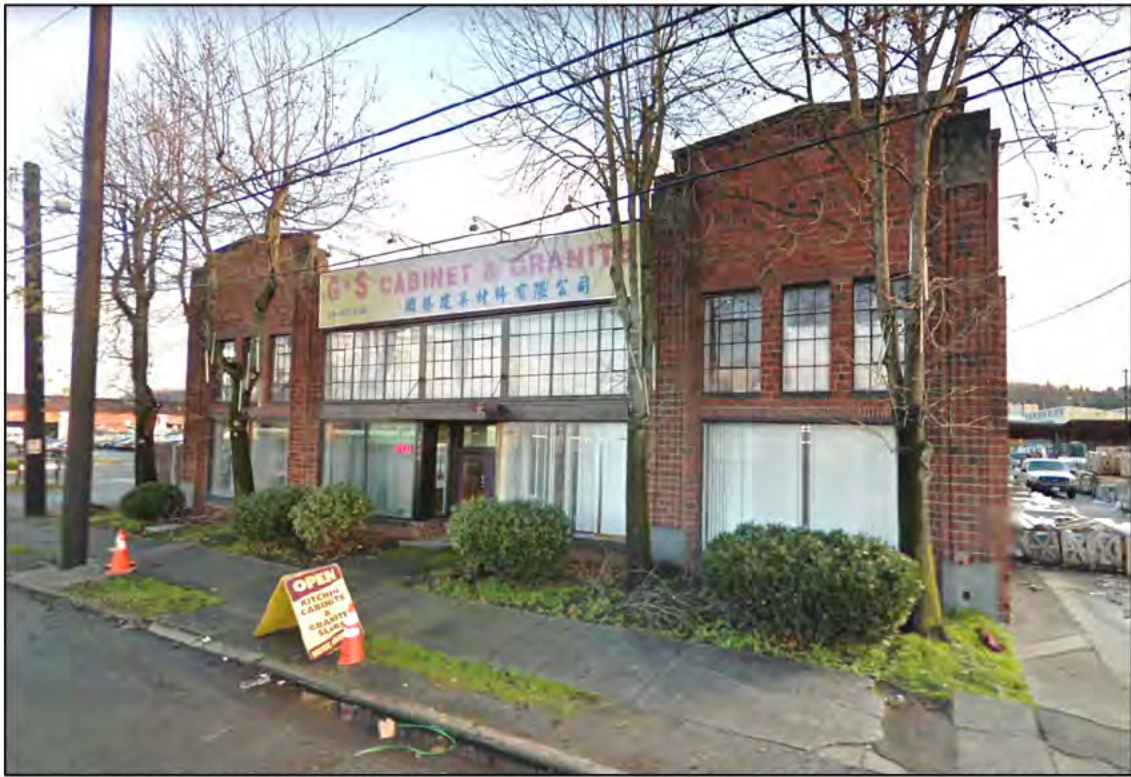
Fig. 134 – Pacific Hoist & Warehouse Company (1931) at 3200 4 th Avenue South. (Google Maps Streetview)
