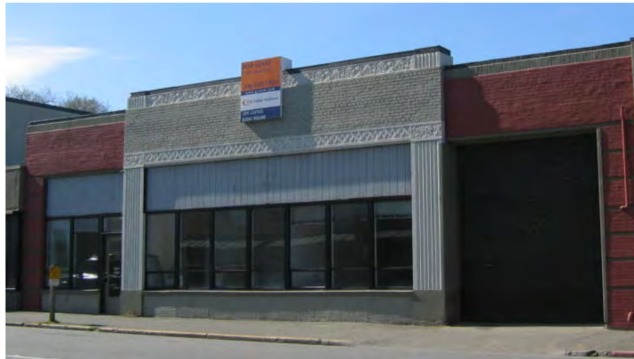
Fig. 112 – 227 9 th Avenue North aka Builder's Hardware (1931, G. W. Stoddard) (King County Assessor)
