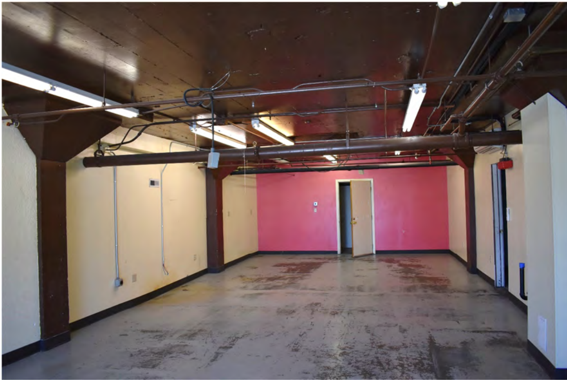
Fig. 50 – Interior, lower floor, commercial tenant spaces. (May 2019) Note concrete pier structure with drop panels and pyramidal caps.
