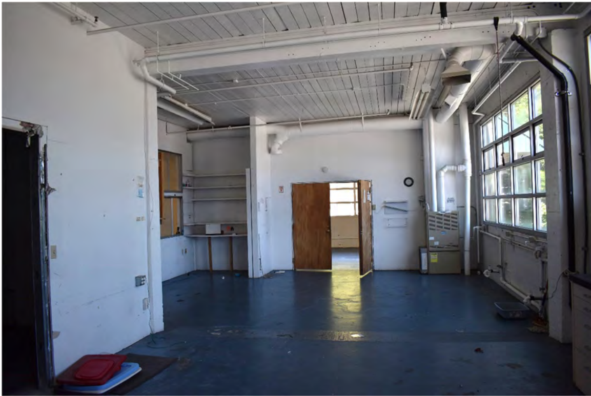
Fig. 36 – Interior, upper floor, former office space along south wall. (May 2019)
