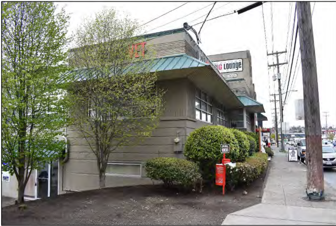
Fig. 9 – East elevation, south corner.
