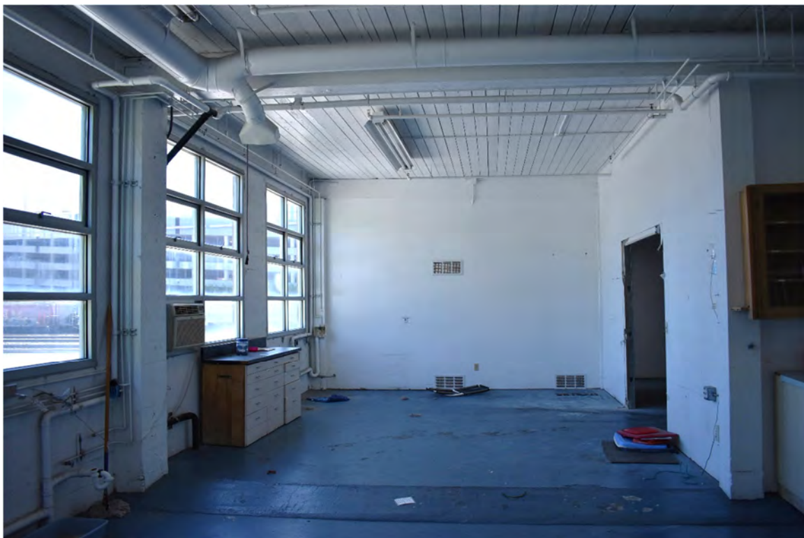
Fig. 35 – Interior, upper floor, former office space along south wall. (May 2019)
