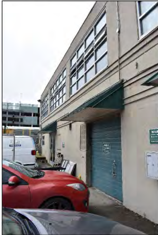
Fig. 21 – South elevation, detail.
