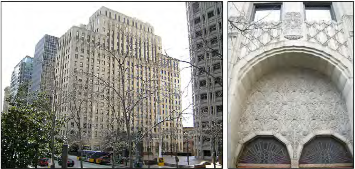
Fig. 119 – Exchange Building (John Graham Sr., 1929-31), a Seattle landmark. (Joe Mabel)
