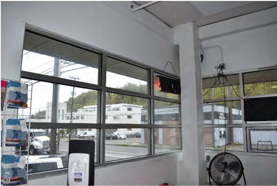
Fig. 32 – Interior, upper floor, reception desk area at northeast building corner.
