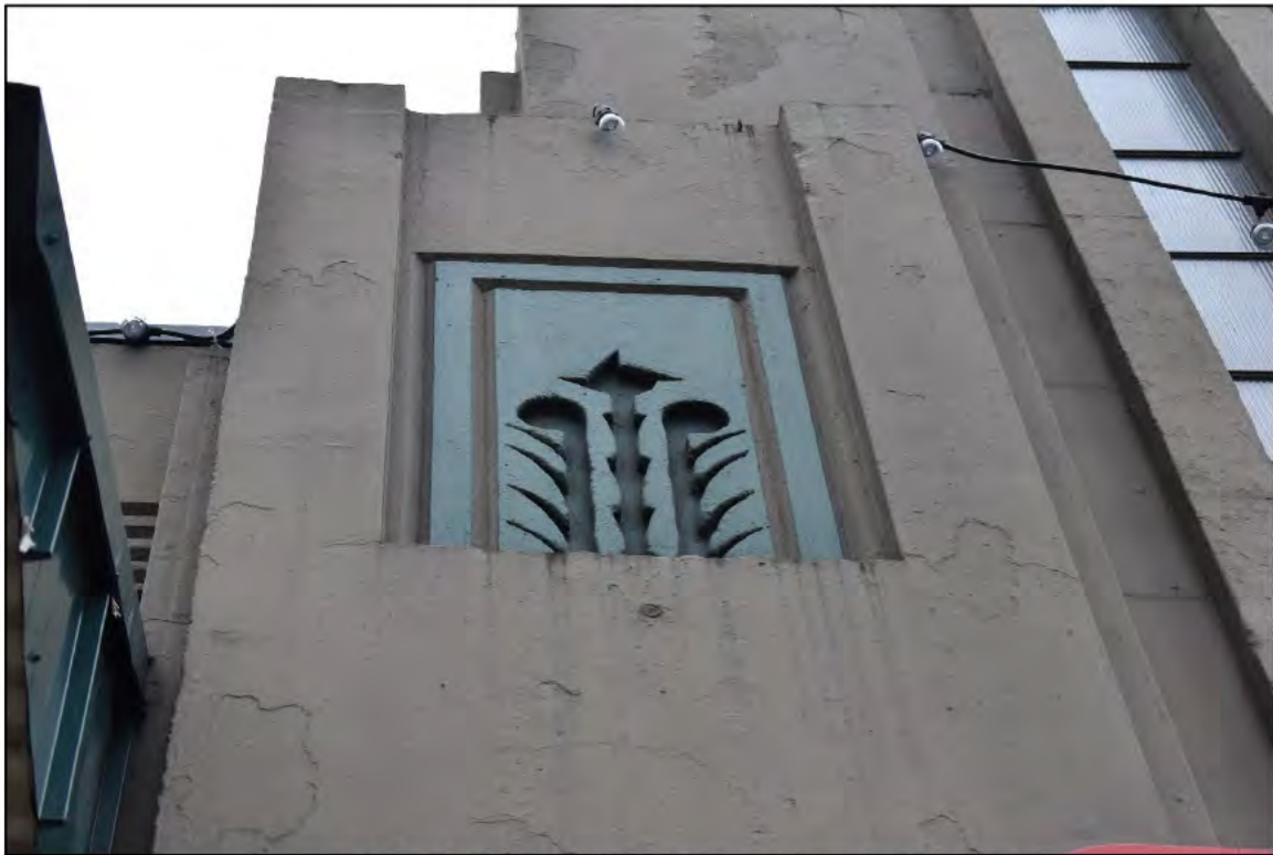
Fig. 12 – East elevation, detail of entry tower, concrete work.
