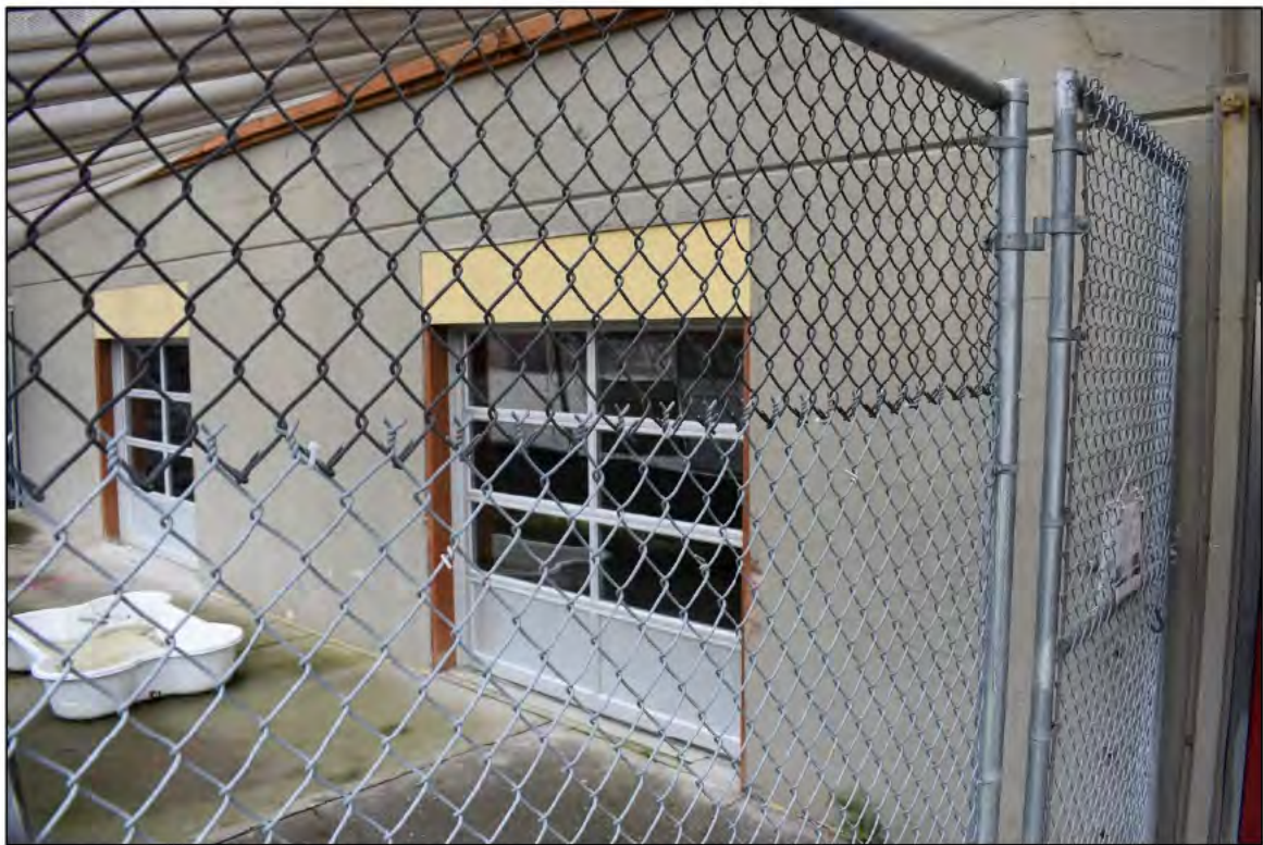
Fig. 24 – West elevation, detail of lower level openings, north part.
