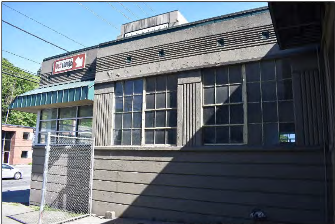
Fig. 17 – North elevation (at loading dock). (May 2019)
