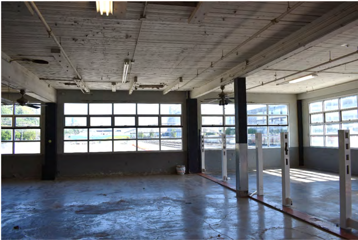
Fig. 44 – Interior, upper floor at southeast building corner, view east (former factory floor). (May 2019)
