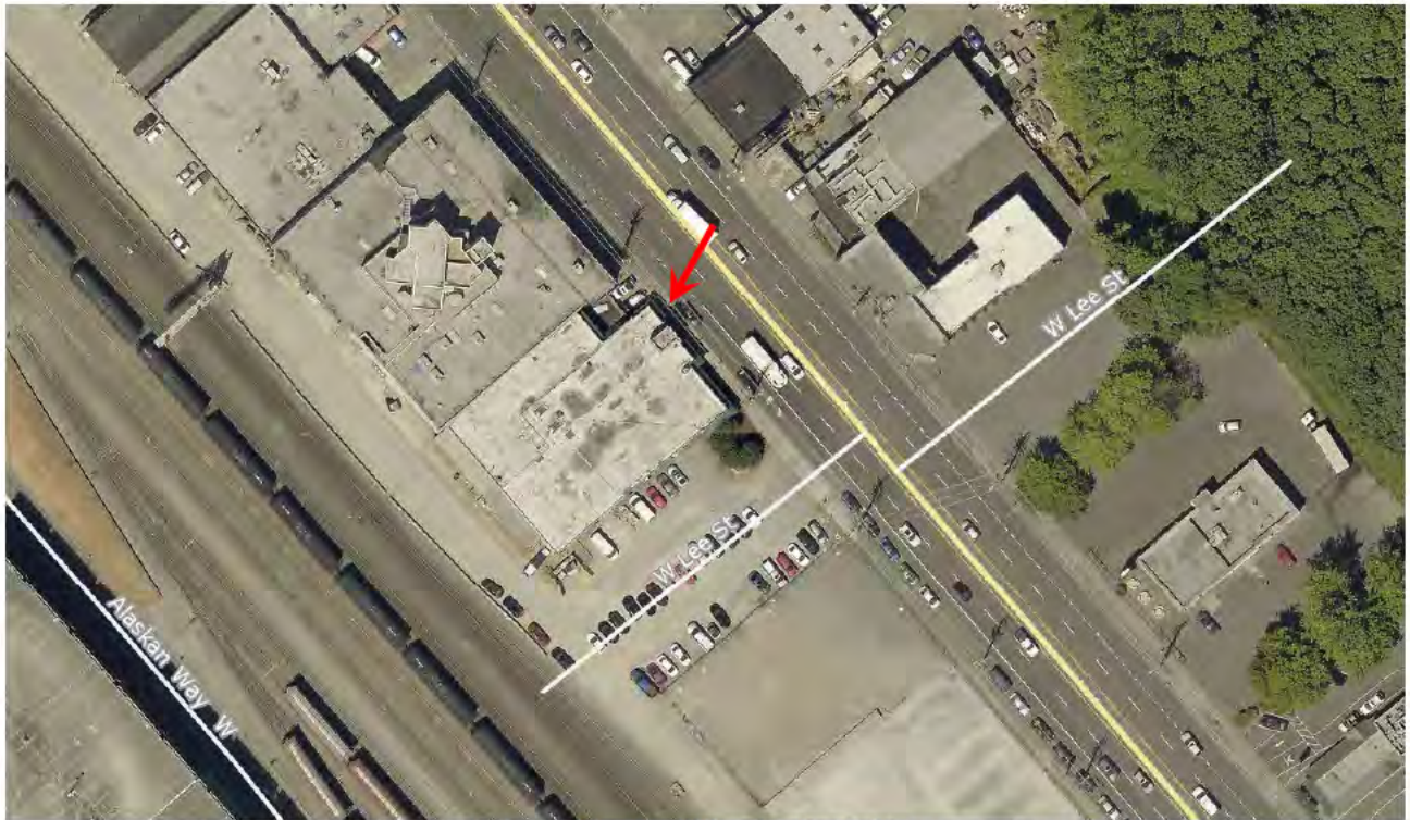
Fig. 3 – Aerial photo of site. Subject building indicated by arrow. True north is up; for purposes of the report, Elliott Avenue will be considered oriented north-south, so that the building front elevation facing Elliott Avenue is the east elevation. (Google Maps)
