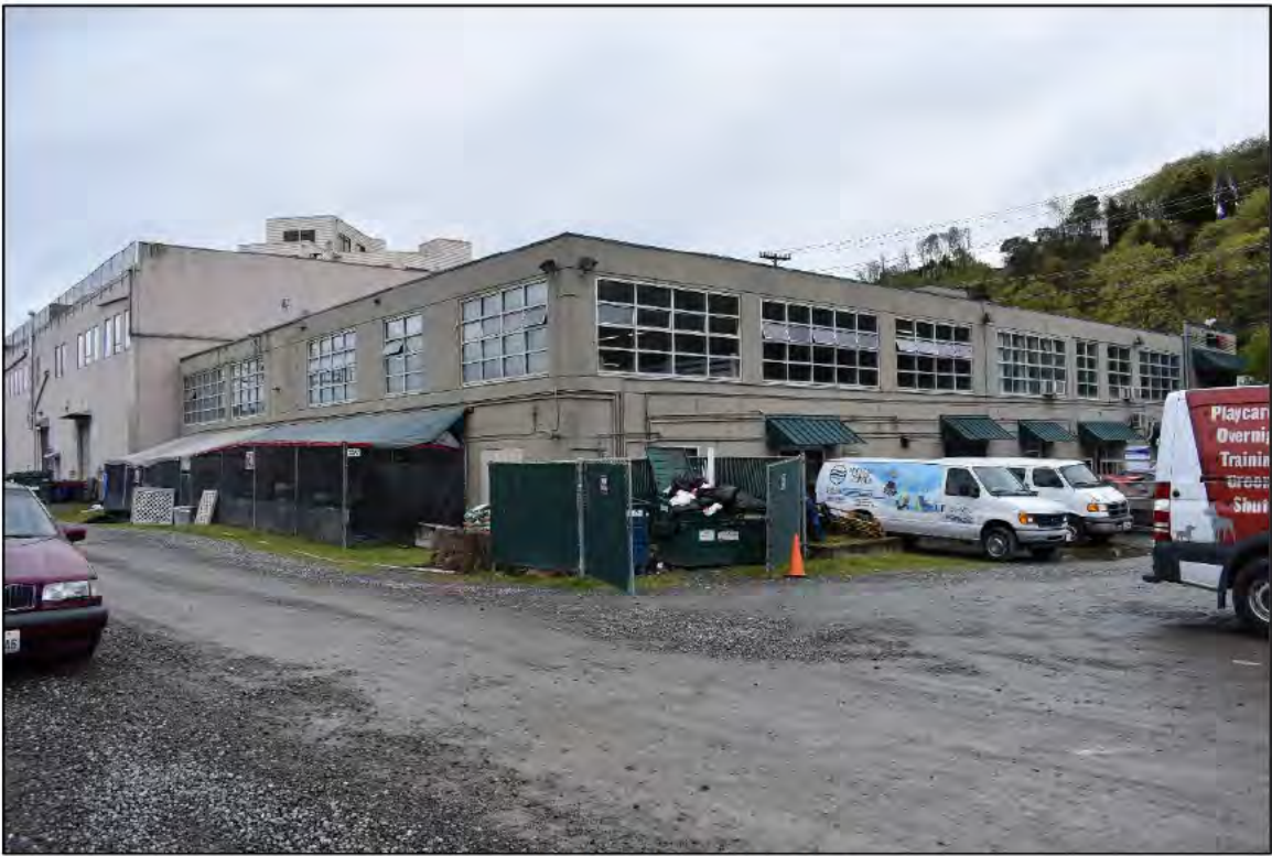
Fig. 22 – South and west elevations.
