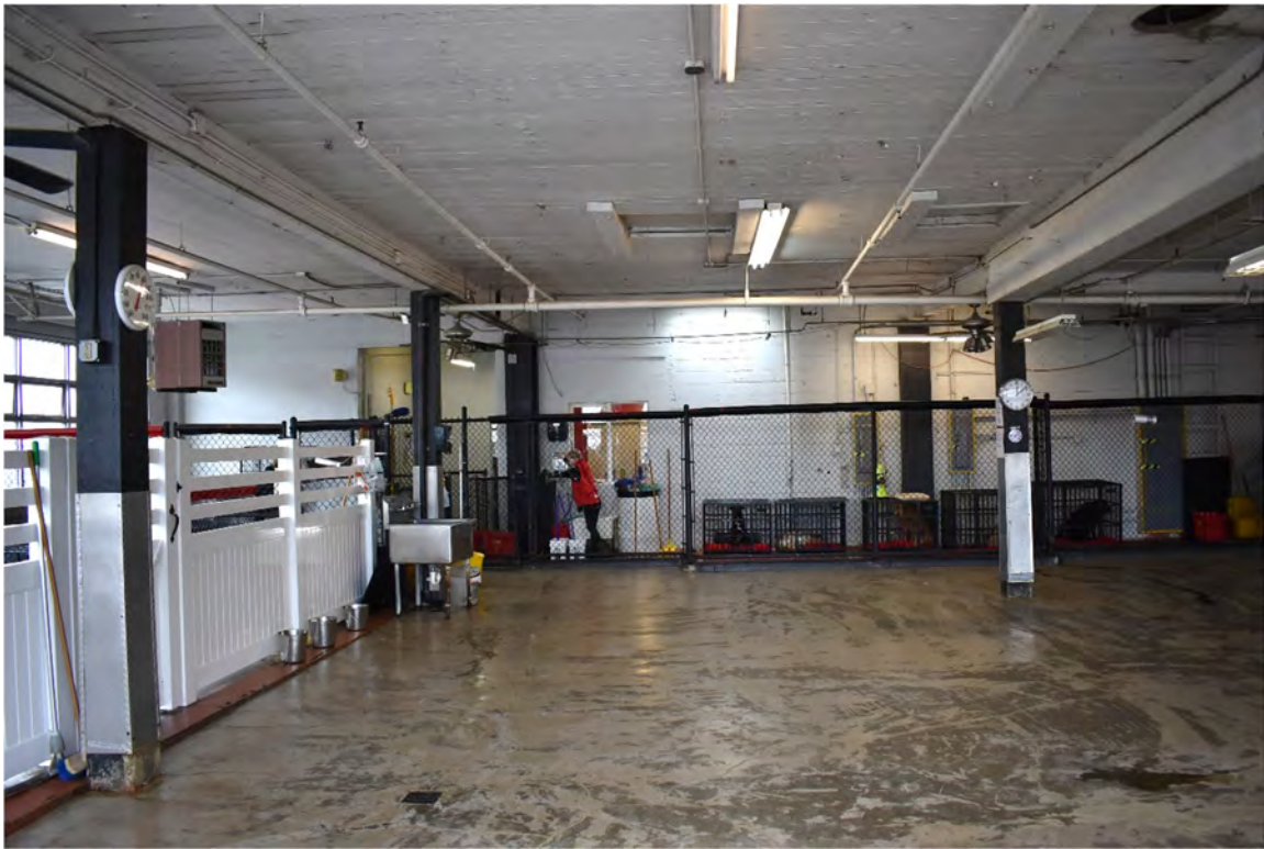
Fig. 42 – Interior, upper floor at southeast building corridor, view north (former factory floor).
