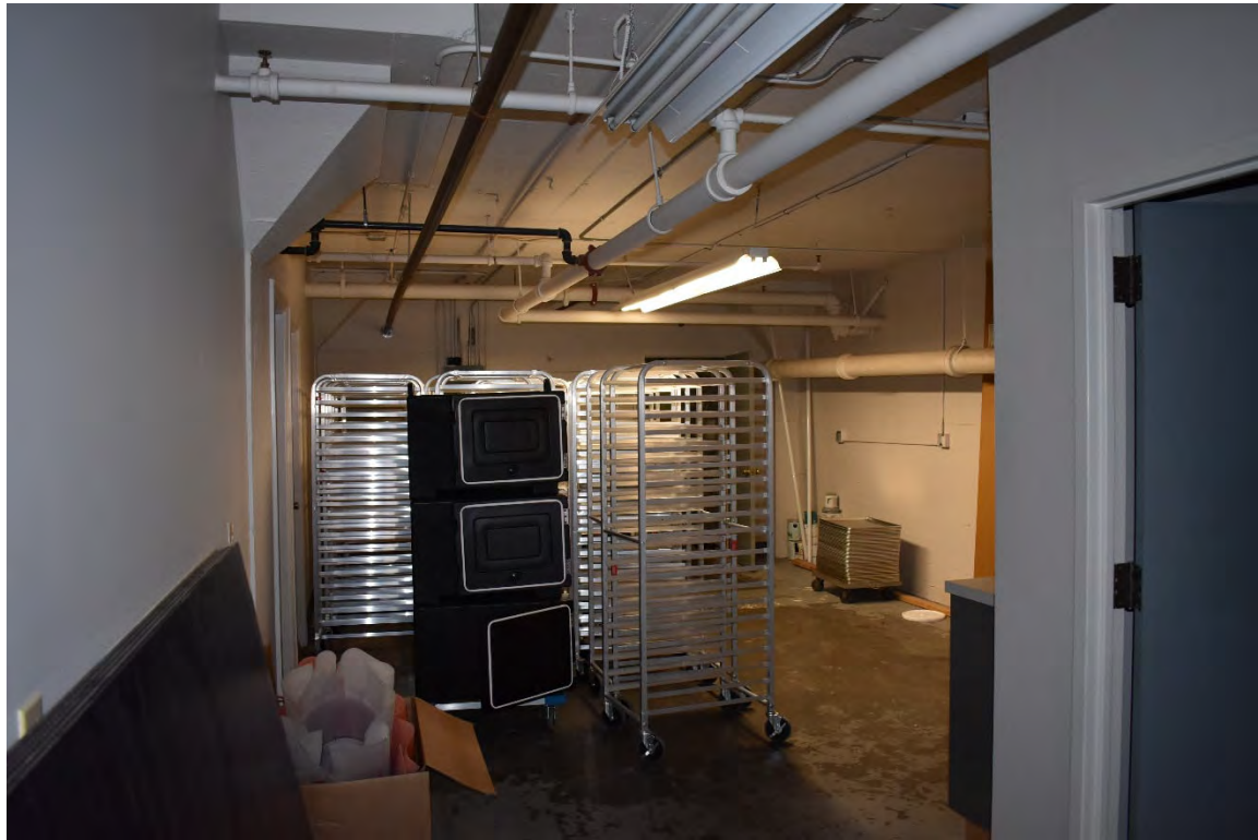
Fig. 51 – Interior, lower floor, typical interior corridor.
