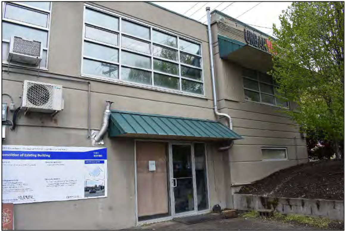
Fig. 20 – South elevation, detail.
