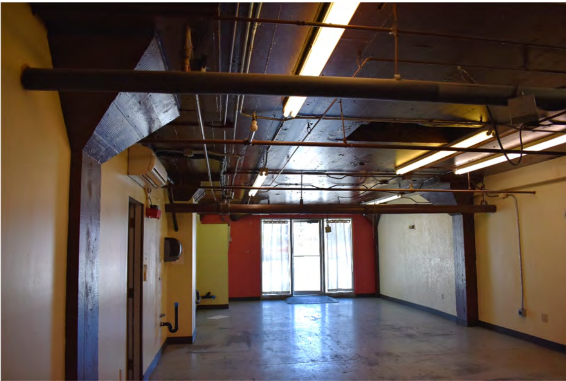
Fig. 49 – Interior, lower floor, commercial tenant spaces. Door to outside is on south elevation. Note concrete pier structure with drop panels and pyramidal caps. (May 2019)
