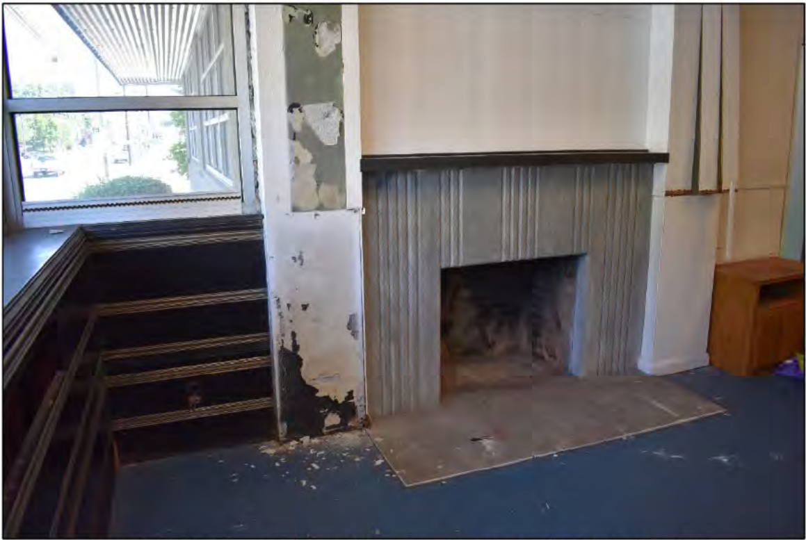
Fig. 38 – Interior, upper floor, office space along east wall, detail of fireplace. Originally built as the executive office. (May 2019)
