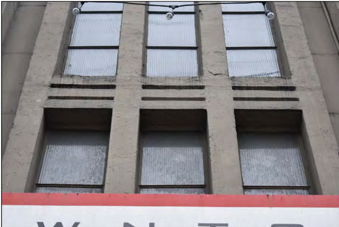
Fig. 13 – East elevation, detail of entry tower, concrete work, windows.
