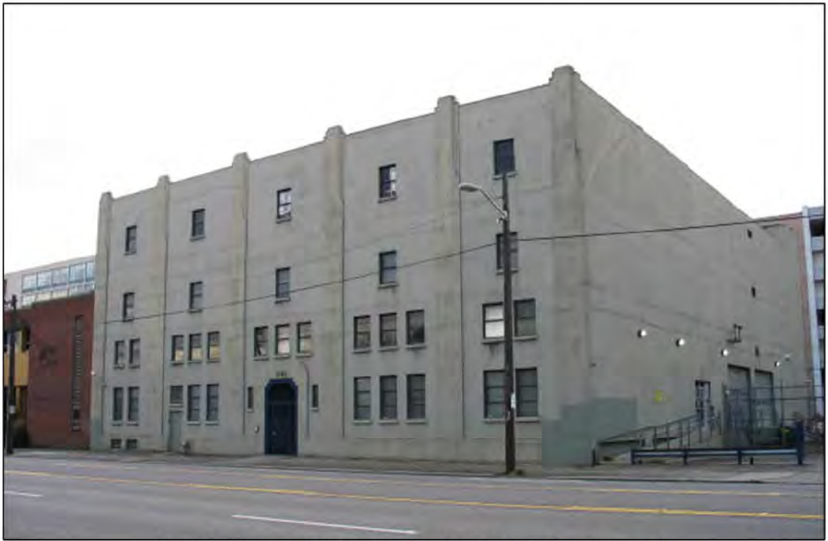
Fig. 130 – Eyres Storage Company (1930) at 2245 1 st Avenue S. (DON)
