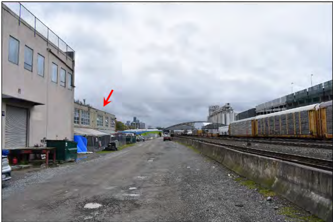
Fig. 6 – View south on railroad corridor at rear (Alaskan Way West right of way). Subject building indicated by arrow.
