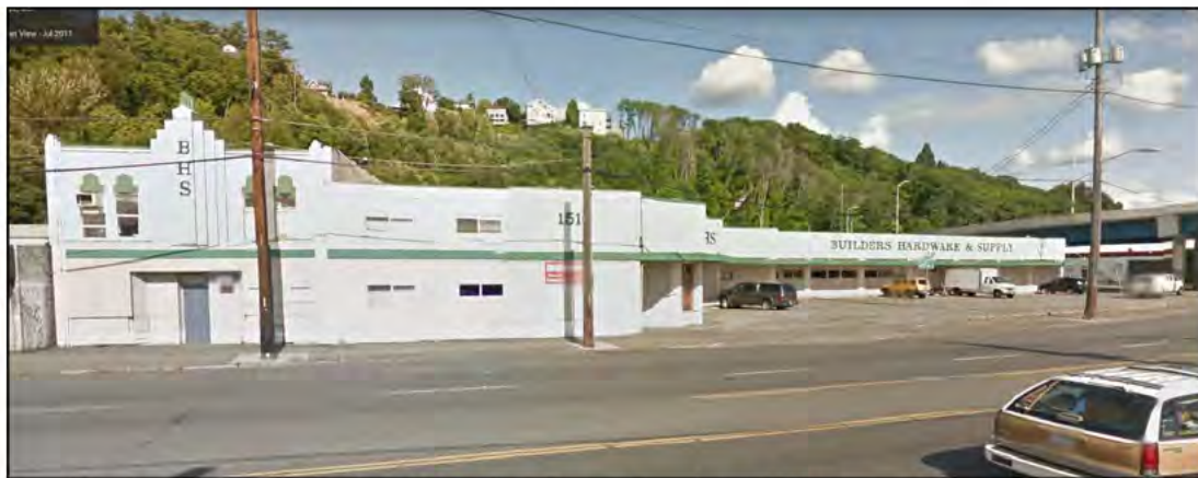
Fig. 82 – (Two images) Builder's Hardware Supply on Elliott Avenue at Galer Street, two blocks north of the subject site, was originally the Cove Mid-City Market, built in 1931 in the Art Deco style. An Art Deco remnant remains at the north end (lower image, far left). (PSRA, from Rob Ketcherside; and Google Maps Streetview).
