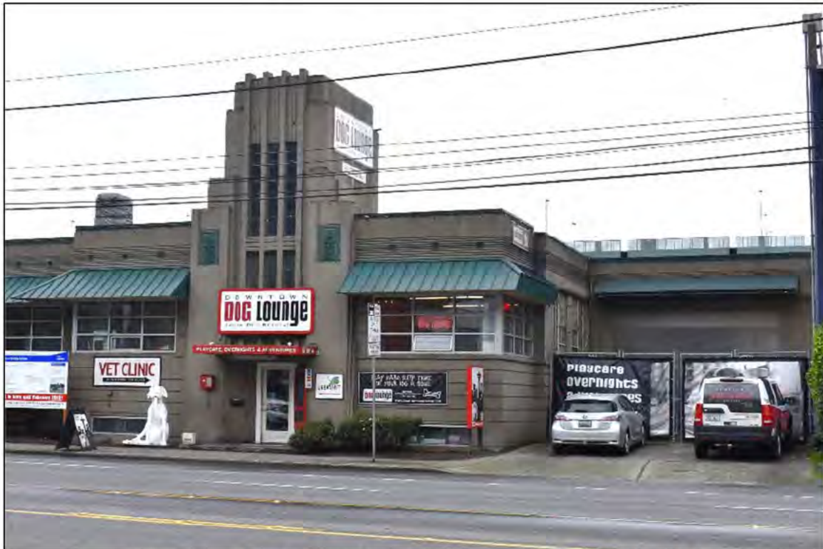
Fig. 10 – East elevation, north portion at entry tower and loading dock.
