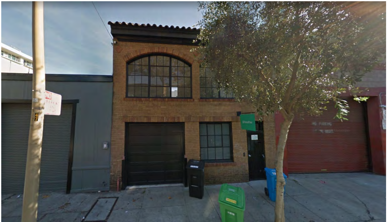
Fig. 103 – San Francisco: William's first San Francisco CA factory location, at 459 Clementina Street, used c.1928-1935. (Google Maps Streetview)
