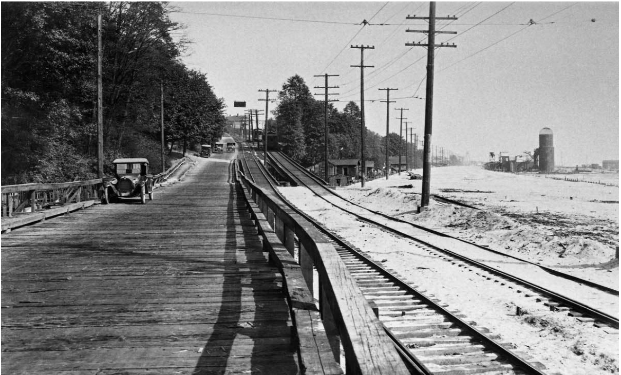
Fig. 67 – 1921 view south on Mercer Street (left) merging onto Elliott Avenue (right), which was initially built over tideflats but here being filled. Building in distance is a creosote works at West Thomas Street (now location of pedestrian bridge over Elliott to waterfront). (SMA 1862)
