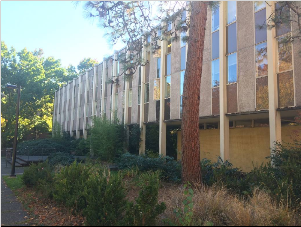
Figure 17. View looking east/southeast along the primary north facade.
