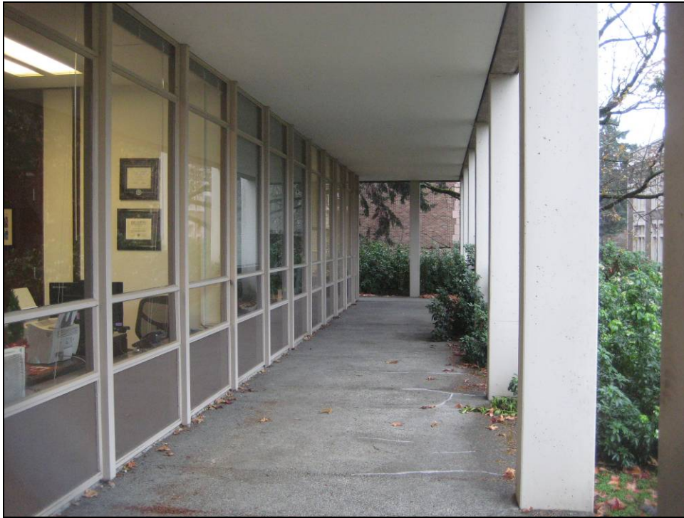
Figure 23. View looking east along the loggia at the south side of the building. This section of the perimeter walls features glazing and spandrel panels.
