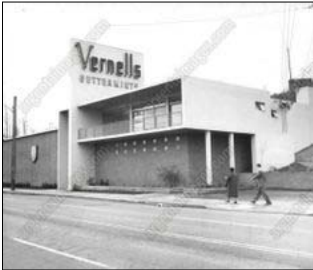
Figure 32. Left, Vernell's Fine Candies at 1825 Westlake Avenue N (1952). The building has been altered and is occupied by KCPQ television station.
