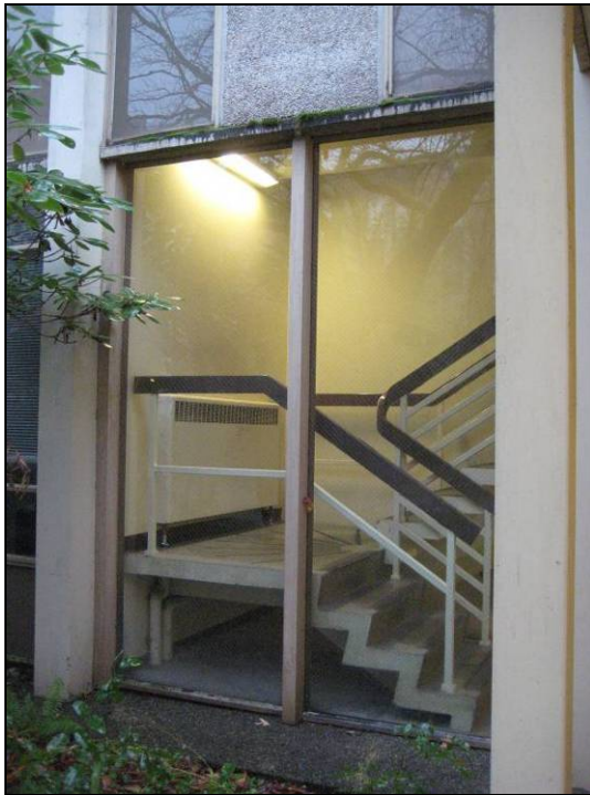
Figures 24 & 25. Two views within the entry courtyard show the transparency of the building and its frame due to glazing, including the exposed steel-framed stairs.
