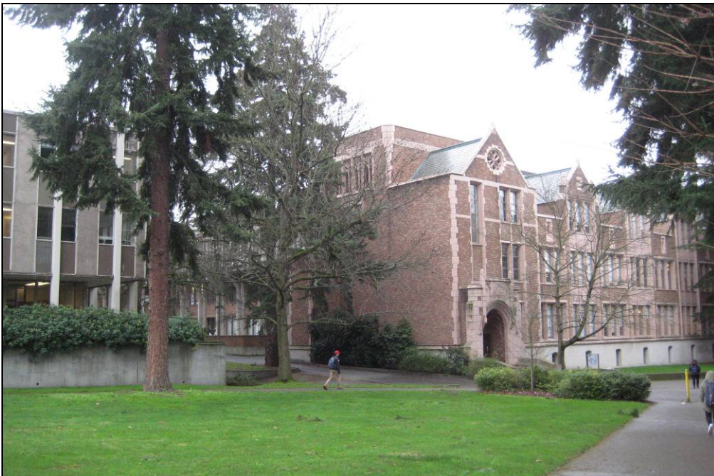
Figure 10. View looking northeast showing the relationship between Mackenzie Hall and the 1949 portion of the Gothic Revival Art Building to the east.
