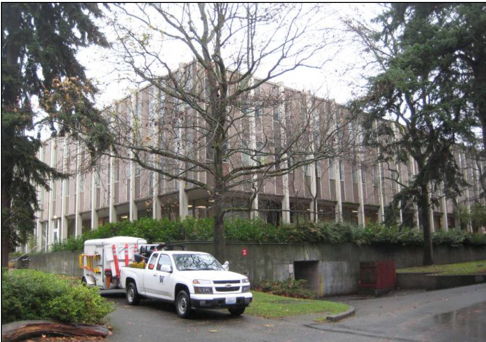
Figure 16. View looking northwest from Chelan Lane, showing the retaining wall and partial south and east facades.
