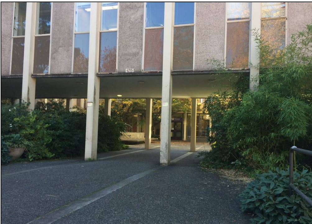
Figure 18. View looking southeast from in front of the building, into the courtyard.
