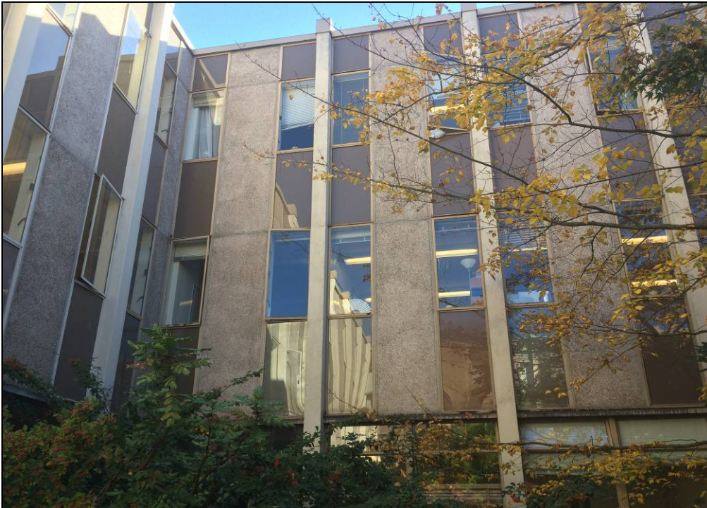
Figure 22. Detail view showing concrete columns, window bays, upper level spandrel and precast concrete panels.
