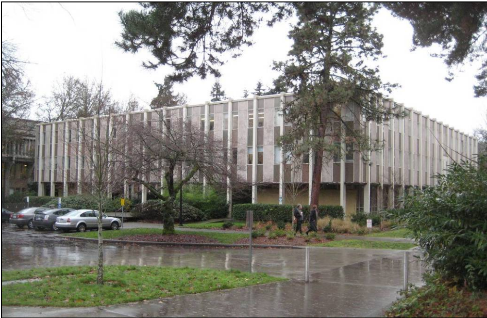
Figure 15. View looking southeast from Stevens Way, showing the primary north facade and an oblique view of the west facade.
