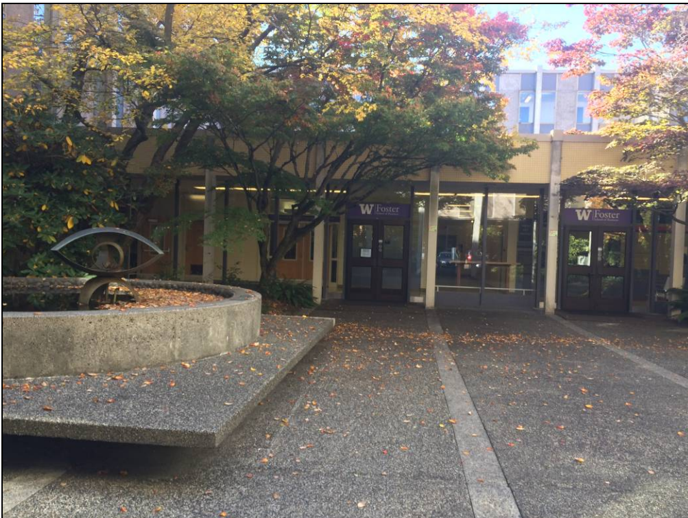
Figure 20. View looking south at the main entrance within the courtyard.
