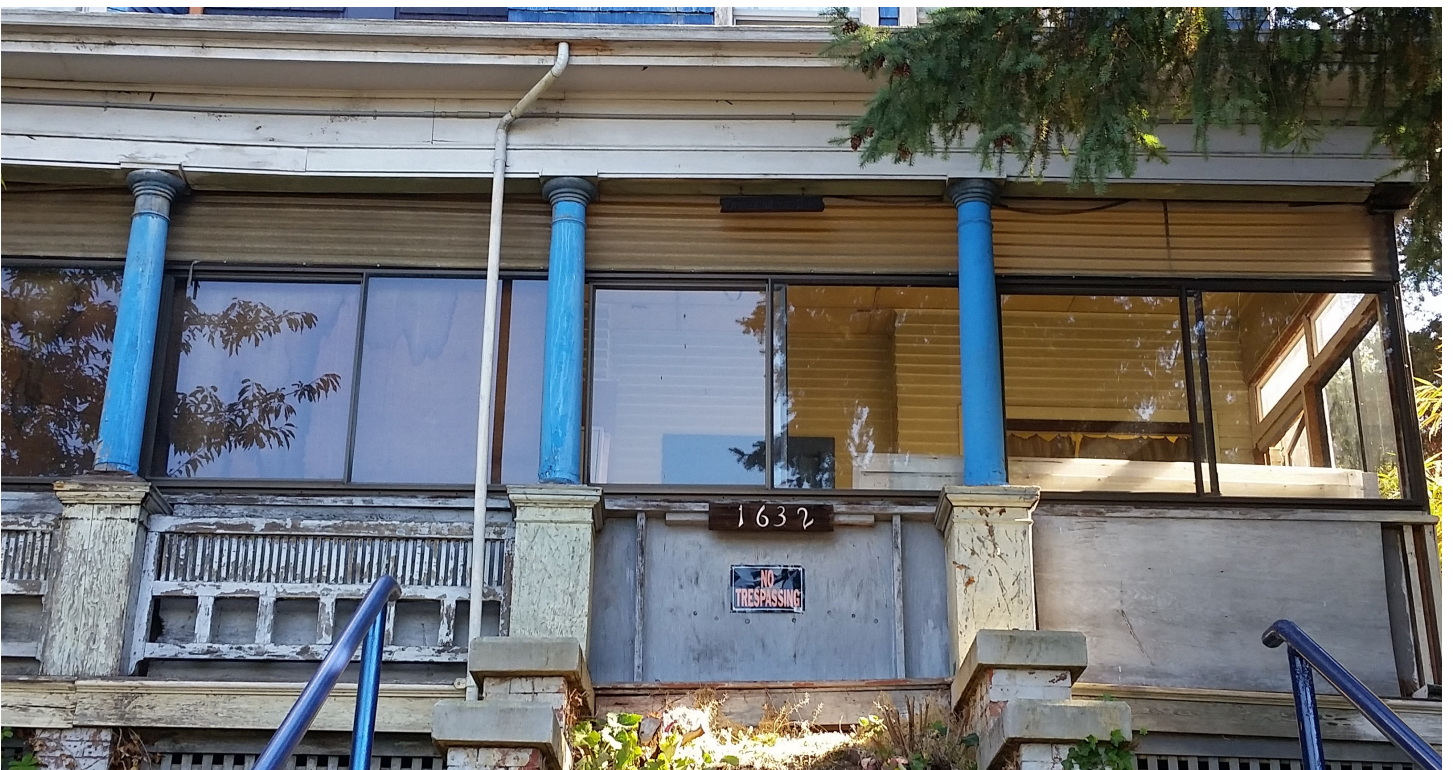
The Patrick J. Sullivan House; Close-up of porch enclosure alteration; Castanes Architects P.S. 2017
