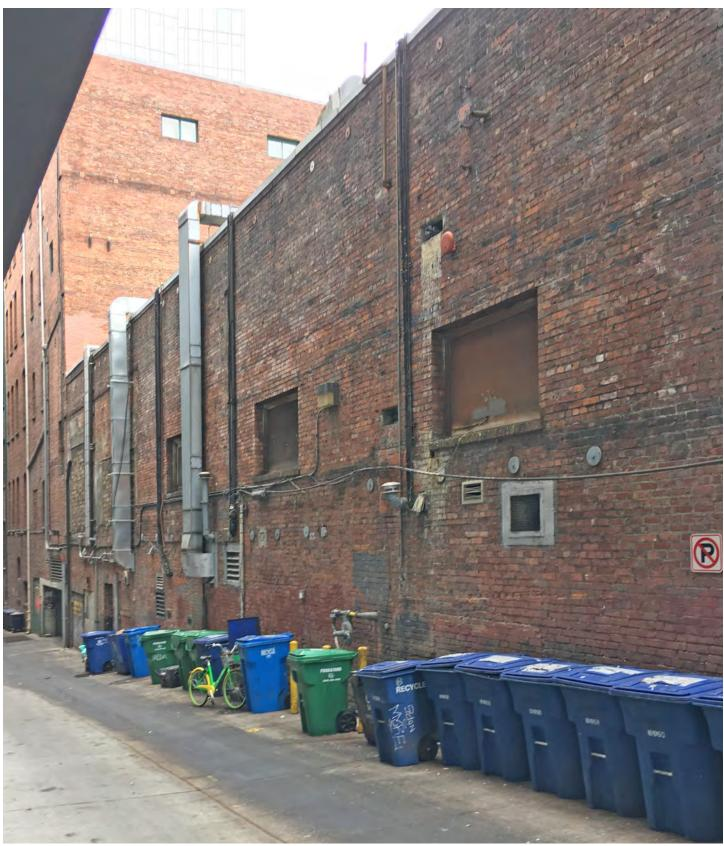
**Figure 19.** East alley facade looking south. The load bearing brick construction stems from the building's 1916 construction.
