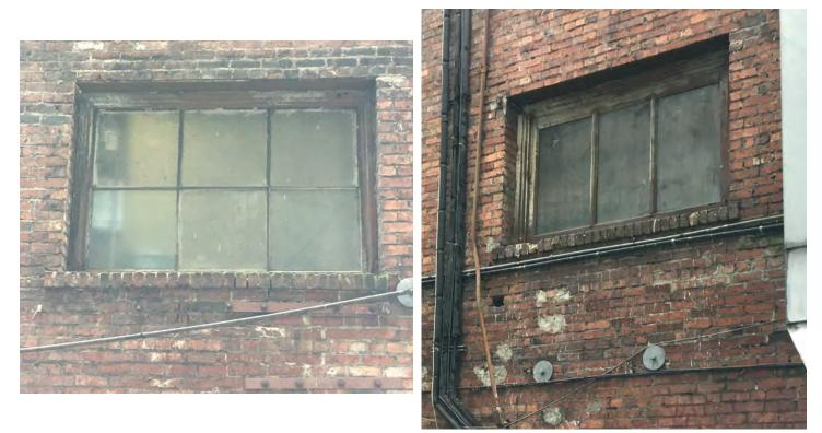
Figure 59. Alley facade, detail of the 6-lite (above left) and 3-lite (above right) sash along this facade.
