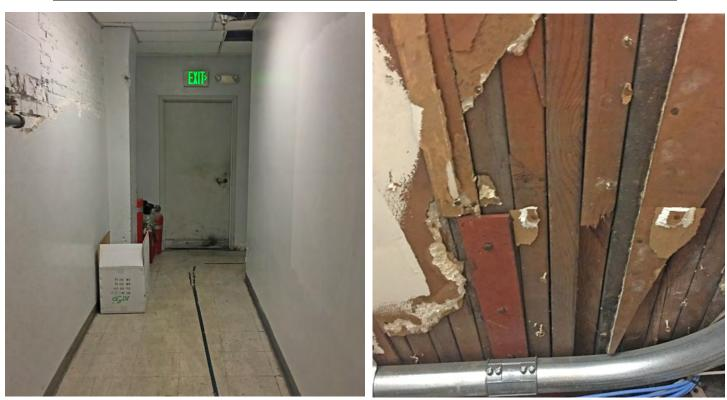
**Figure 58.** Service area, looking east and showing typical wall finishes (above left). The wall along the left side is the outer brick masonry wall. Note the brick pier that steps out to support the massive east to west beams carrying the second floor. A detail (above right) of the crib construction (2x boards on edge) comprising the floor structure for the second floor.
