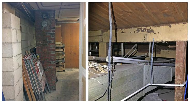
**Figure 57.** Service area, looking east along the rebuilt north facade. The brick chimney is original to the 1916 construction of the building (above left). A view looking west (above right) below the Showbox passageway showing the framing and ramp that are original to the 1939 remodel.
