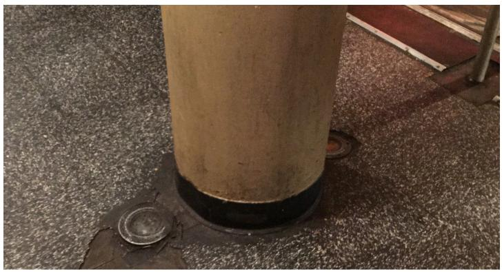
Figure 38. Showbox, detail of the floor lights original to the 1939 remodel that provided a light wash up the column.
