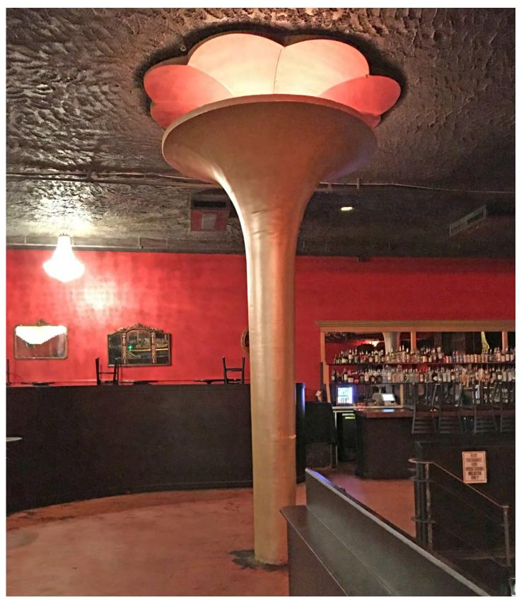
**Figure 37.** Showbox, detail of column original to the 1939 remodel. The core is a wood post with an outer plaster and wood form.
