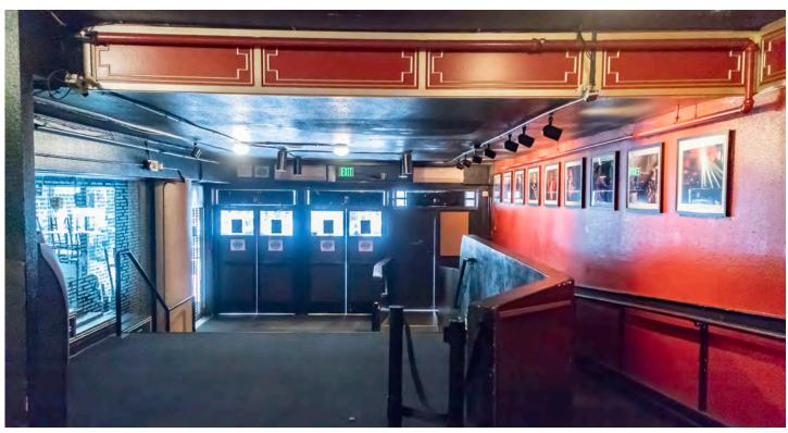
**Figure 25.** Showbox, looking west along the passageway at the three doorways providing access. The soffit above marks the line of the second floor framing. The volume of this passageway, door surrounds, and the large column at left are original to the 1939 remodel creating the Showbox.
