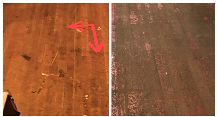
**Figure 43.** Showbox, detail (above left) of the maple dance floor original to the 1939 remodel. Detail (above right) of the Douglas fir flooring at sections of the raised seating area and behind the stage and at the ticket counter that are original to the 1939 remodel.
