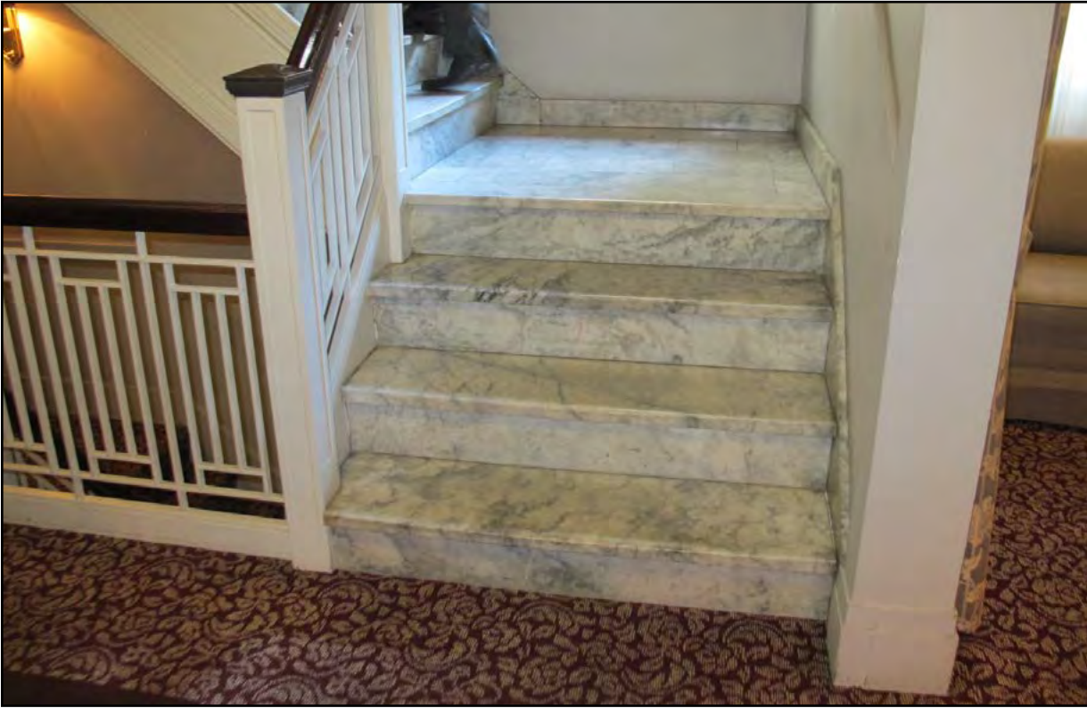
Figure 23 • Sheridan Apartment Building, main stair up from main floor
