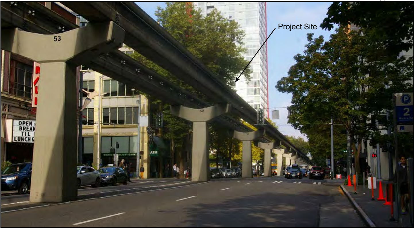
Figure 4 • View A - Viewing north on Fifth Avenue
