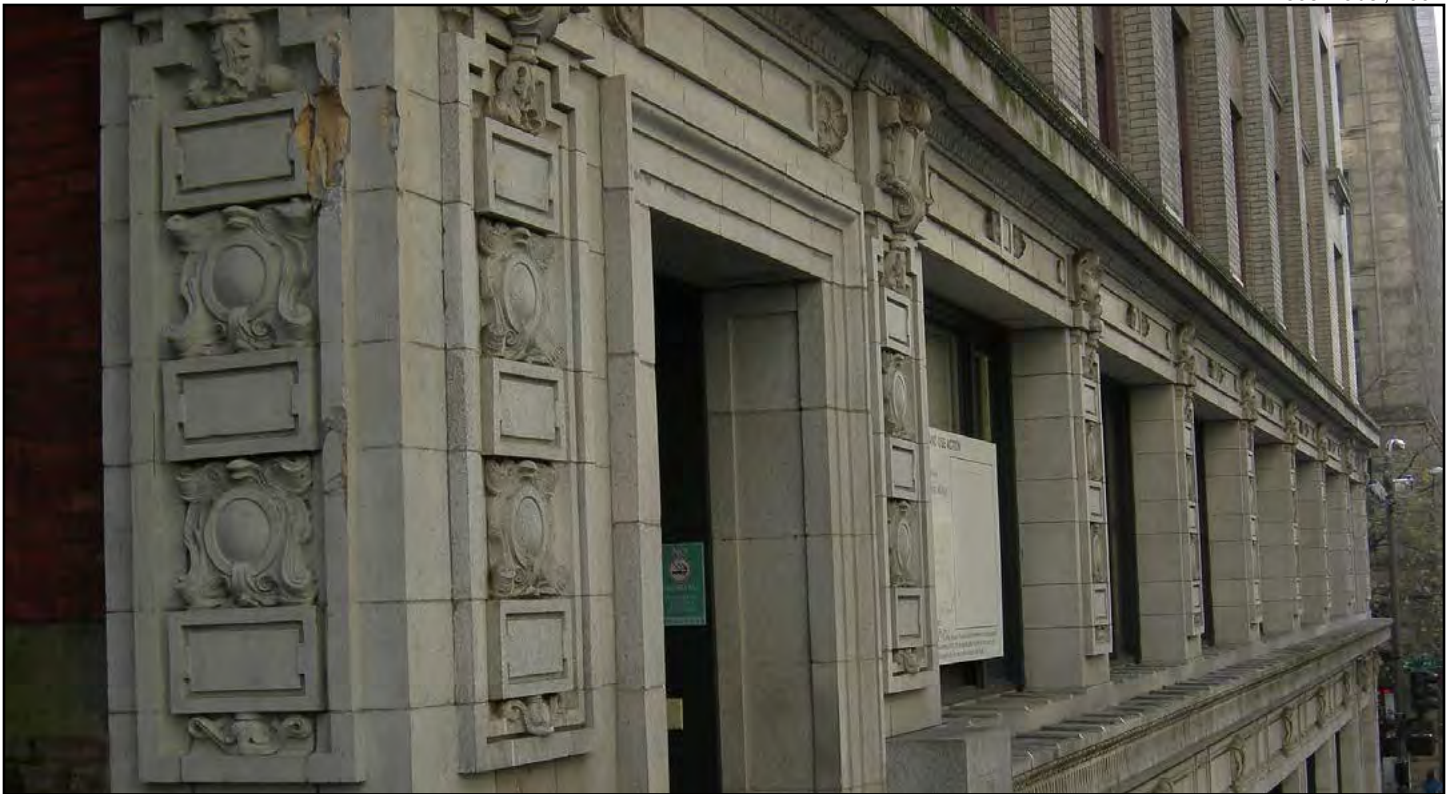
Figure 55 • Terra cotta detail on the Alaska Building (1904, Eames & Young with Saunders & Lawton, City of Seattle Landmark)
