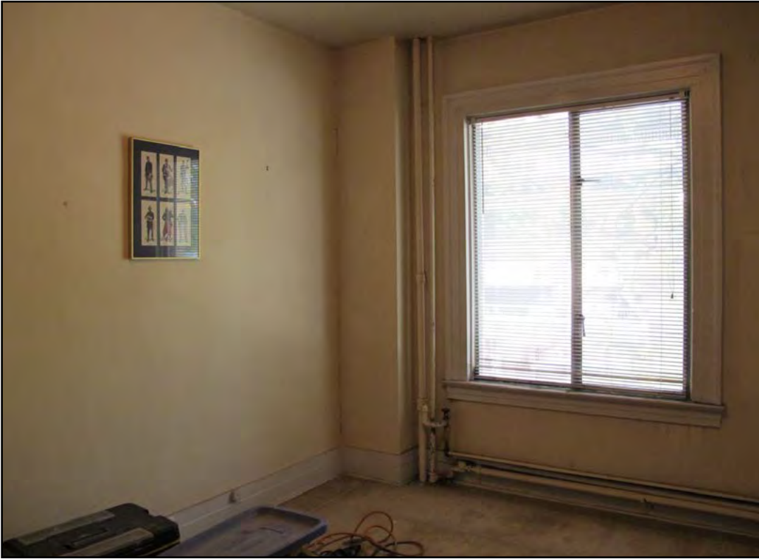
Figure 27 • Sheridan Apartment Building, typical apartment room
