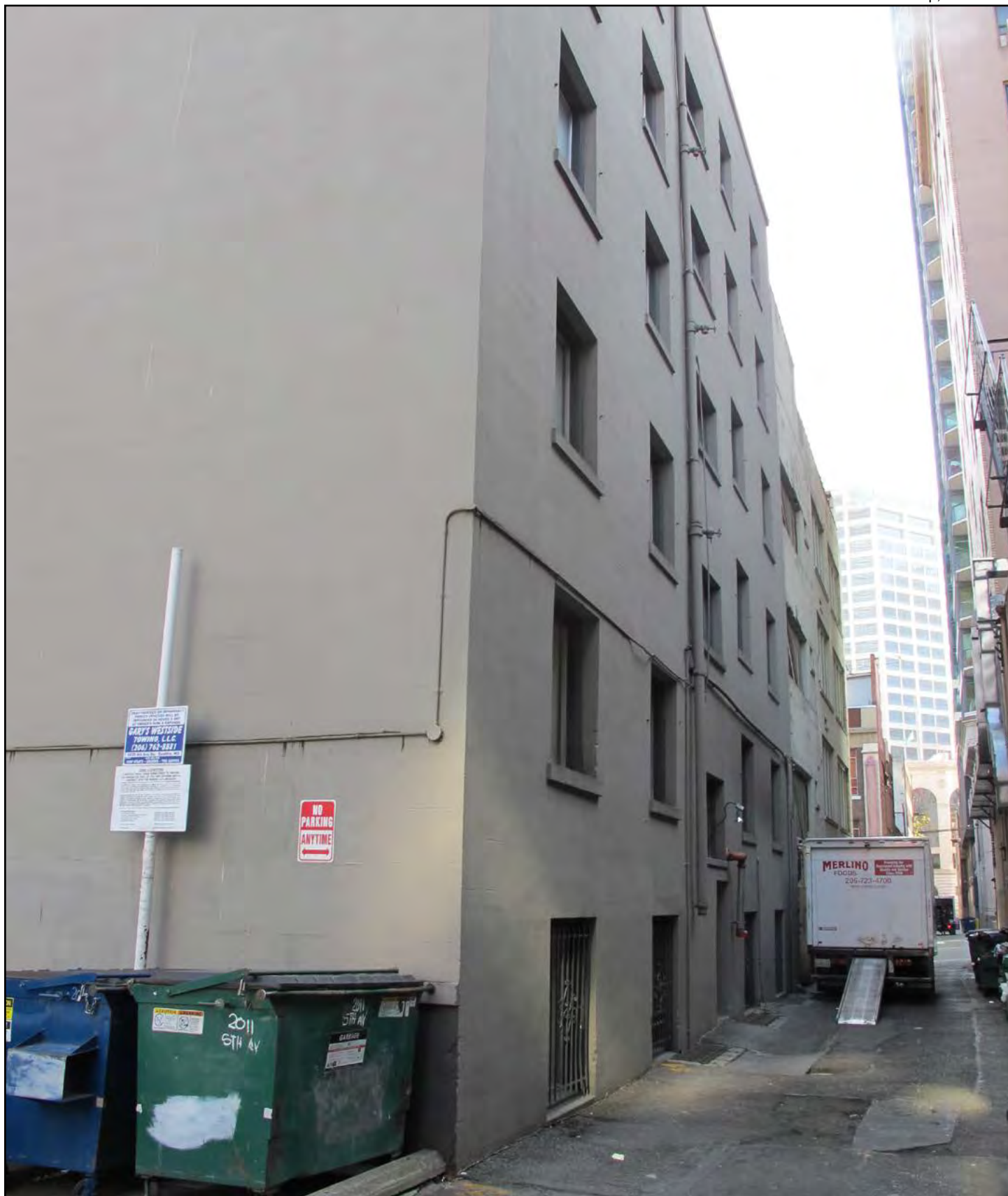
Figure 16 • Sheridan Apartment Building, western alley façade viewing south
