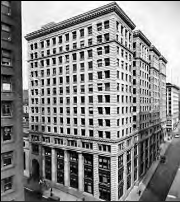
Figure 56 • Dexter Horton Building (1922, John Graham, Sr., City of Seattle Landmark)
