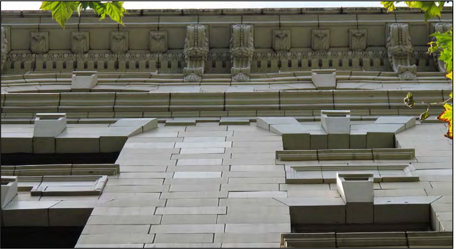
Figure 14 • Sheridan Apartment Building, detail of cornice and upper level window treatment
