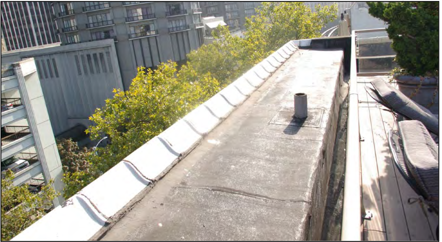
Figure 19 • Sheridan Apartment Building, detail of top of cornice on eastern façade
