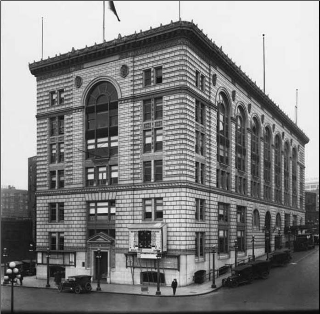
Figure 34 • Times Square Building, 1916
