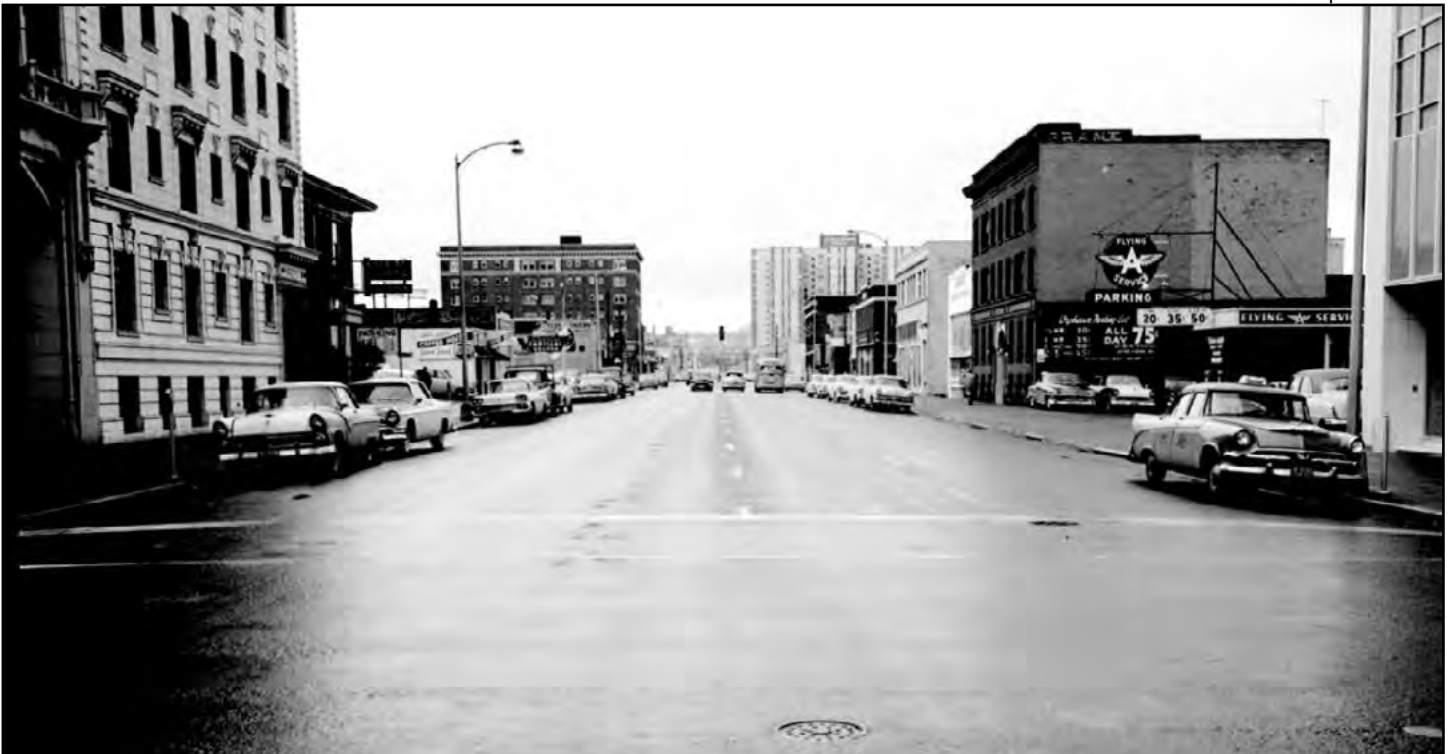
Figure 43 • Sheridan Apartment Building (far left), 1958
