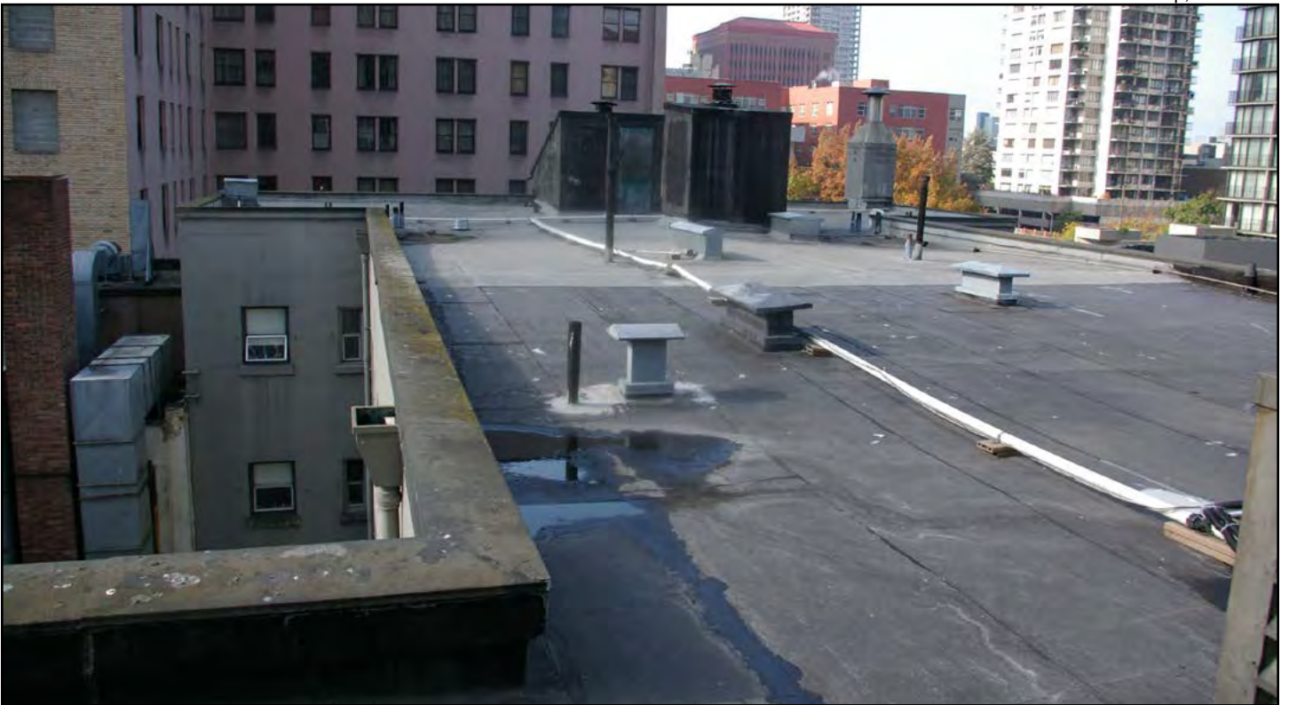
Figure 20 • Sheridan Apartment Building, roof viewing east over courtyard
