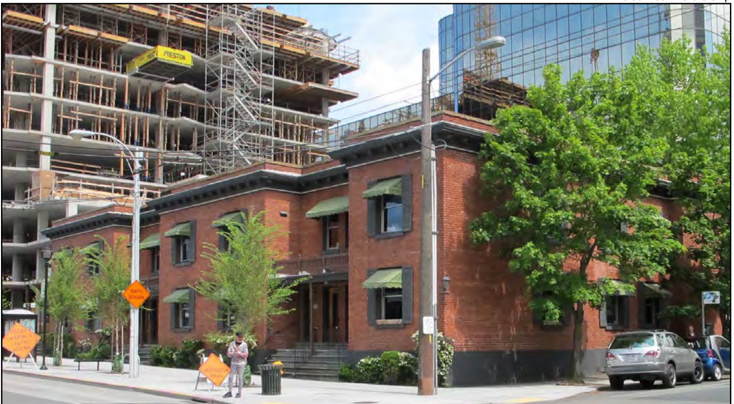
Figure 47 • Vine Court, 2600 Third Avenue (1911)
