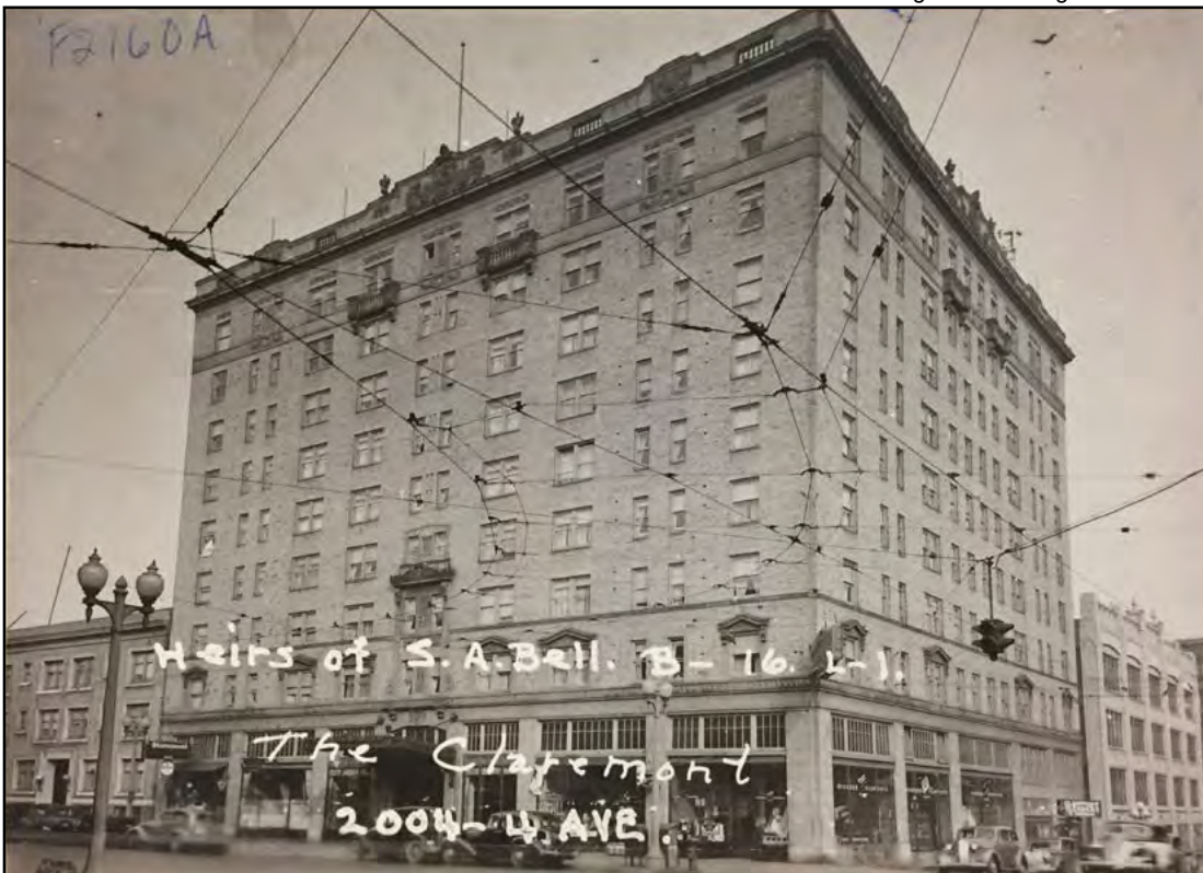
Figure 53 • The Claremont/Hotel Ändra, 2004 Fourth Avenue (1926)
