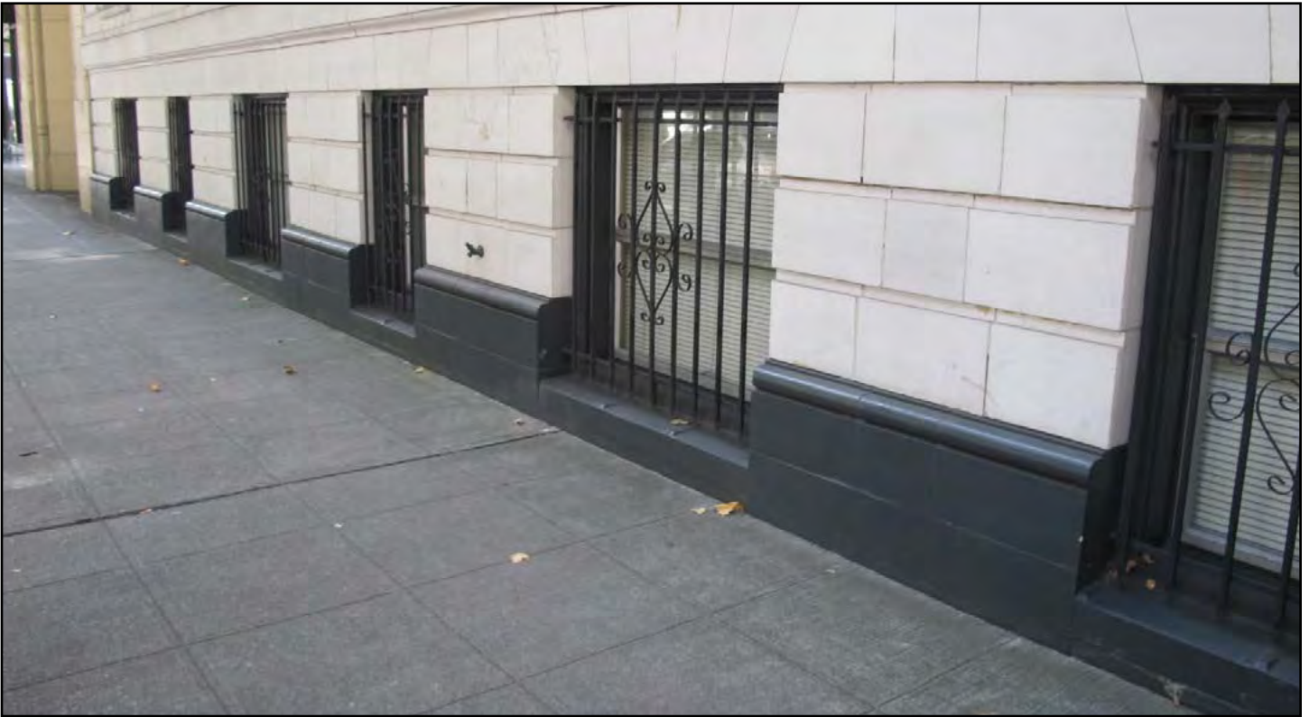
Figure 10 • Sheridan Apartment Building, detail of base of building on eastern façade
