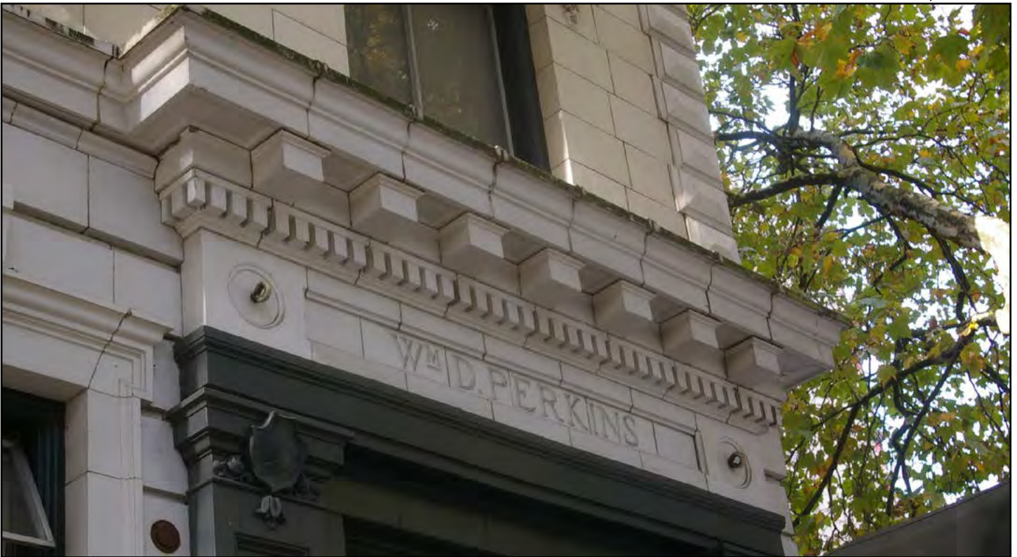
Figure 11 • Sheridan Apartment Building, detail of second floor feature window head treatment
