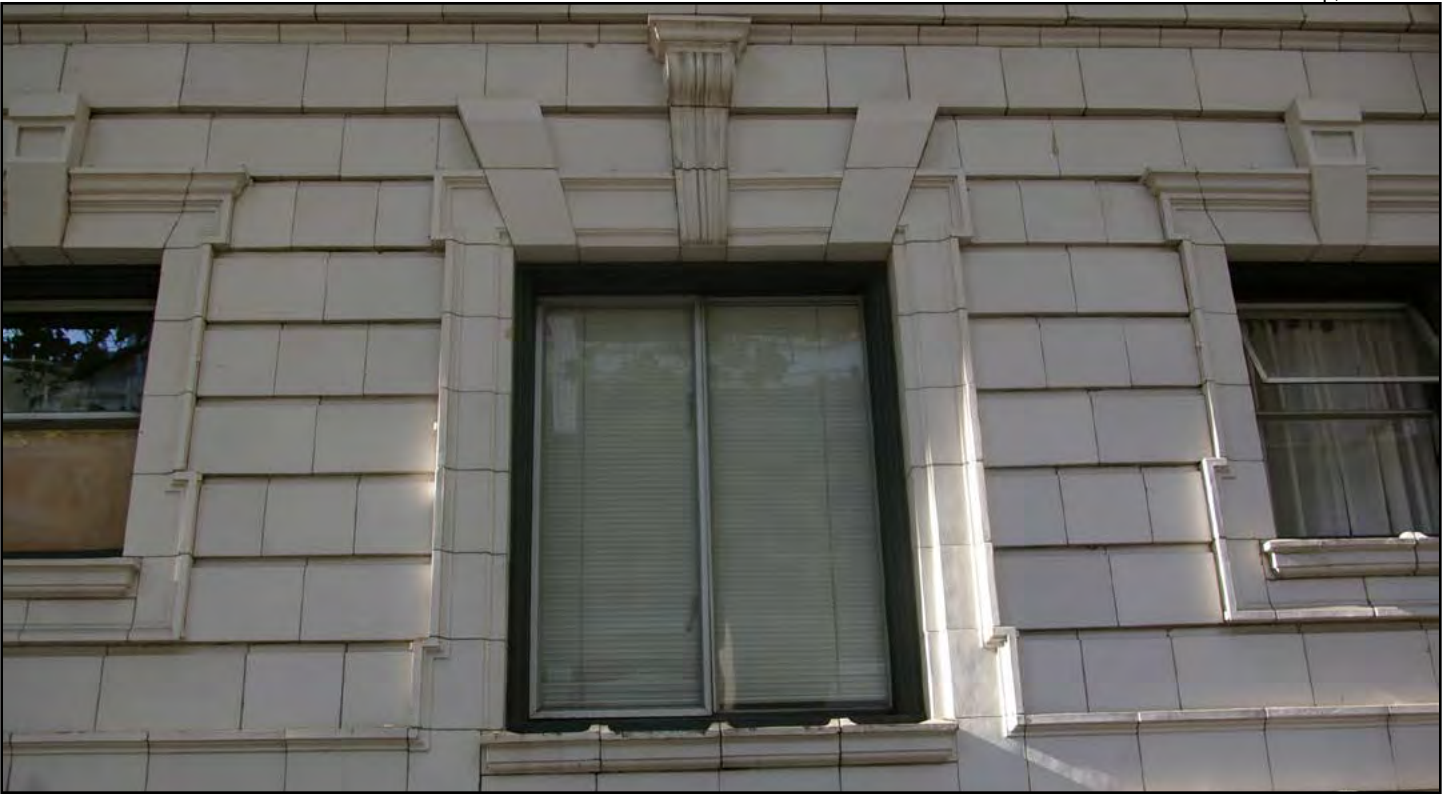
Figure 12 • Sheridan Apartment Building, detail of ground floor feature window head and trim
