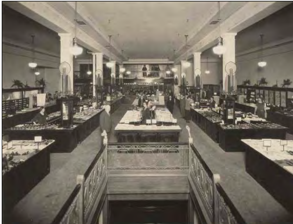
Fig. 110 – Rhodes Brothers Ten Cent Store at 1507 4 th Avenue, interior, in 1924. (MOHAI 1996.10.62)
