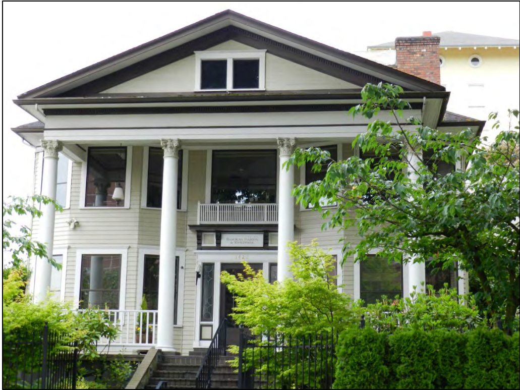
Fig. 138 – Arvesen & Lidral, contractors: Booth Undertaking Company at 1422 Bellevue Avenue (Alterations and additions, 1923). (DON)
