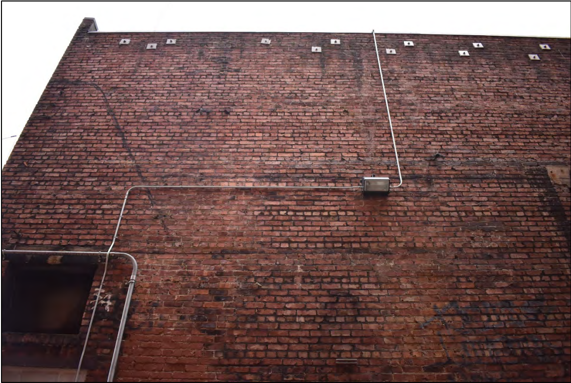
Fig. 21 – West/alley elevation, detail upper part.
