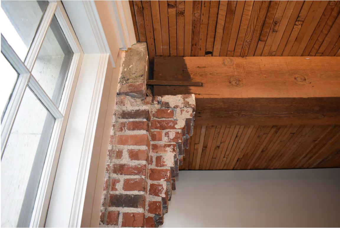
Fig. 43 – Interior, second floor office, detail wall pier
