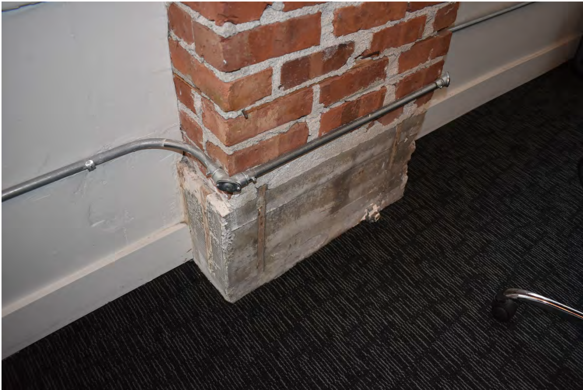
Fig. 44 – Interior, second floor office, detail wall pier
