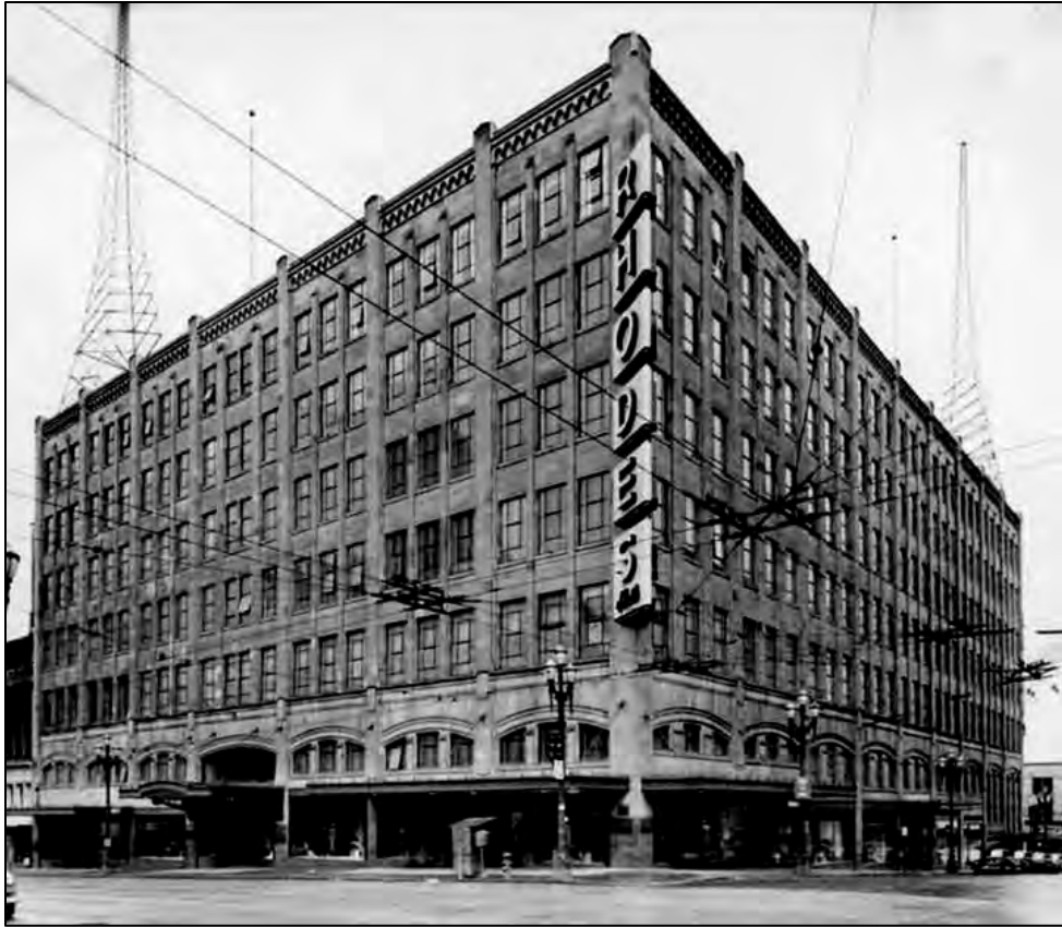
Fig. 104 –Rhodes Department Store at 2 nd & Union (Harlan Thomas, 1927, destroyed). (Puget Sound Theater Organ Society). Rhodes' radio station KFOA broadcasting towers on roof.
