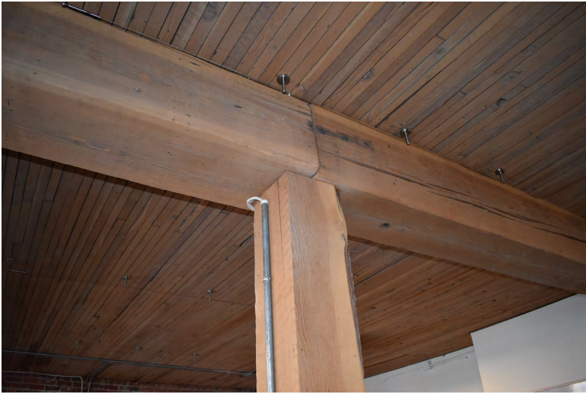
Fig. 65 – Interior, third floor office, detail structure
