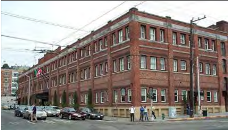
Fig. 135 – Seattle Engineering School (1918) renovated for Vance Company (Victor Voorhees, 1925). Today the building is the Marqueen Hotel at Queen Anne Avenue and Mercer Street. (DON)
