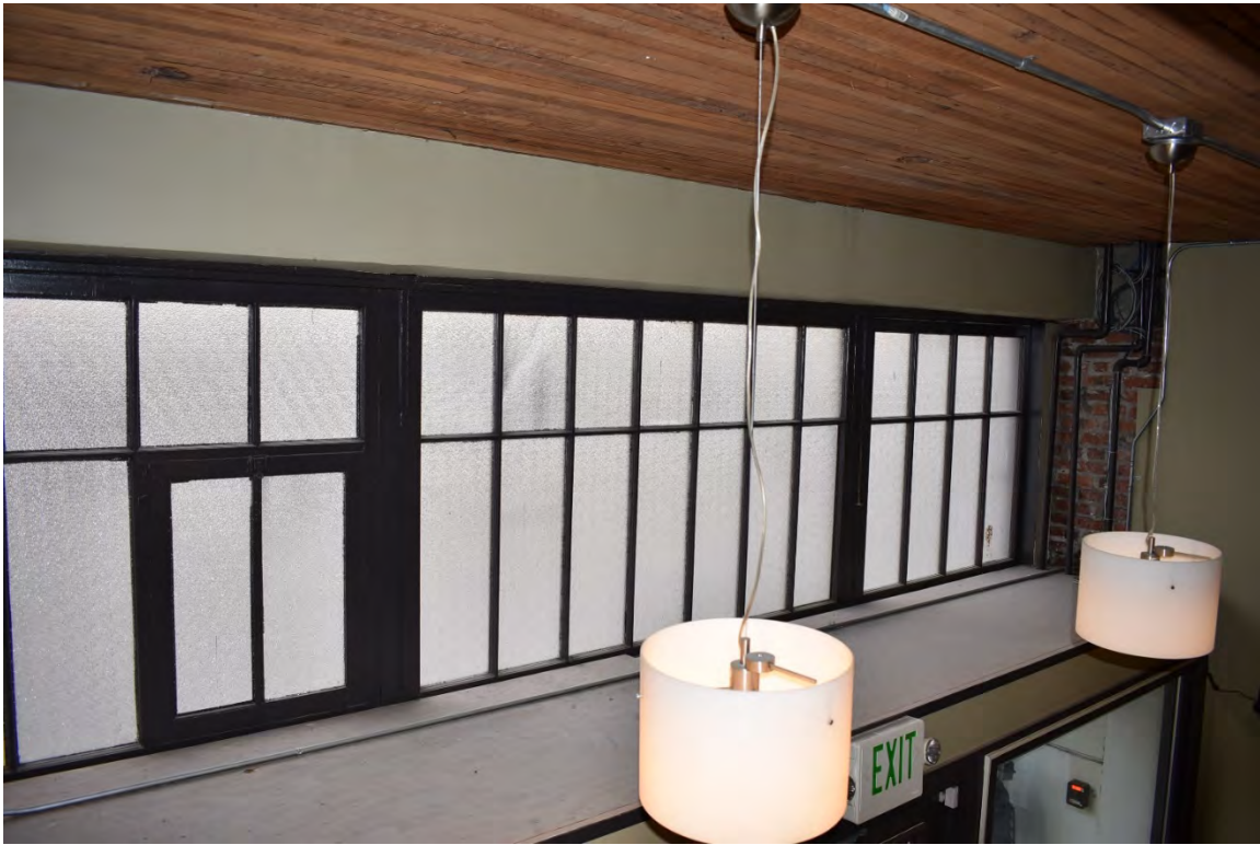
Fig. 37 – Interior, third bay, ground floor vestibule
