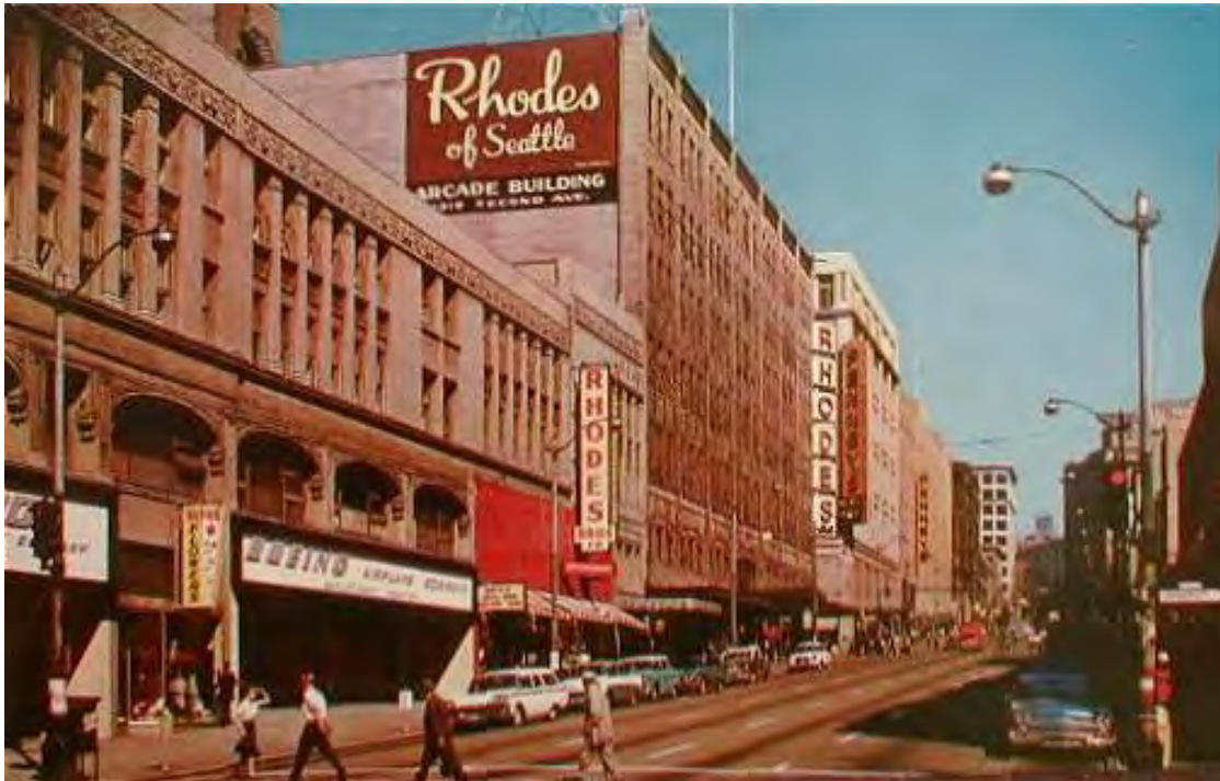
Fig. 106 – 1960s view, 2nd Avenue side of the old Arcade Building (left) and new Rhodes Department Store, which was built on the demolished northern half of the Arcade Building. (right). The block, from 1 st to 2 nd Avenues, and from University to Union Street, is now the site of the Seattle Art Museum and Russell Investments Tower.
