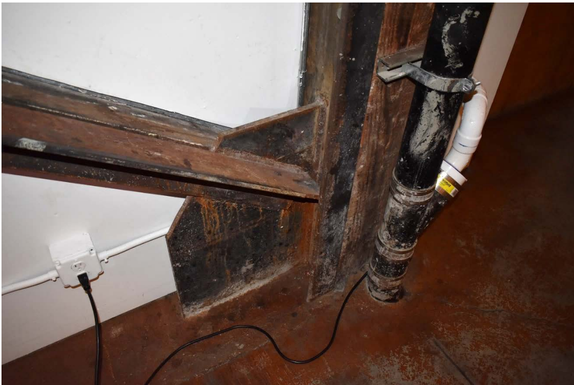
Fig. 26 – Interior, first bay, ground floor commercial space
