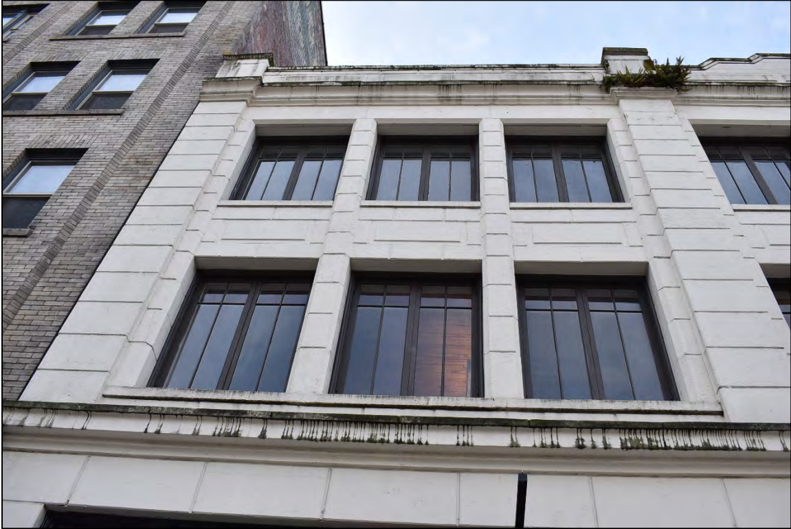
Fig. 9 – East elevation, first/left bay, upper floors
