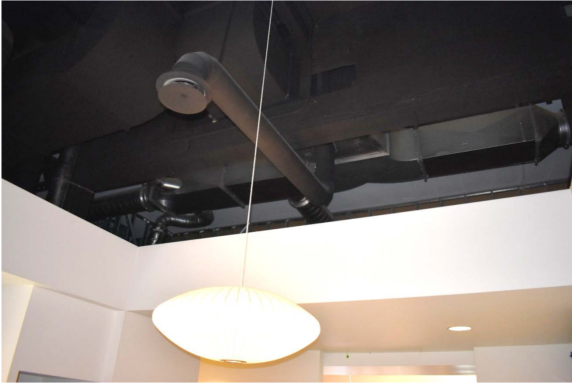
Fig. 55 – Interior, second floor office, kitchen area, actual ceiling height above kitchen
