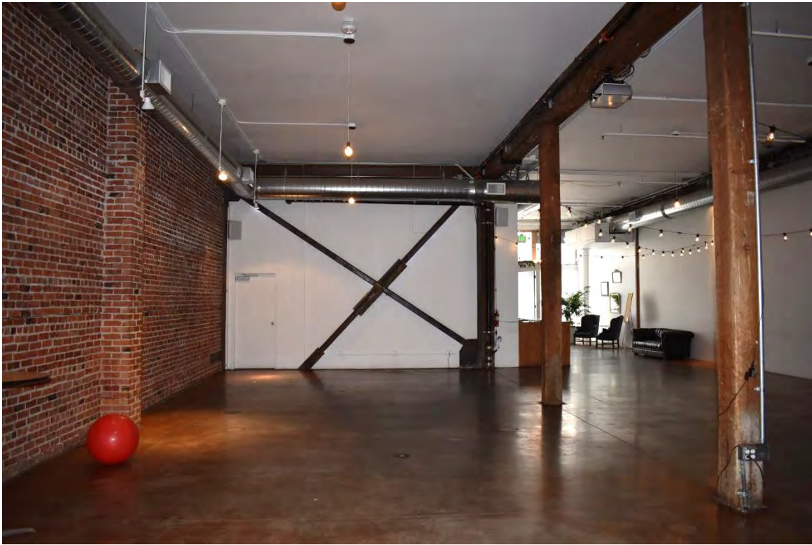
Fig. 25 – Interior, first bay, ground floor commercial space
