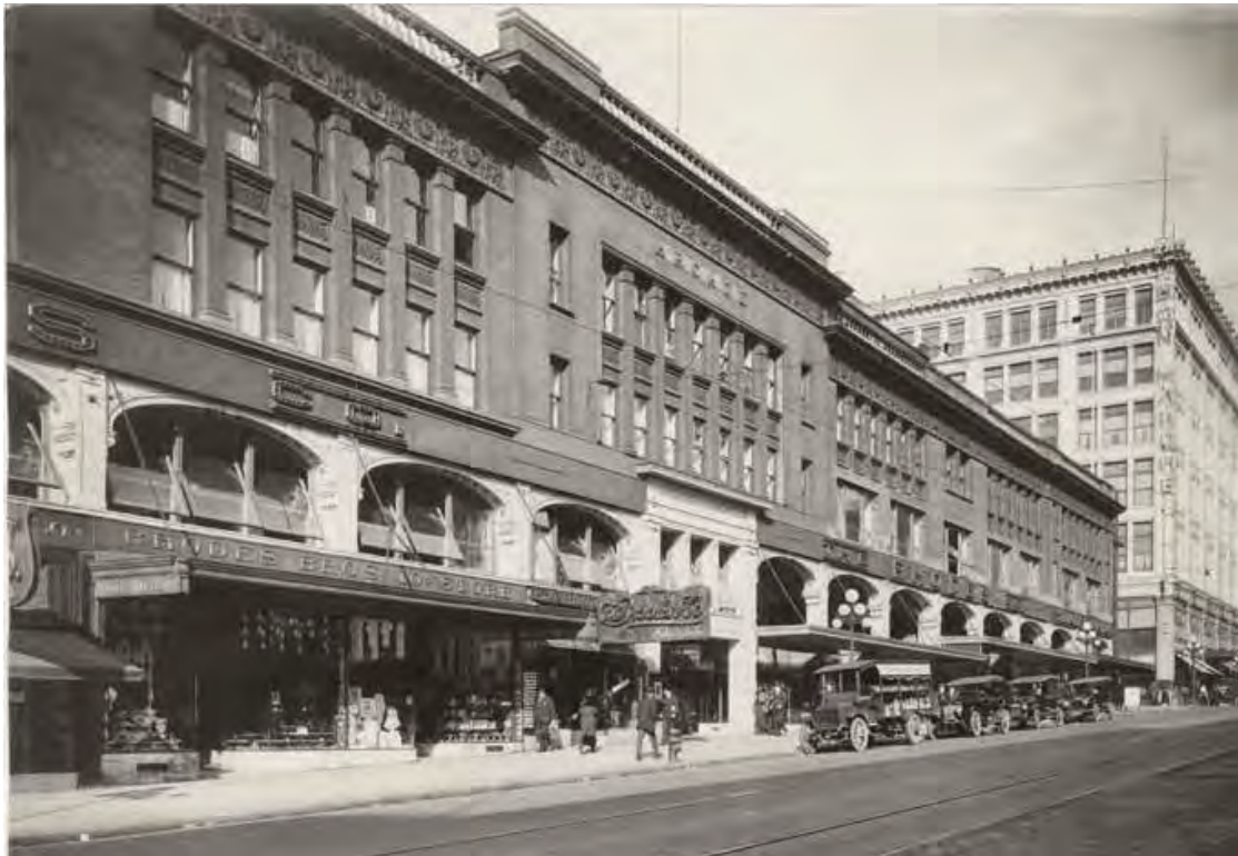
Fig. 99 – Arcade Building c.1913, after renovations to enlarge exterior arcade for Rhodes Department Store (at right in image). Destroyed. (MOHAI 1983.10.9588)
