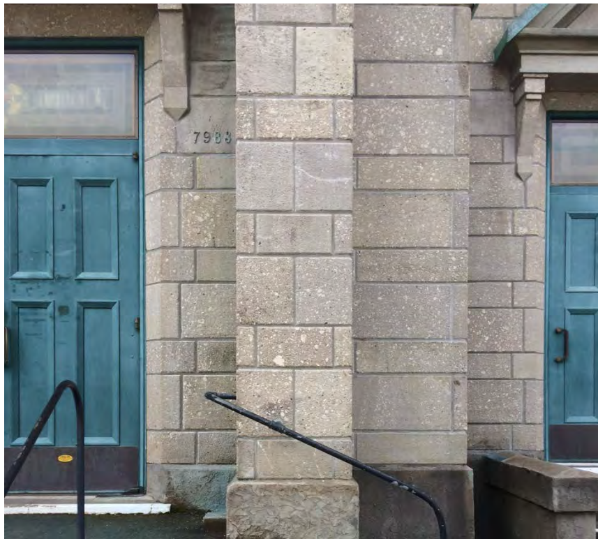
Fig. 144 – St. Agatha Catholic Church (Ernest Kroner, 1920), in Portland, Oregon, detail of exterior wall. (Lauren Deming)
