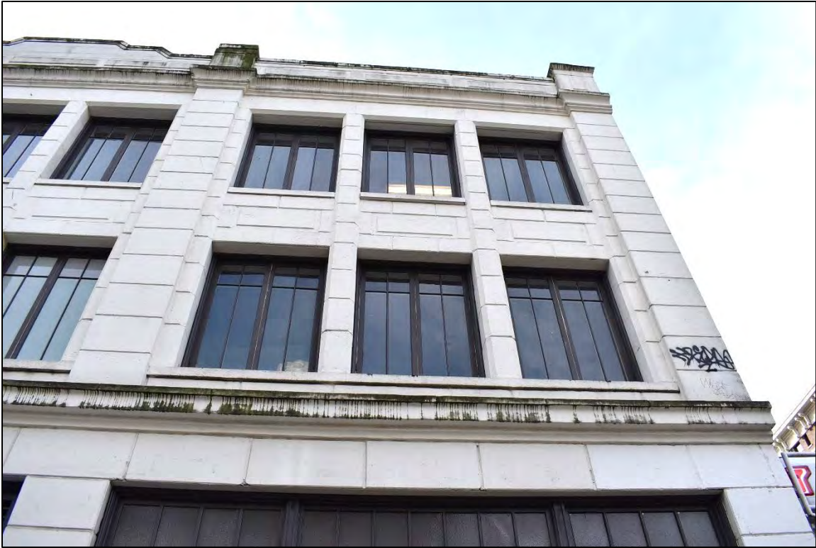
Fig. 13 – East elevation, third/right bay, upper floors
