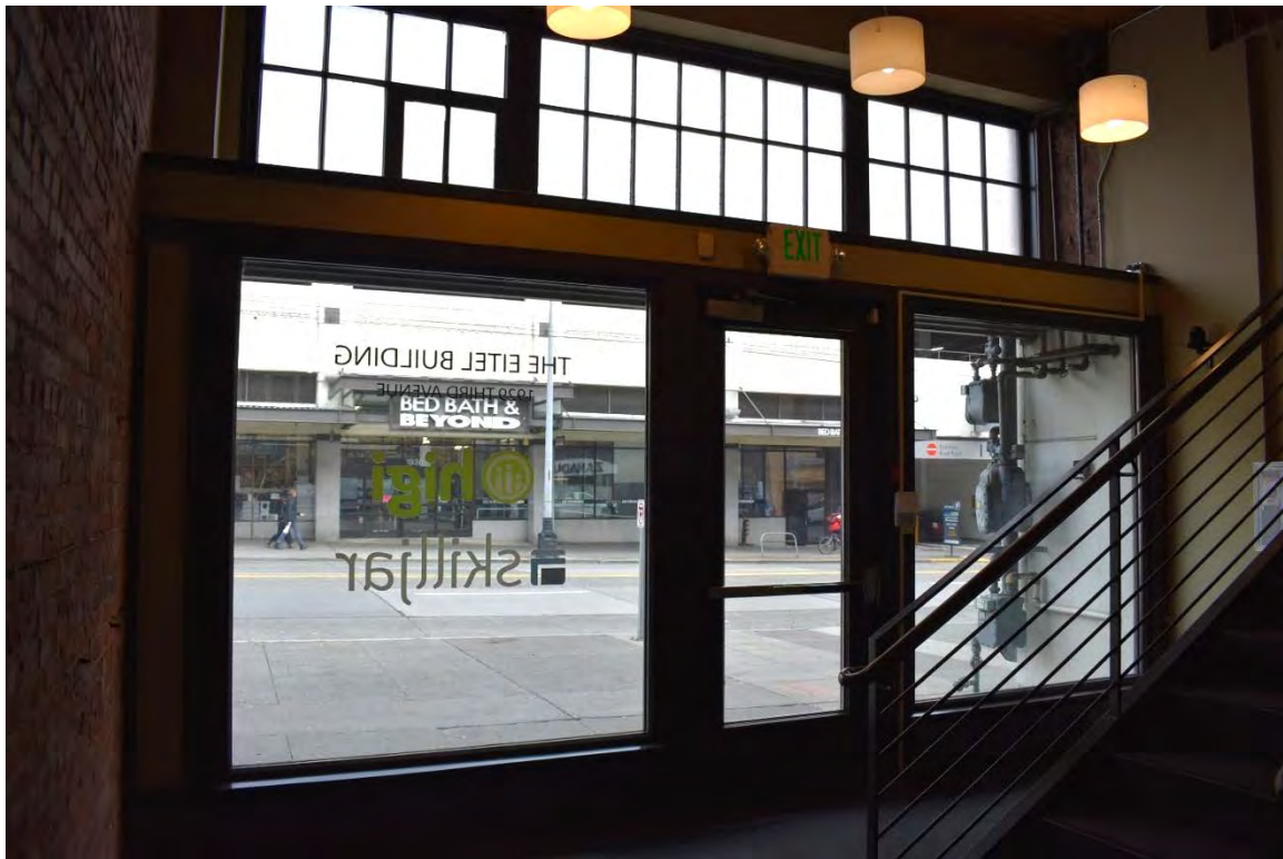
Fig. 36 – Interior, third bay, ground floor vestibule
