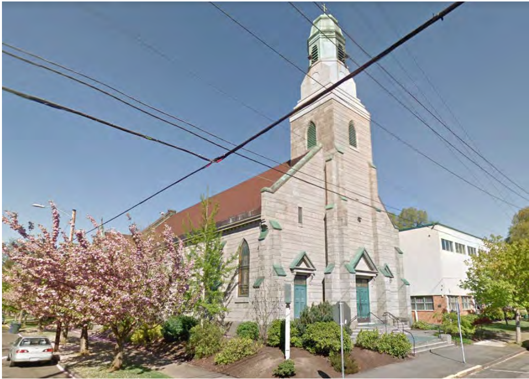
Fig. 143 – St. Agatha Catholic Church (Ernest Kroner, 1920), in Portland, Oregon, constructed with stone from the Mount Angel Quarry. (Google Streetview)
