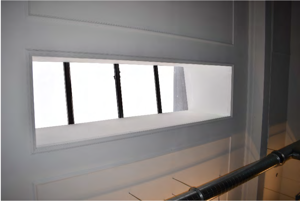
Fig. 53 – Interior, second floor office, central space, detail skylight
