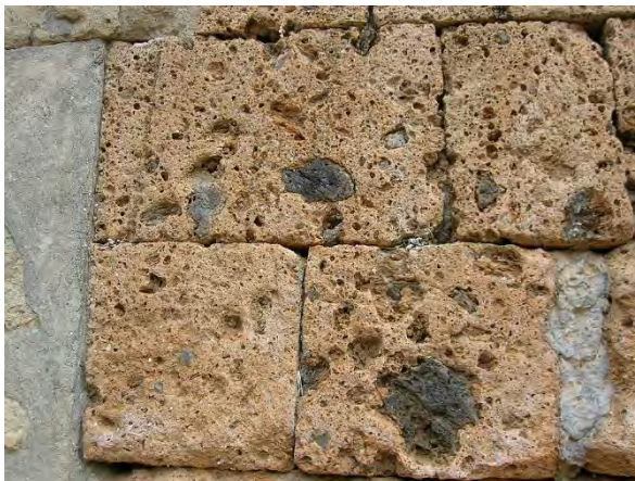
Fig. 142 – (Left) Sample of tuff, from Italy; (Right) Subject building front façade upper left window, detail of 1937 tax photo, when façade was unpainted. Tuff varies widely by texture and color. Tuff cladding the subject building was quarried in Mount Angel, Oregon.
