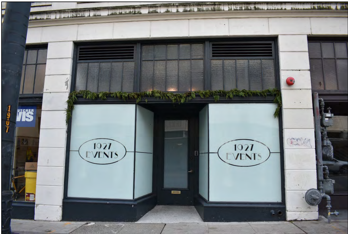
Fig. 12 – East elevation, second/middle bay, ground floor
