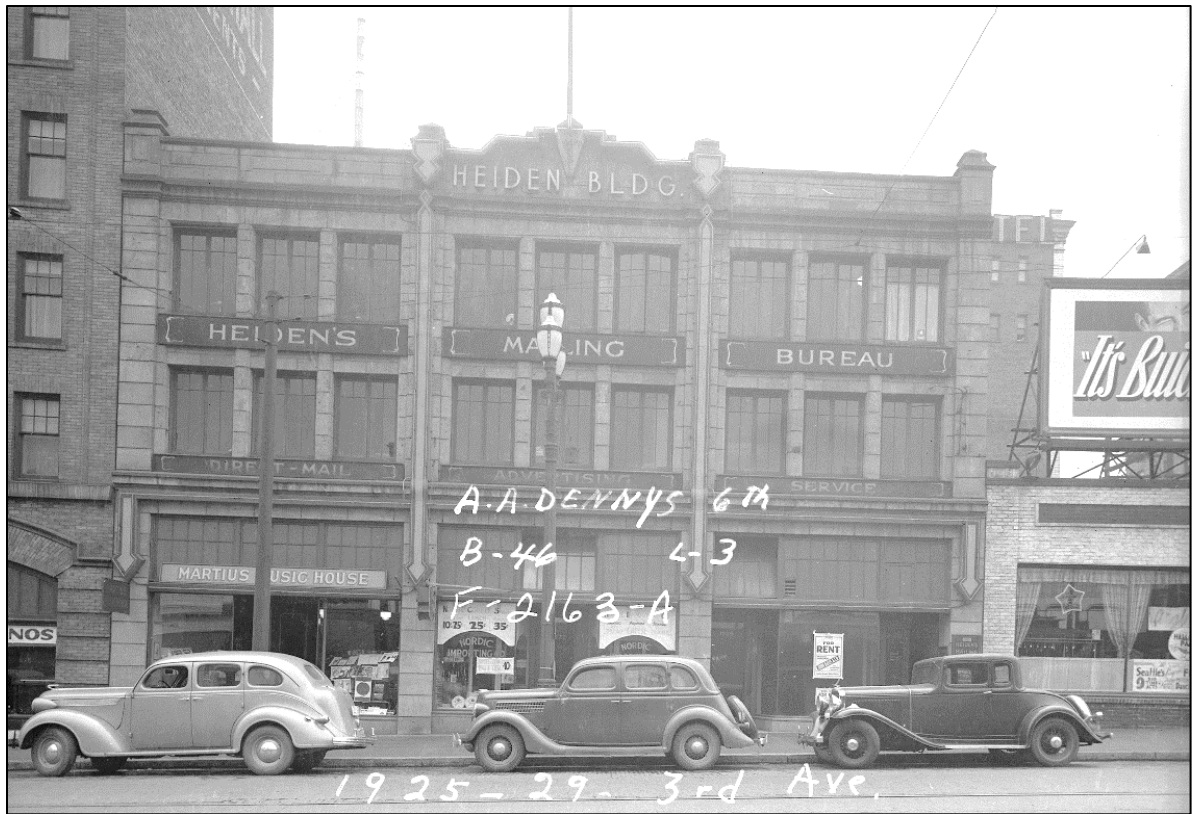
Fig. 87 – 1937 view of the subject building. (PSRA, original poor)
