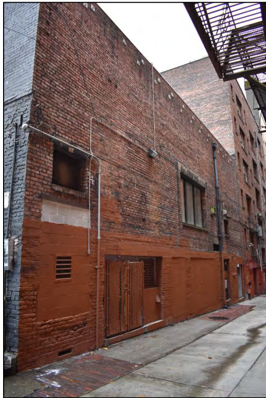
Fig. 18 – West/alley elevation, view southwards
