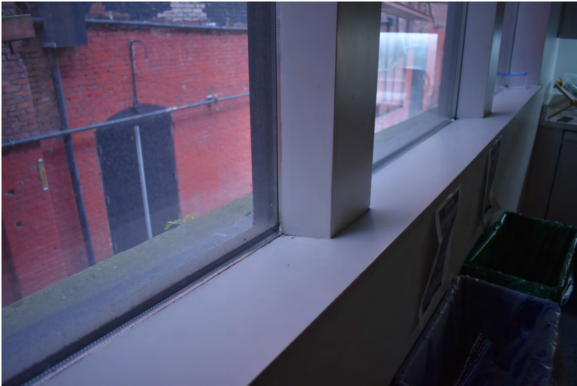
Fig. 56 – Interior, second floor office, central space, alley window
