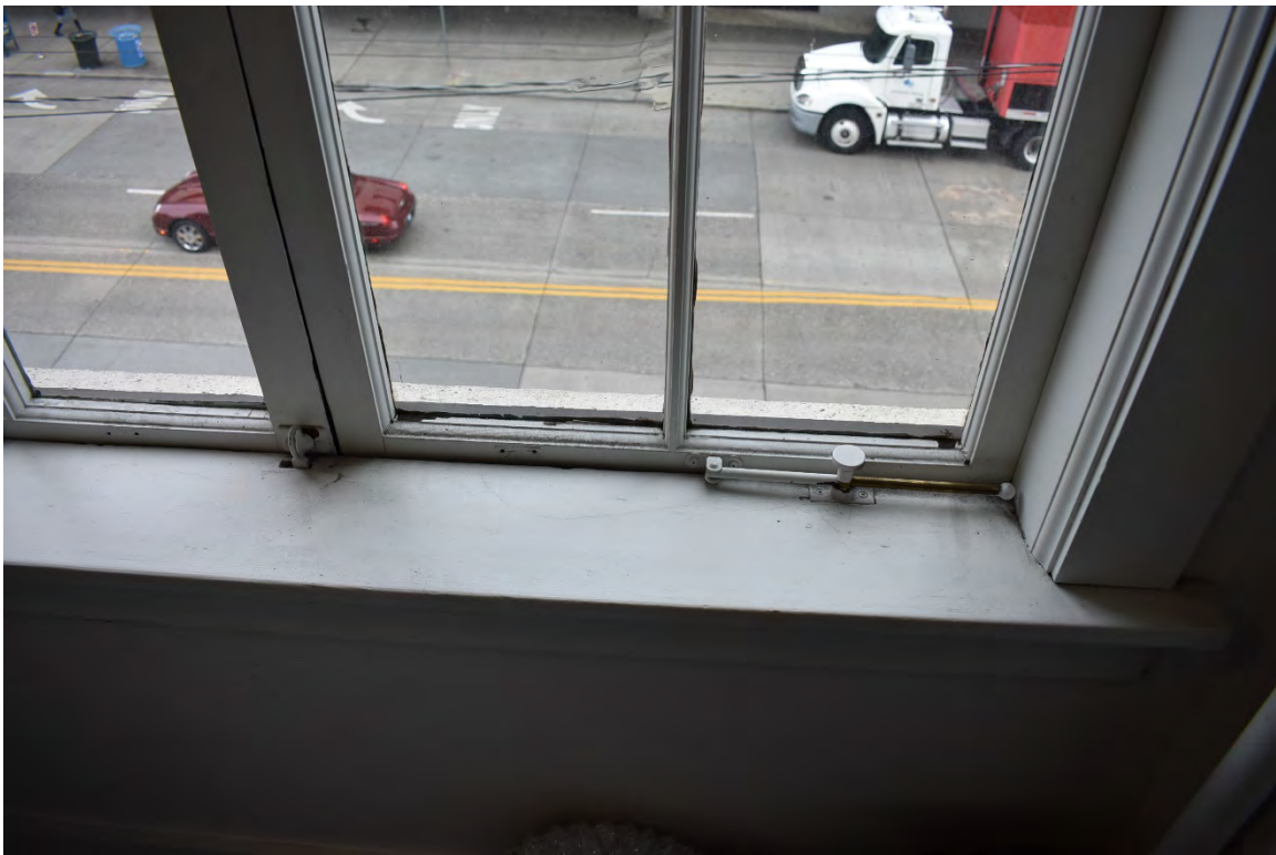
Fig. 64 – Interior, third floor office
