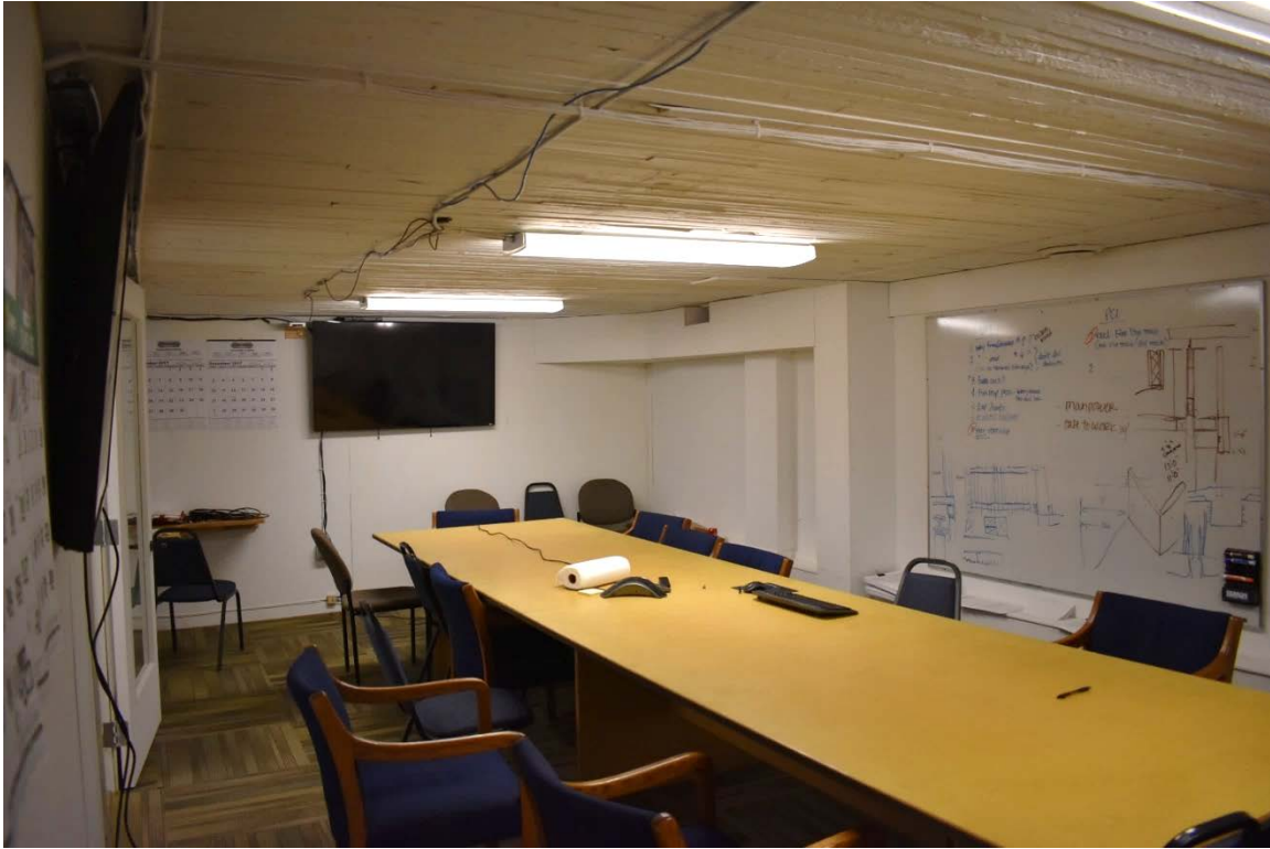
Fig. 31 – Interior, second bay, ground floor commercial space
