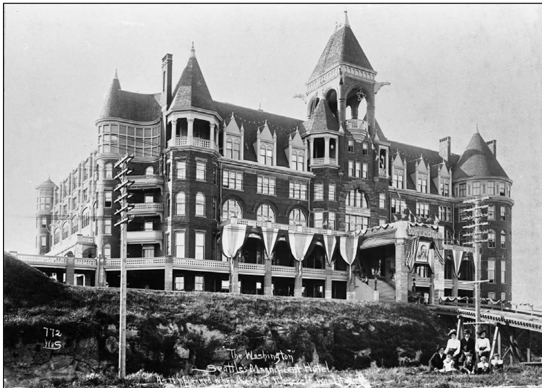
Fig. 72 – 1903 view of front of the Washington (Denny) Hotel. (MOHAI 1983.10.6708)
