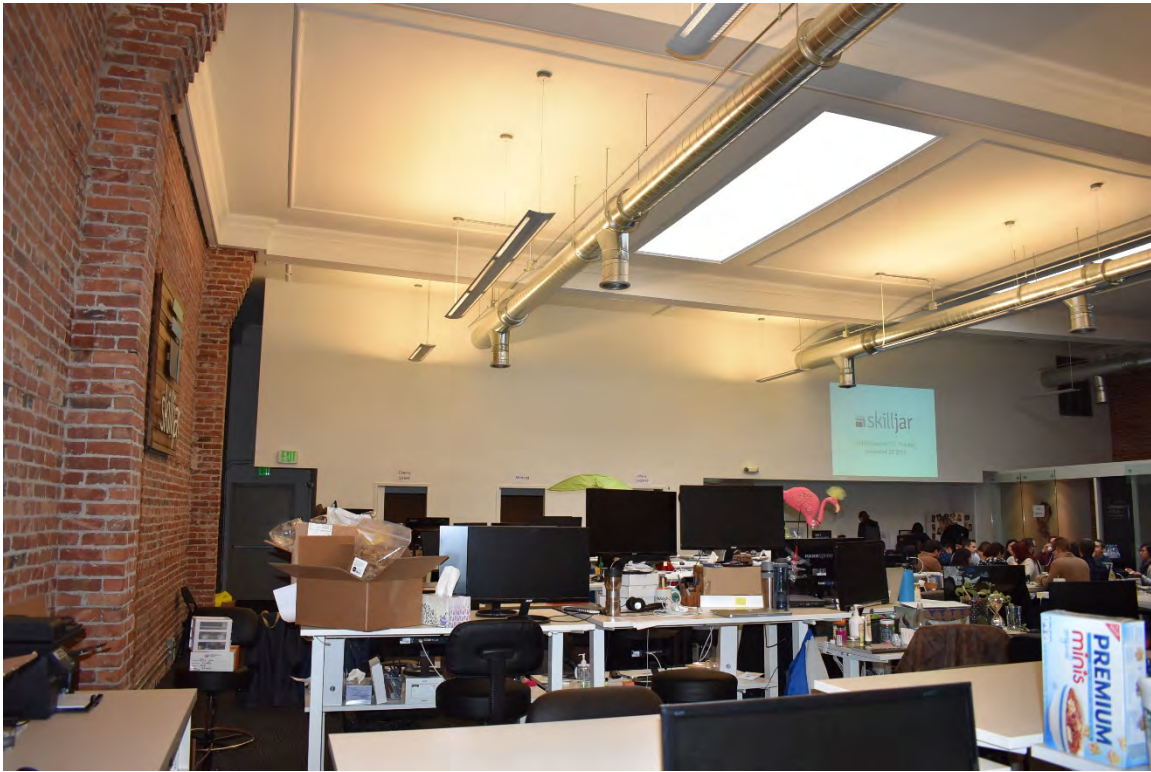
Fig. 47 – Interior, second floor office, central space
