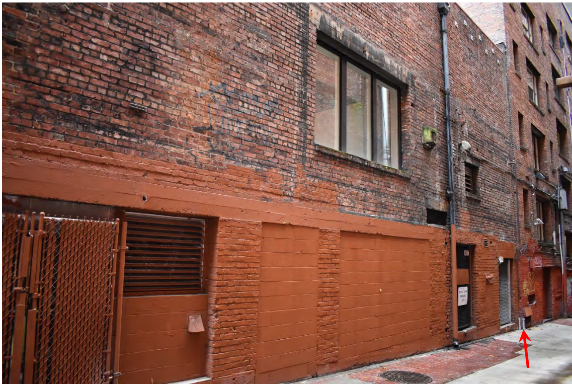
Fig. 20 – West/alley elevation, detail lower part, view southwards. Arrow indicates property line.
