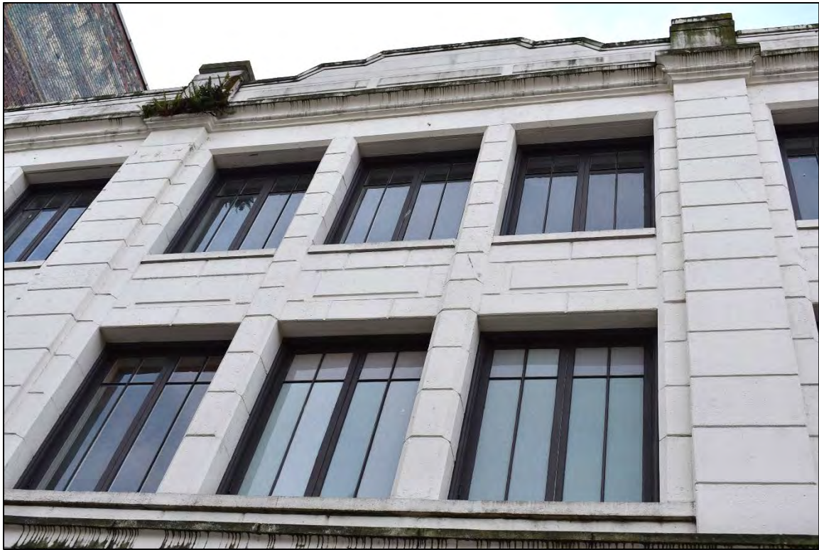
Fig. 11 – East elevation, second/middle bay, upper floors
