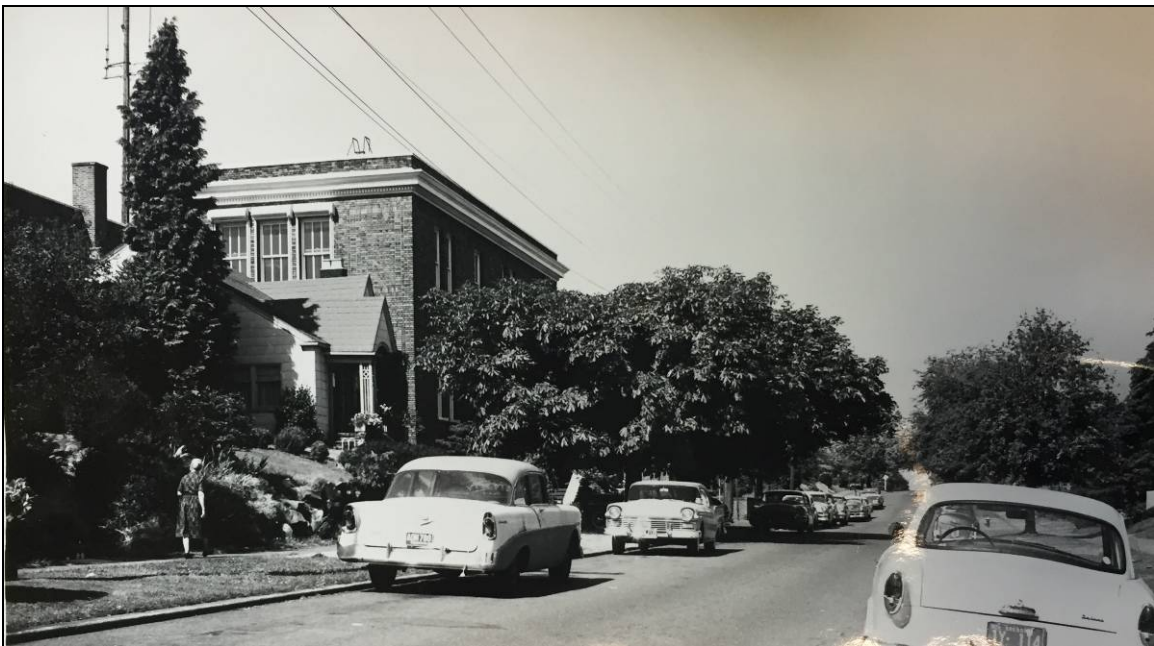
Figure 22. Below, a view looking northwest on 4 th Avenue W at the partial south and east facade. The horse chestnut trees that obscures the front is situated in the parking strip in front of the neighboring residence to the south of the Exchange building (Museum of Communications).
