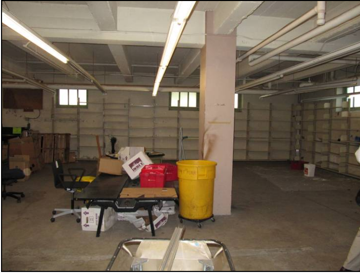
Figure 51. Left, a view looking north in the basement.
