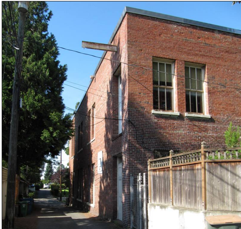
Figure 40. Below, the back door on the west facade.
