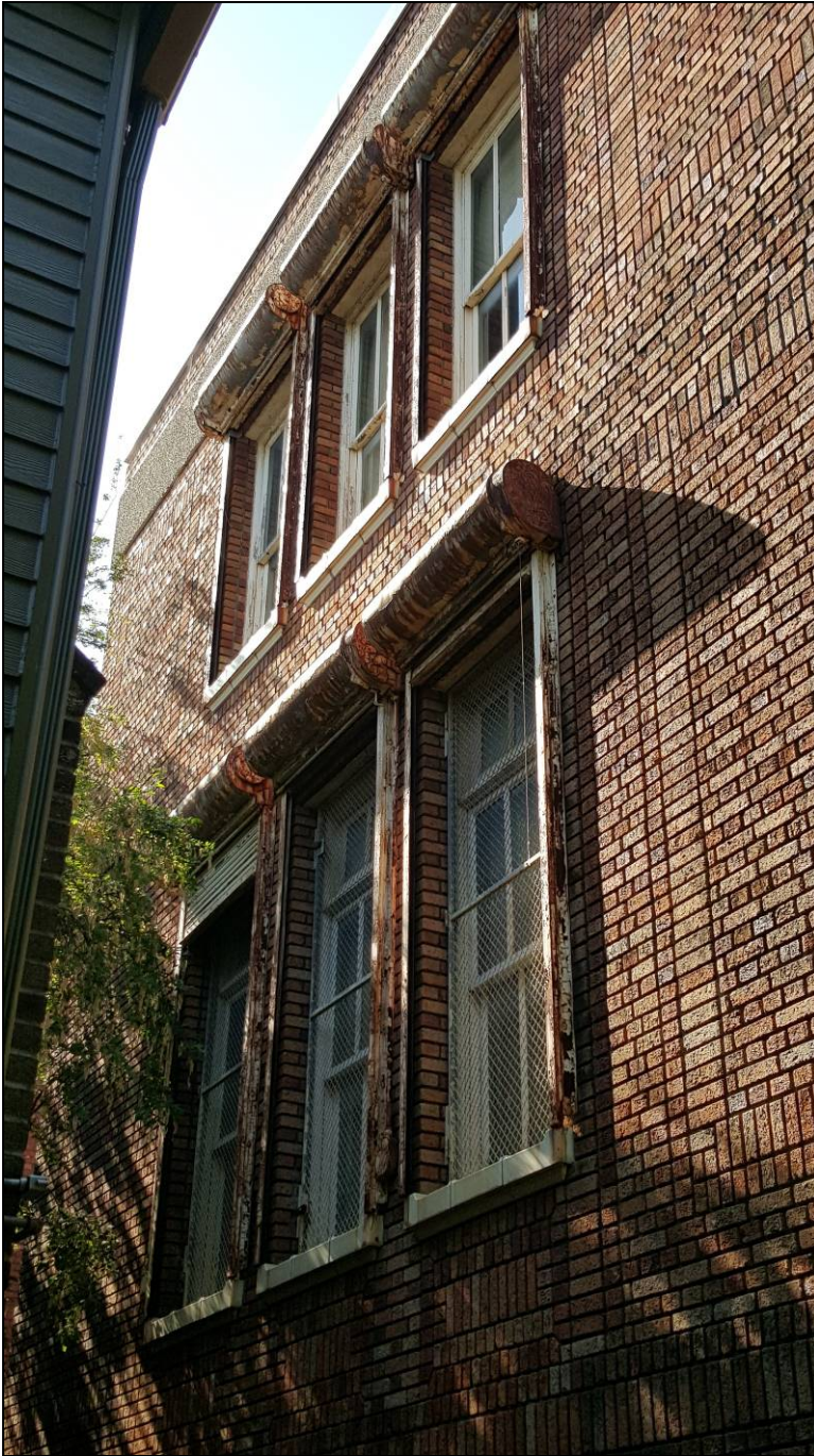
Figure 45. Above, looking west at the eastern portion of the south facade.
