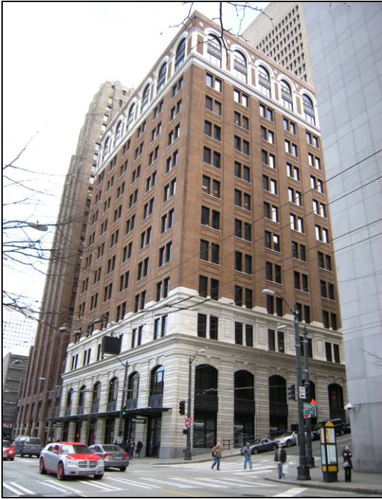
Figure 14. Right, the Pacific Telephone and Telegraph building at 1200 3rd Avenue in downtown Seattle, was built in 1921 and 1926. This view, from 2008, is looking northeast on 3 rd Avenue (Wikimedia Commons, Joe Mabel, photographer).
