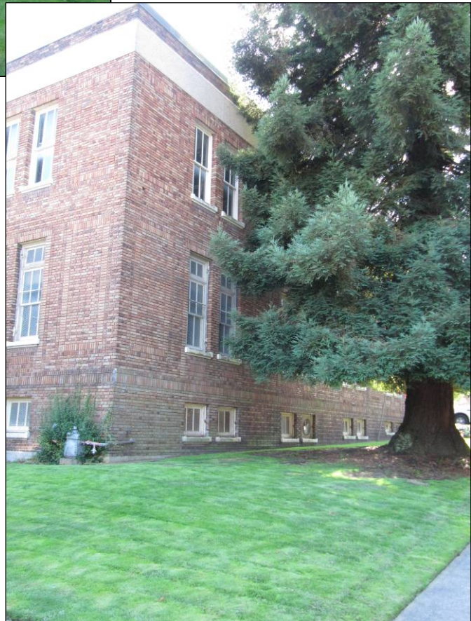
Figure 36. Right, an oblique view of the north facade (looking southwest).
