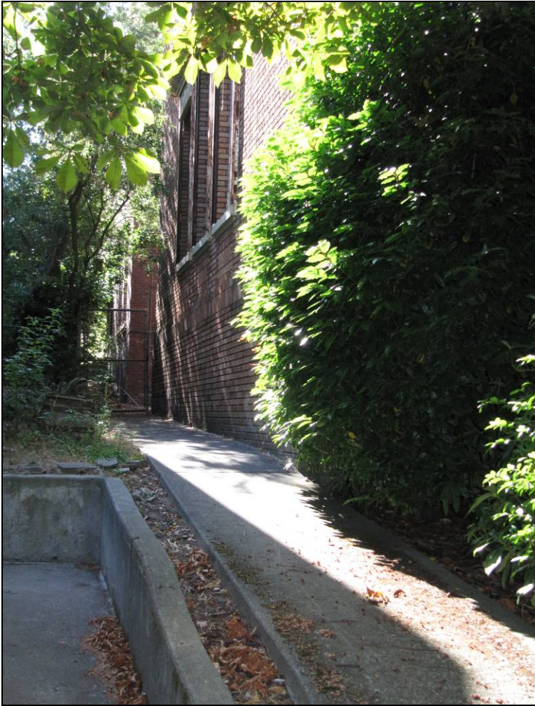
Figure 46. Left, looking west at the south facade.
