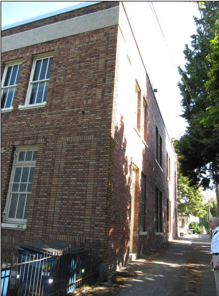
Figure 37. Above, looking northeast at the lower level masonry and grade along the north facade and the northeast corner.
