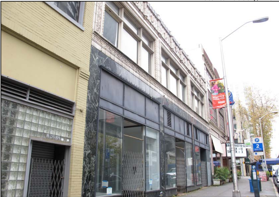
Figure 14 • National Cash Register Building, eastern façade
