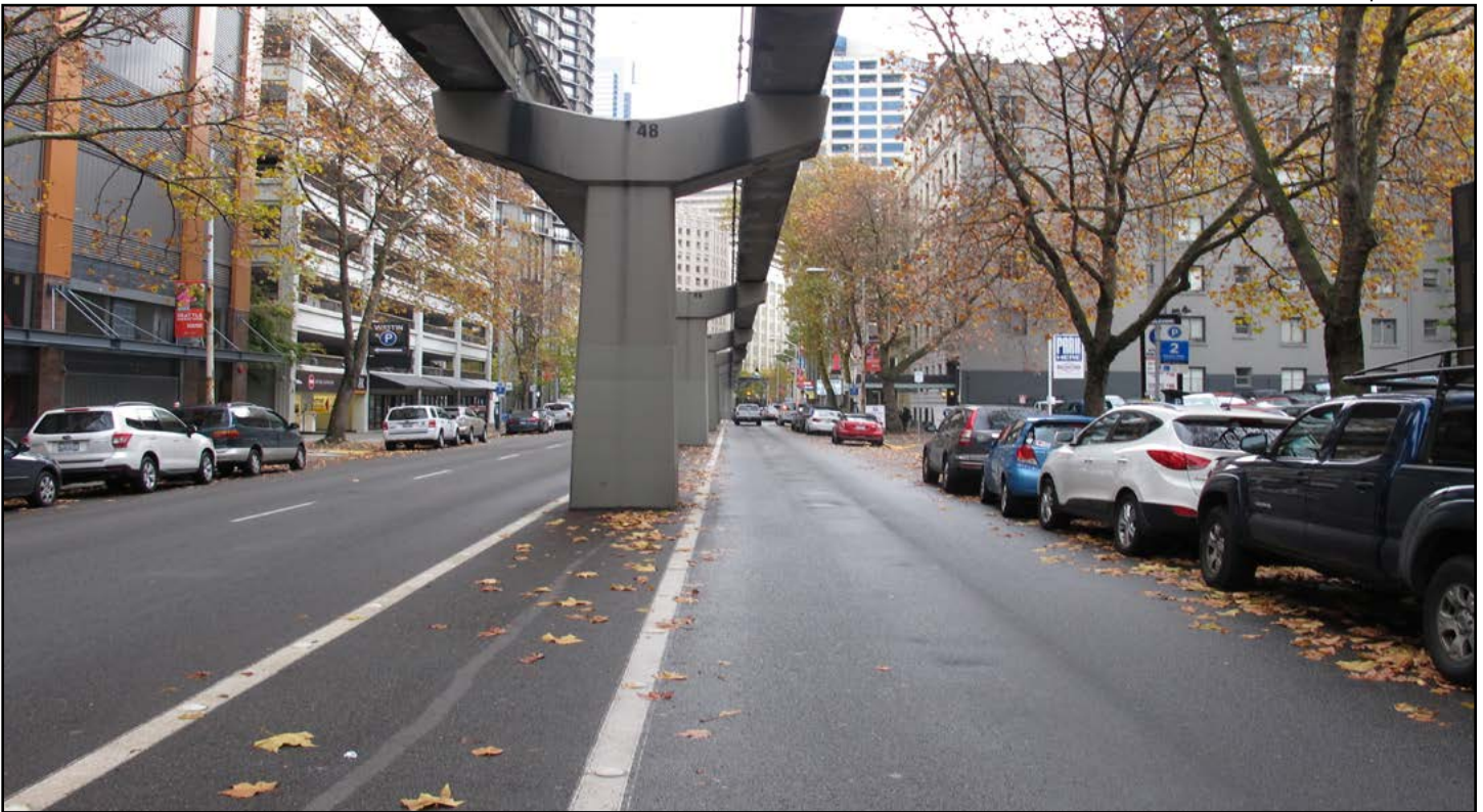
Figure 8 • View D, viewing southeast on Fifth Avenue
