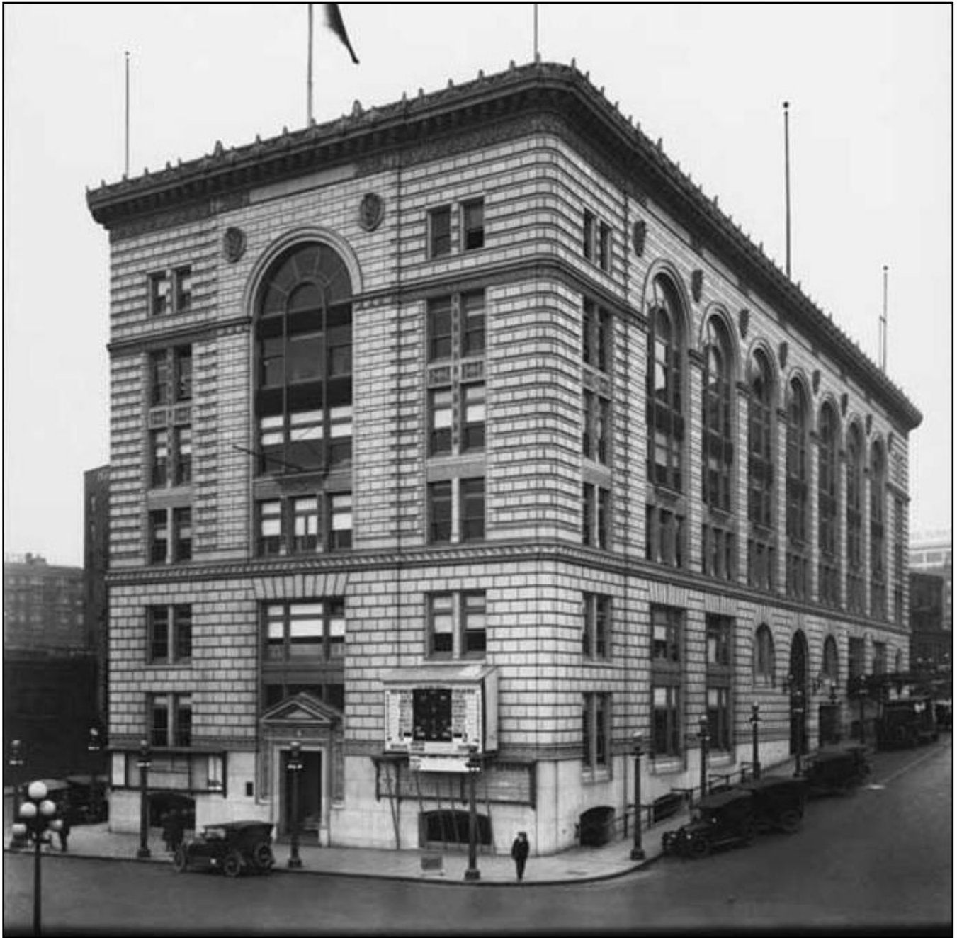
Figure 30 • Times Square Building, 1916
