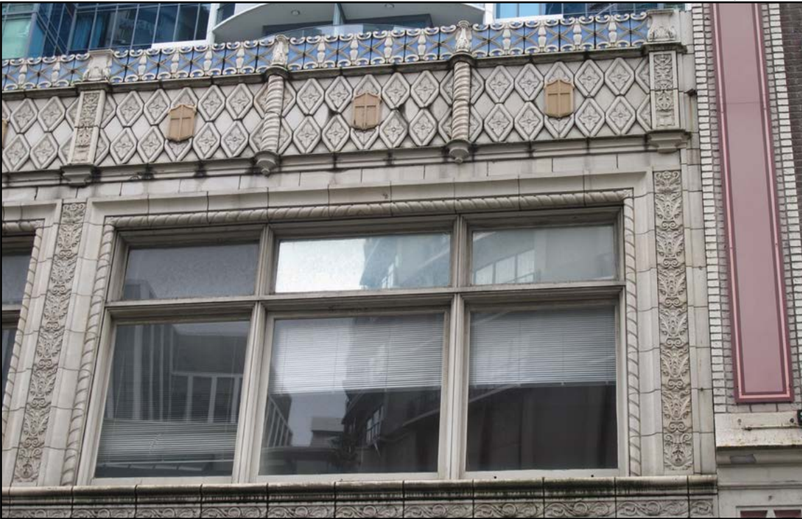
Figure 20 • Second floor windows with terra cotta tiles
