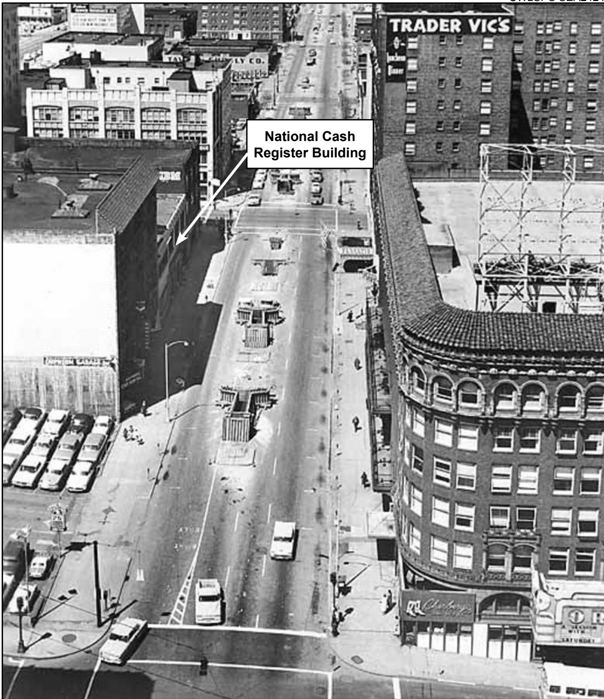
Figure 35 • Monorail Construction, Fifth Avenue, 1961
