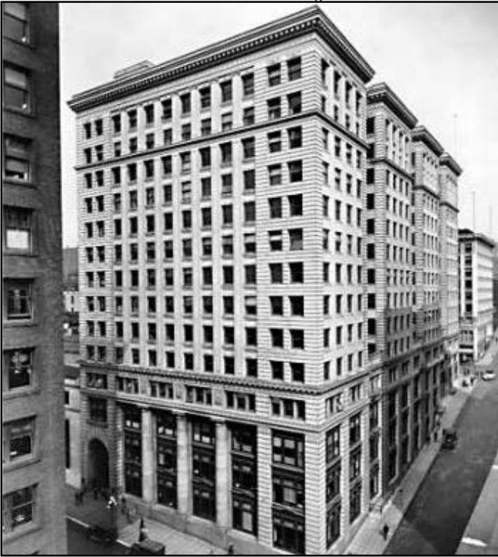
Figure 41 • Dexter Horton Building, John Graham, Sr., 1922
