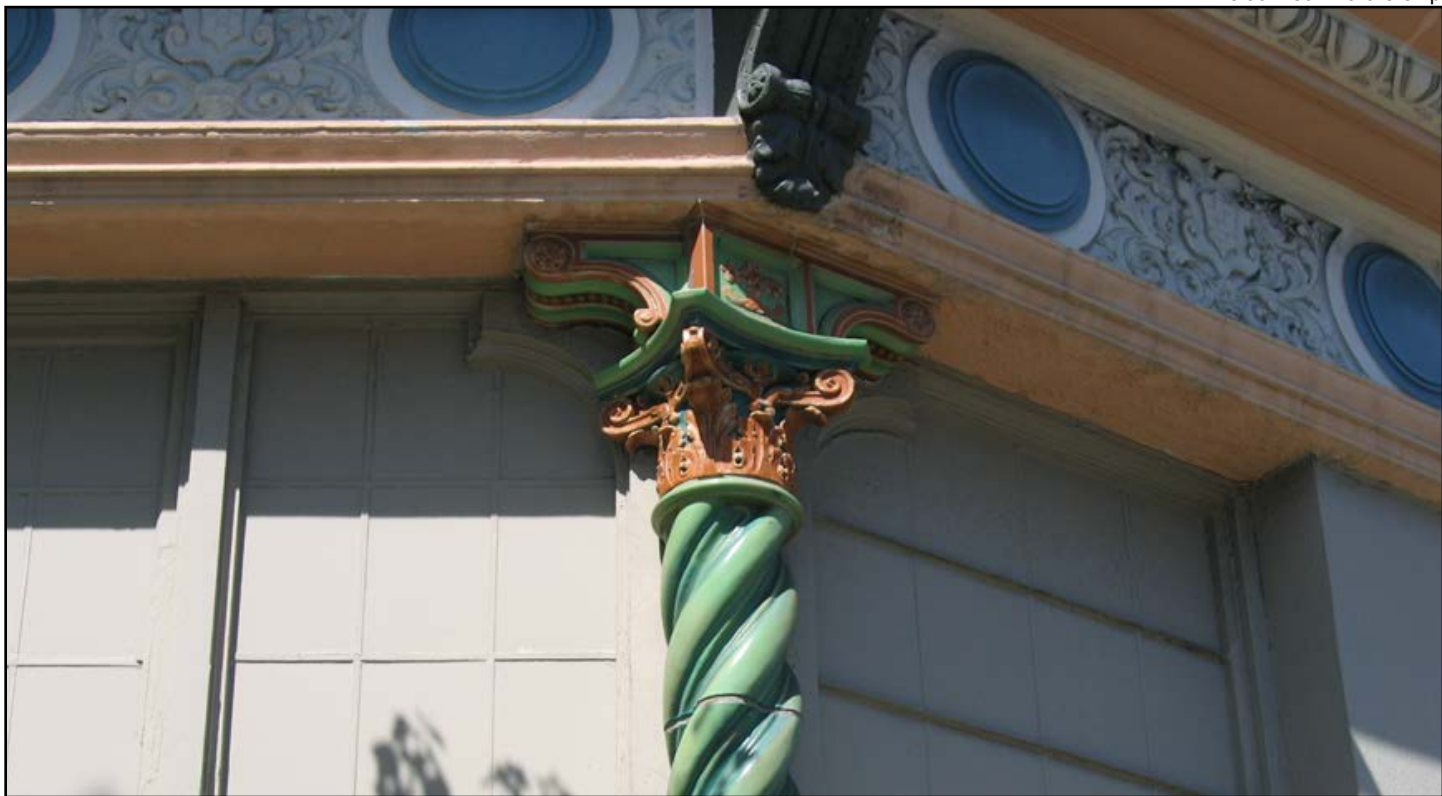
Figure 46 • Eldridge Buick Co. Building, detail of polychrome terra cotta
