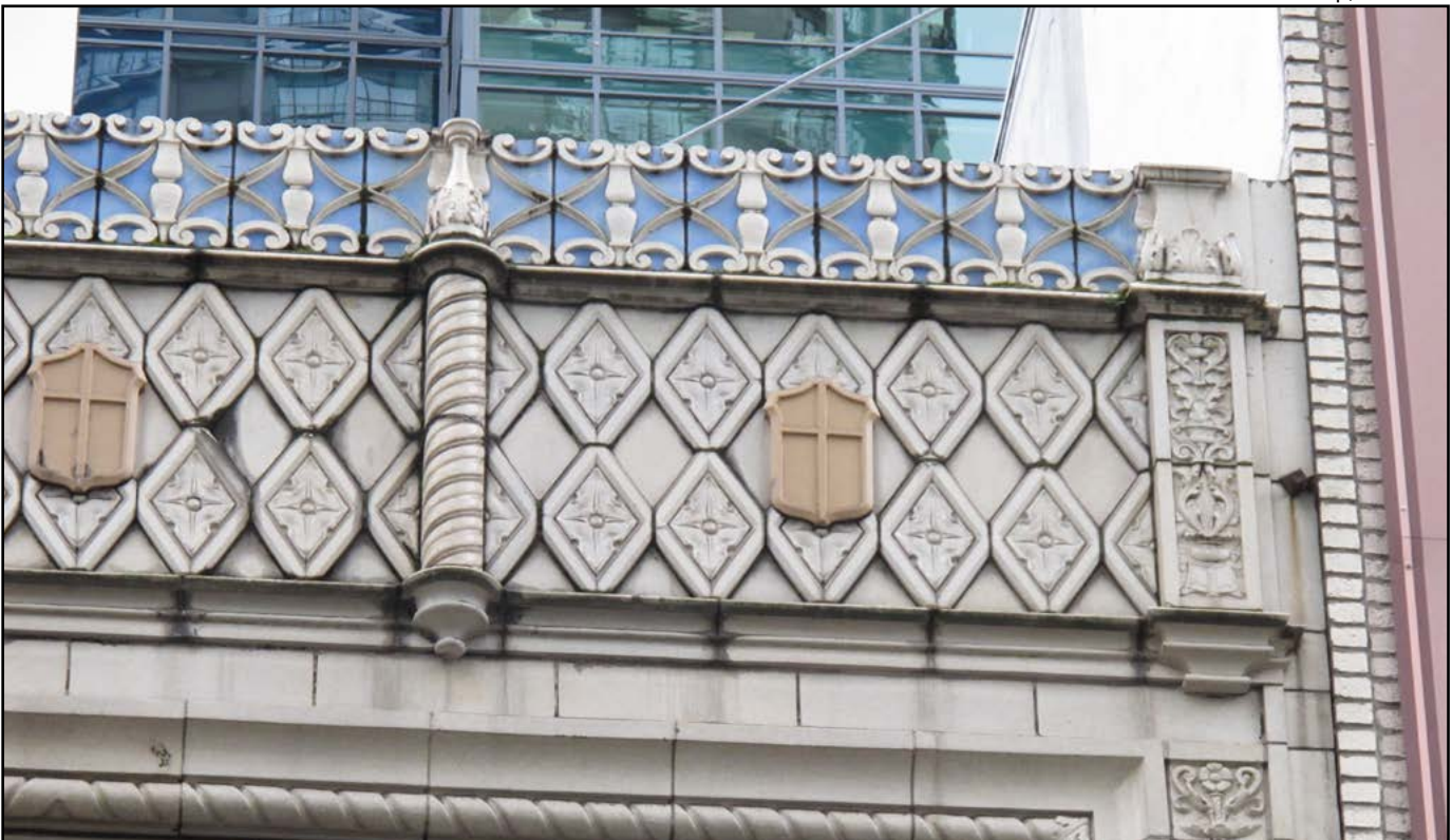
Figure 21 • Terra cotta cornice and parapet
