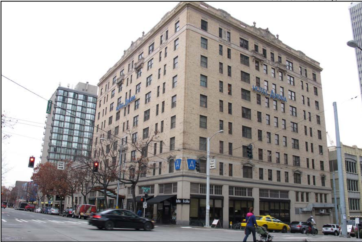
Figure 9 • View E, Hotel Andra (formerly Claremont), corner of Fourth Ave & Virginia Street
