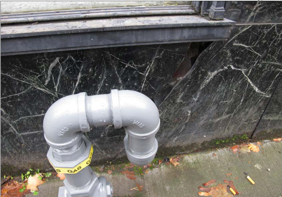
Figure 16 • Detail, black marble and gas line
