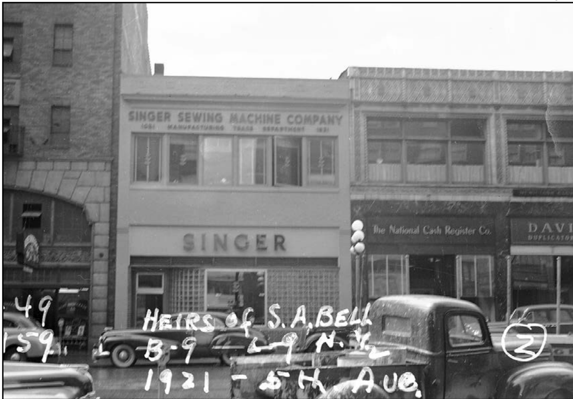
Figure 38 • National Cash Register Building, partial eastern façade, far right, 1949
