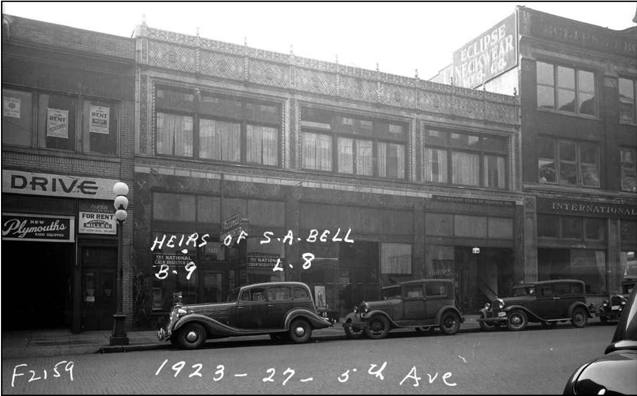
Figure 37 • National Cash Register Building, eastern façade, 1937
