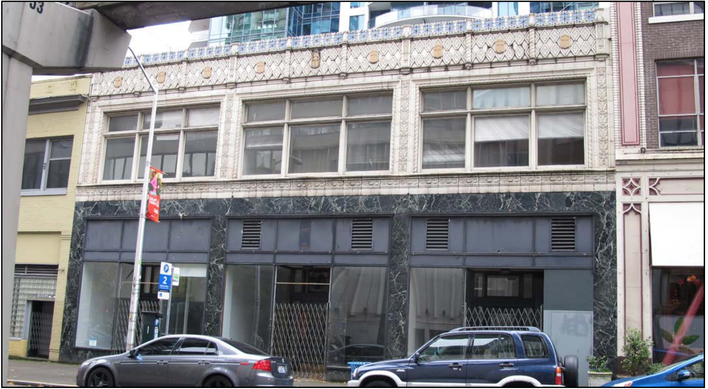
Figure 13 • National Cash Register Building, eastern façade, Fifth Avenue
