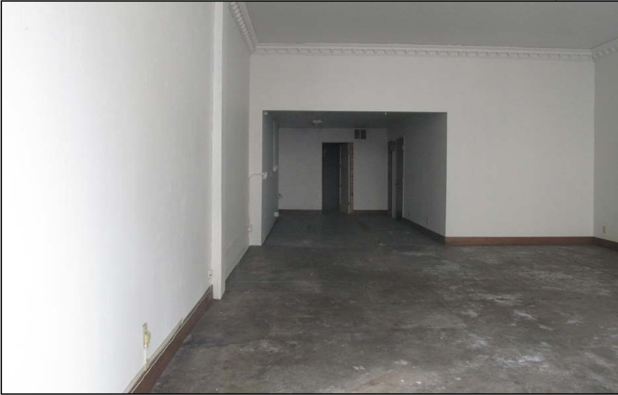
Figure 24 • First floor interior
