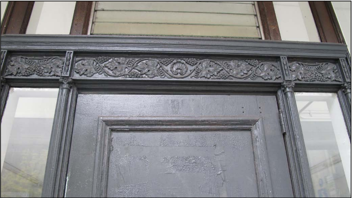
Figure 18 • Door lintel with molding
