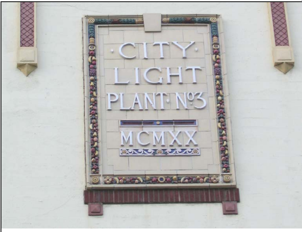
Figure 44 • Seattle City Light Plant No.3, detail of decorative terra cotta (Daniel Huntington, 1921)
