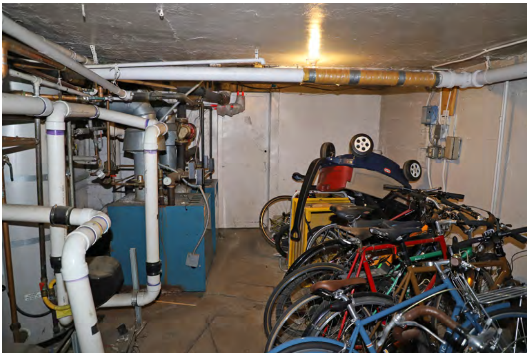
Figure 76. Basement, looking east.
