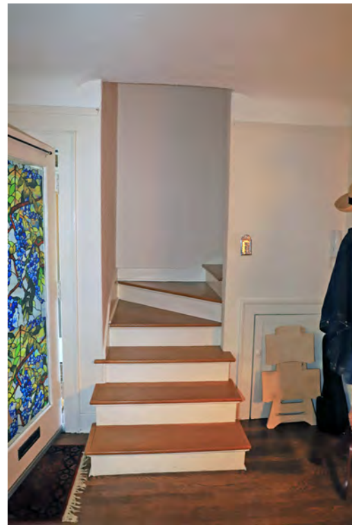
Figure 54. Stairway to second floor.
