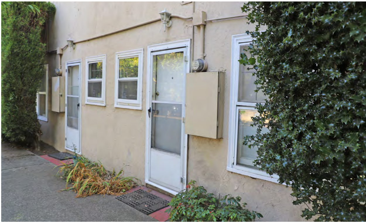
Figure 86. 17th Avenue E entrances, looking northeast.
