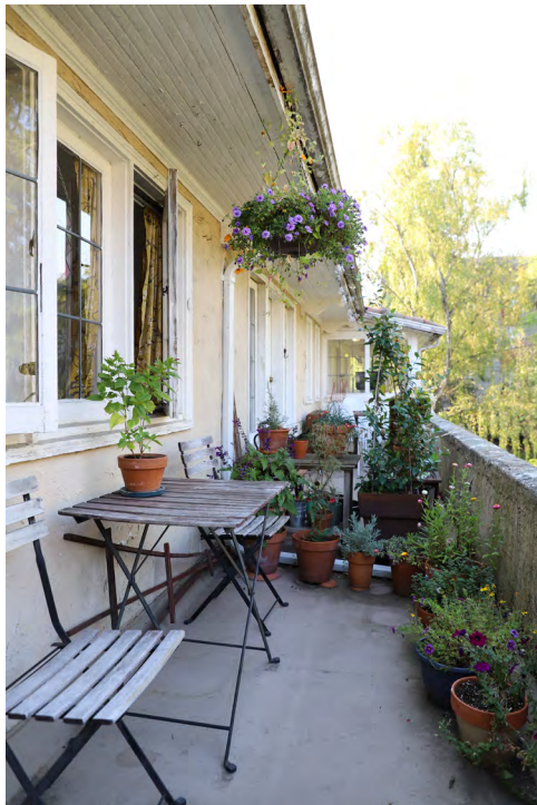
Figure 57. Second floor balcony, looking south.
