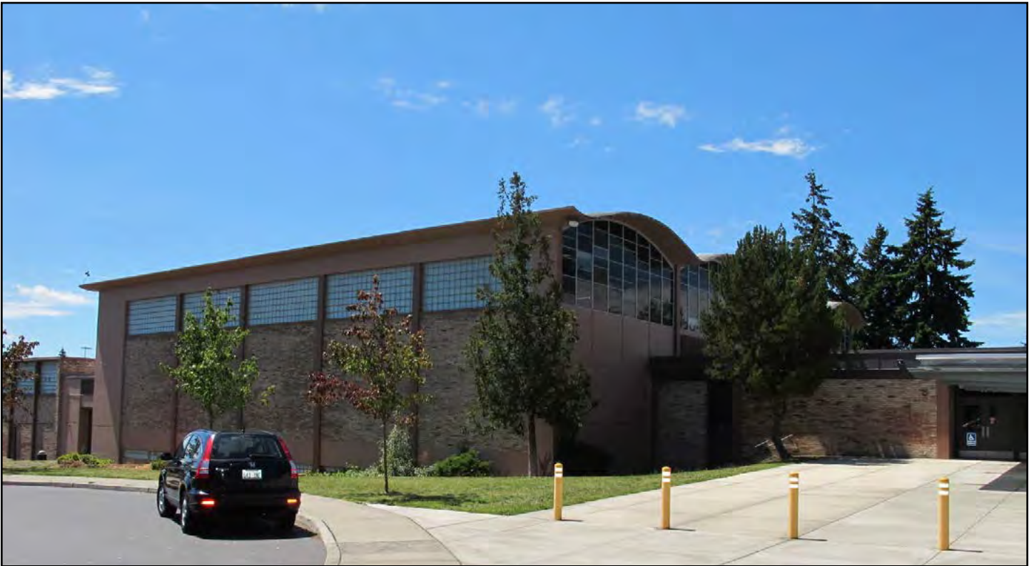
Figure 51. Ingraham High School, Gymnasium, eastern façade
