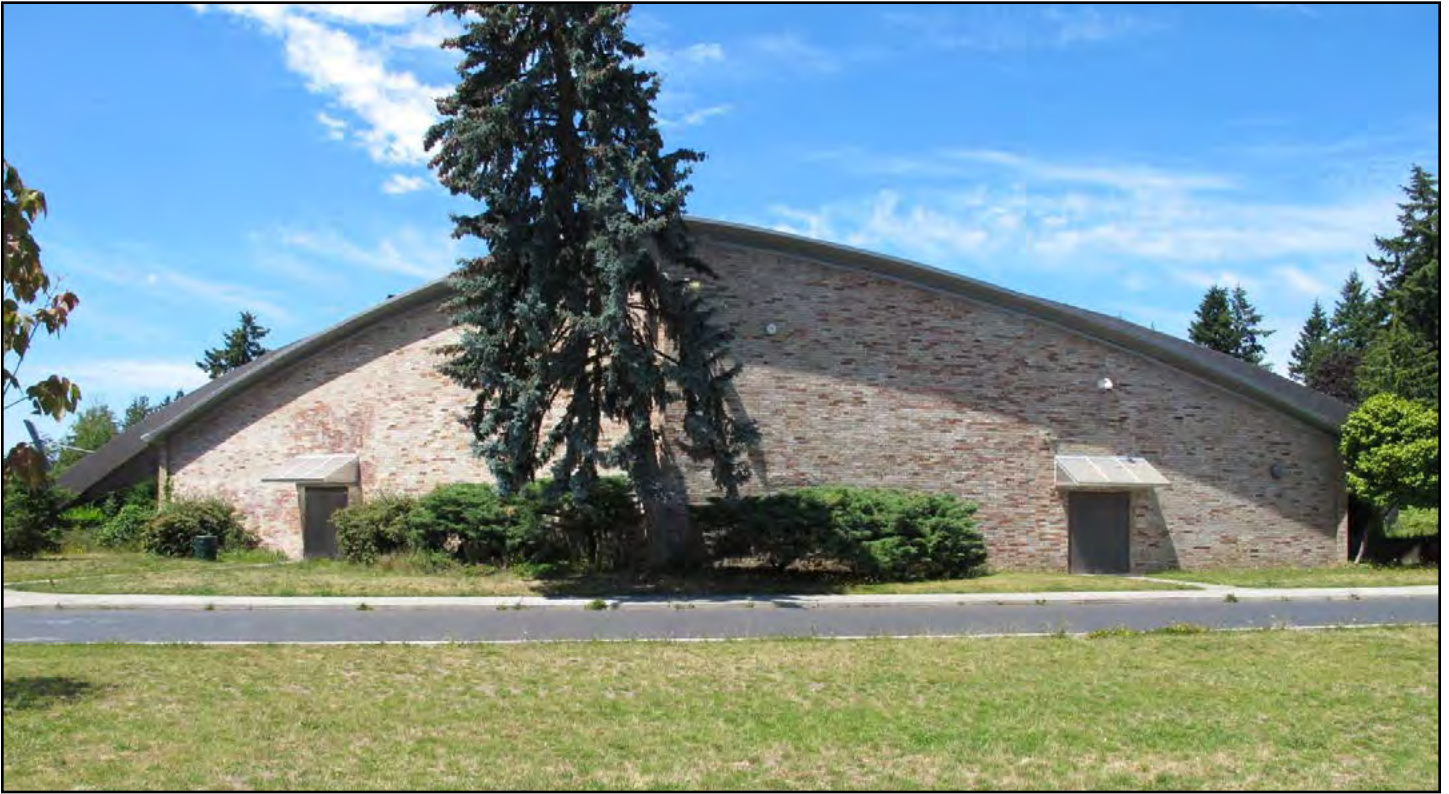
Figure 45. Ingraham High School, Auditorium, southeastern side
