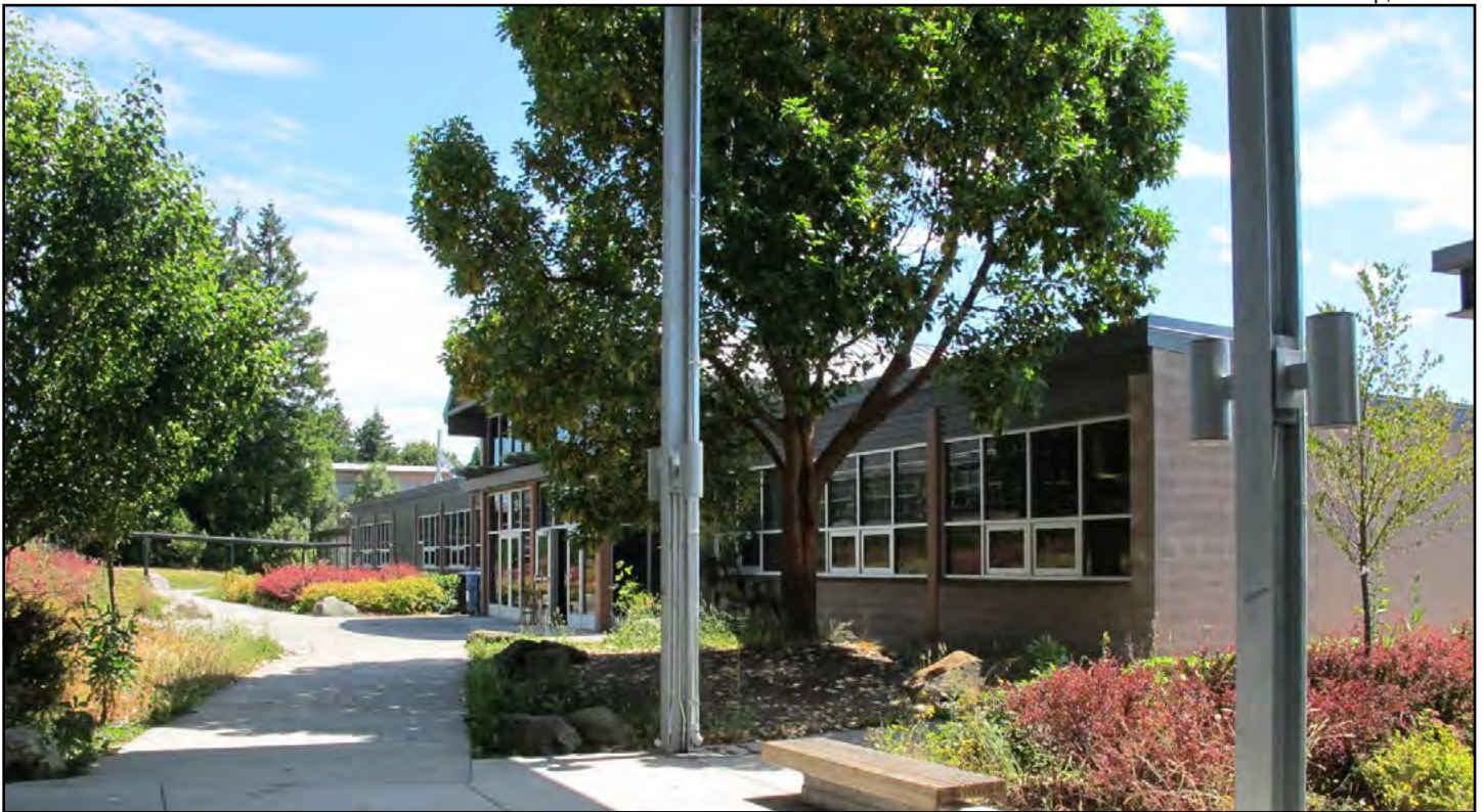
Figure 26. Ingraham High School, Building 200, northern façade
