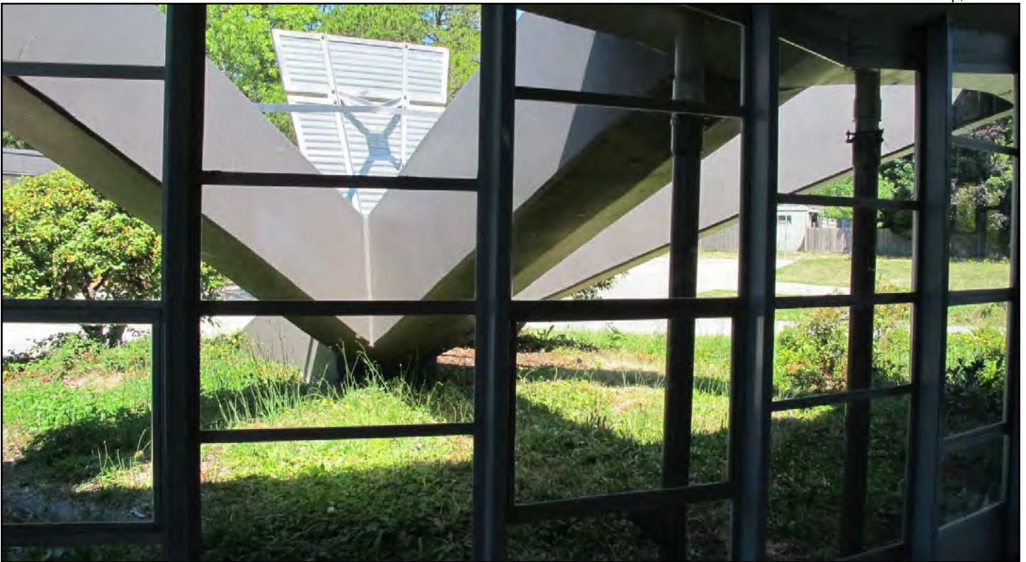
Figure 48. Ingraham High School, Auditorium vestibule viewing towards northwestern abutment
