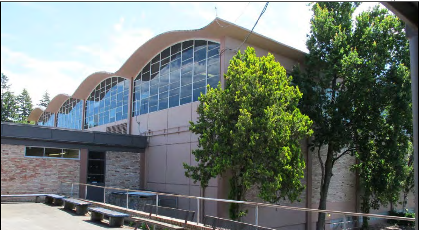
Figure 54. Ingraham High School, Gymnasium, partial northern and eastern façades
