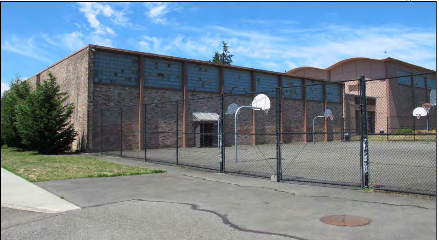
Figure 52. Ingraham High School, Gymnasium, eastern façade
