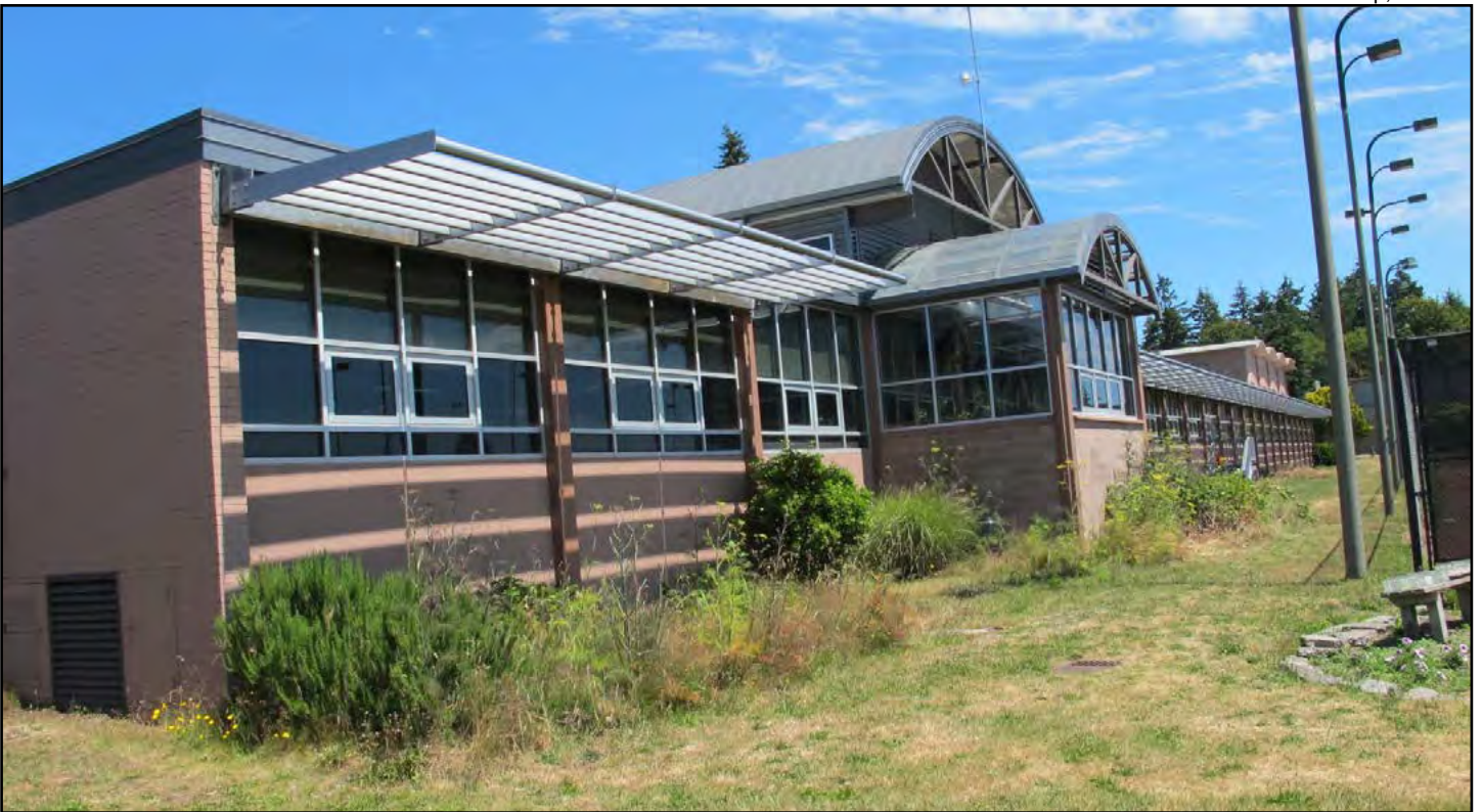
Figure 24. Ingraham High School, Building 200, southern façade
