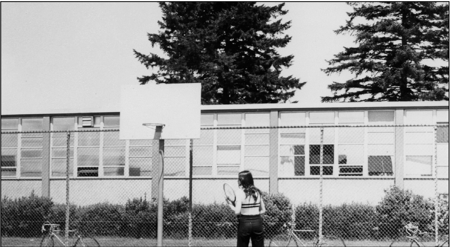
Figure 74. Ingraham High School, southern façade of building 200, viewing from tennis courts, 1960
