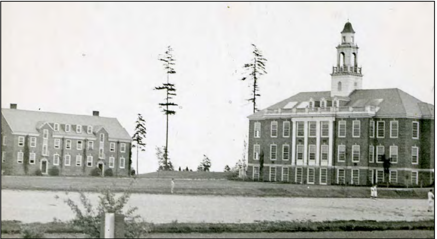
Figure 61. Bliss Hall, The Lakeside Boys' School (now Lakeside School), N 145th Street, 1930
