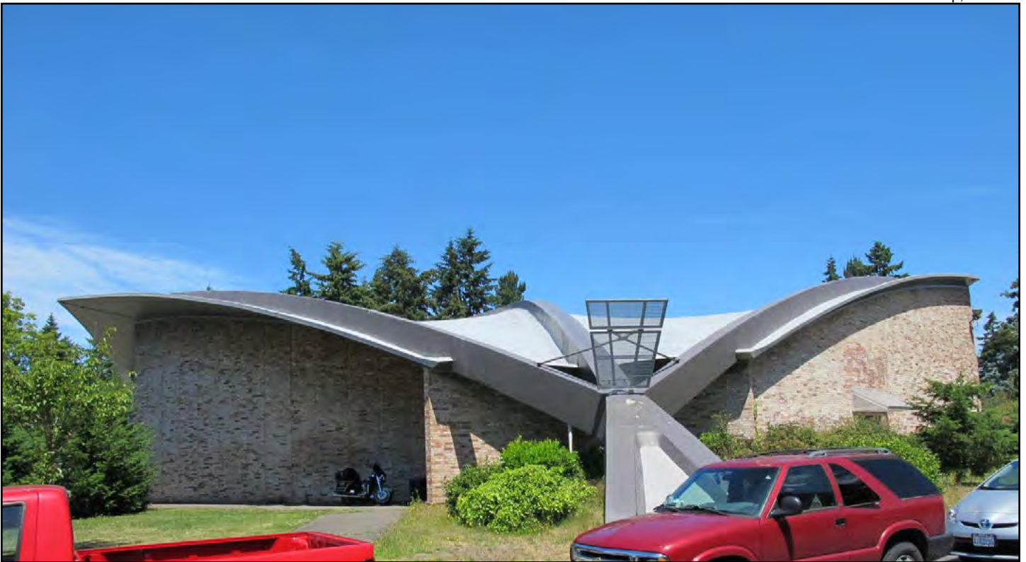
Figure 46. Ingraham High School, Auditorium, southern side
