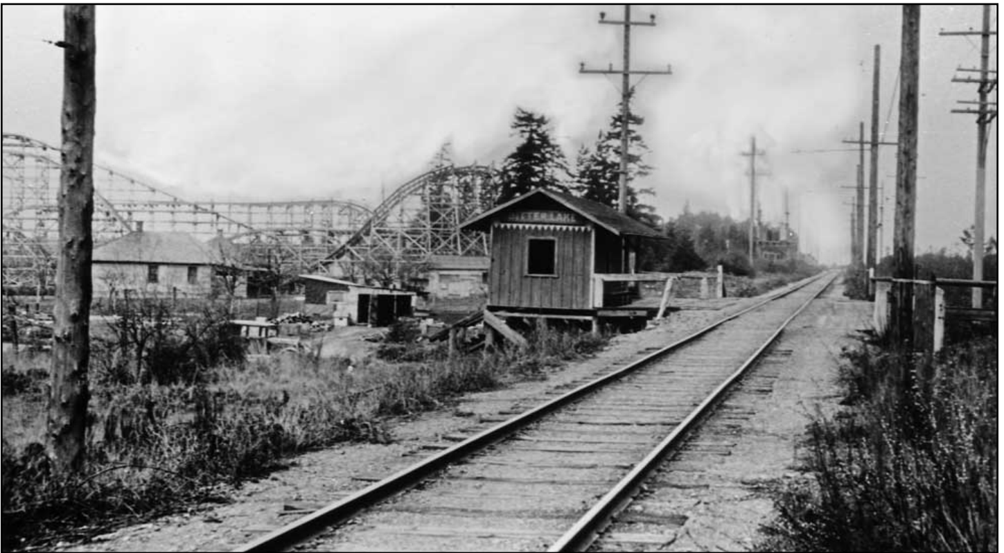
Figure 58. The Seattle-to-Everett Interurban Railway at Bitter Lake Station, ca. 1932
