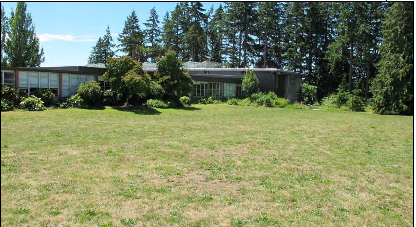
Figure 16. Ingraham High School, Main Building, northern façade
