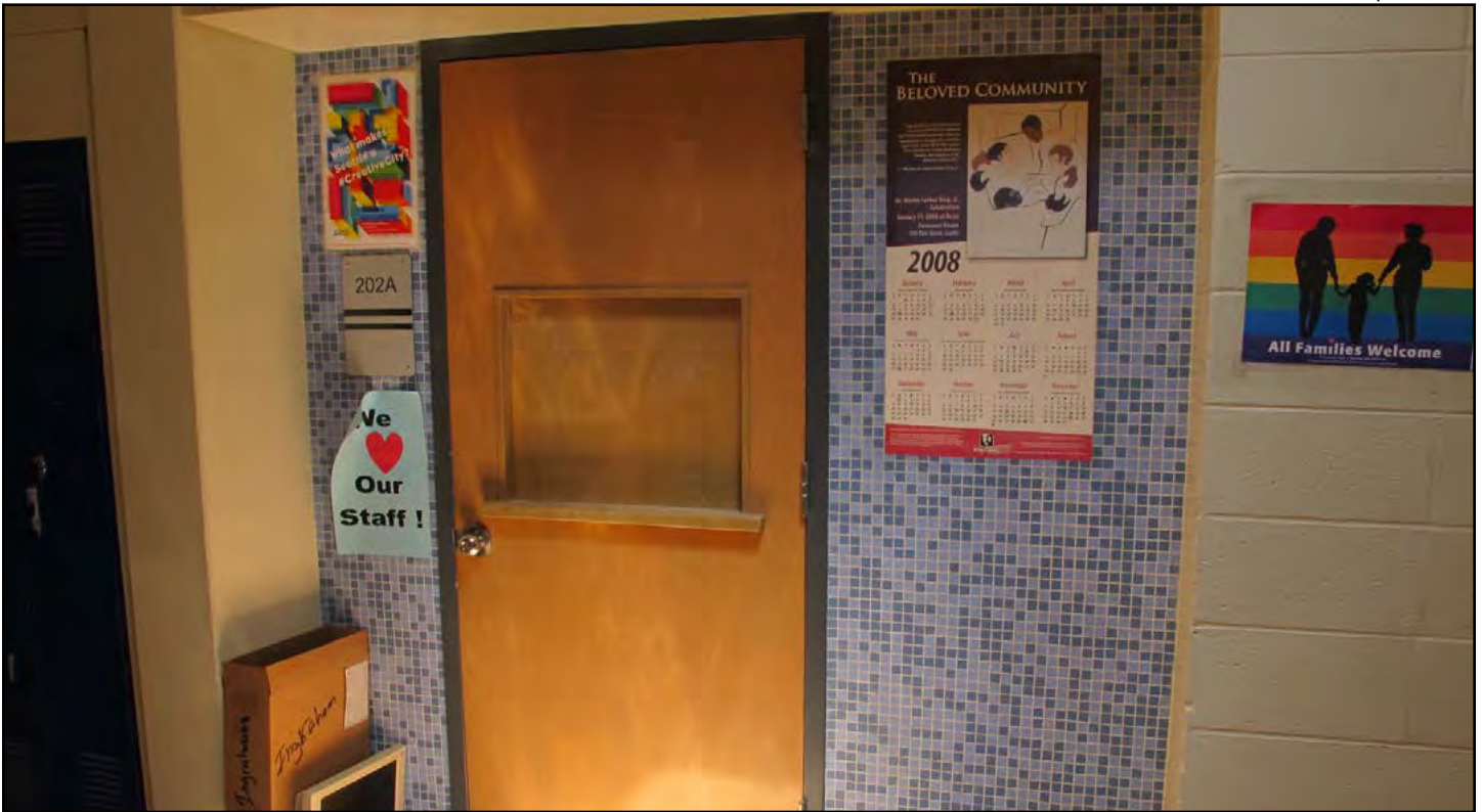
Figure 37. Ingraham High School, typical detail at hallway
