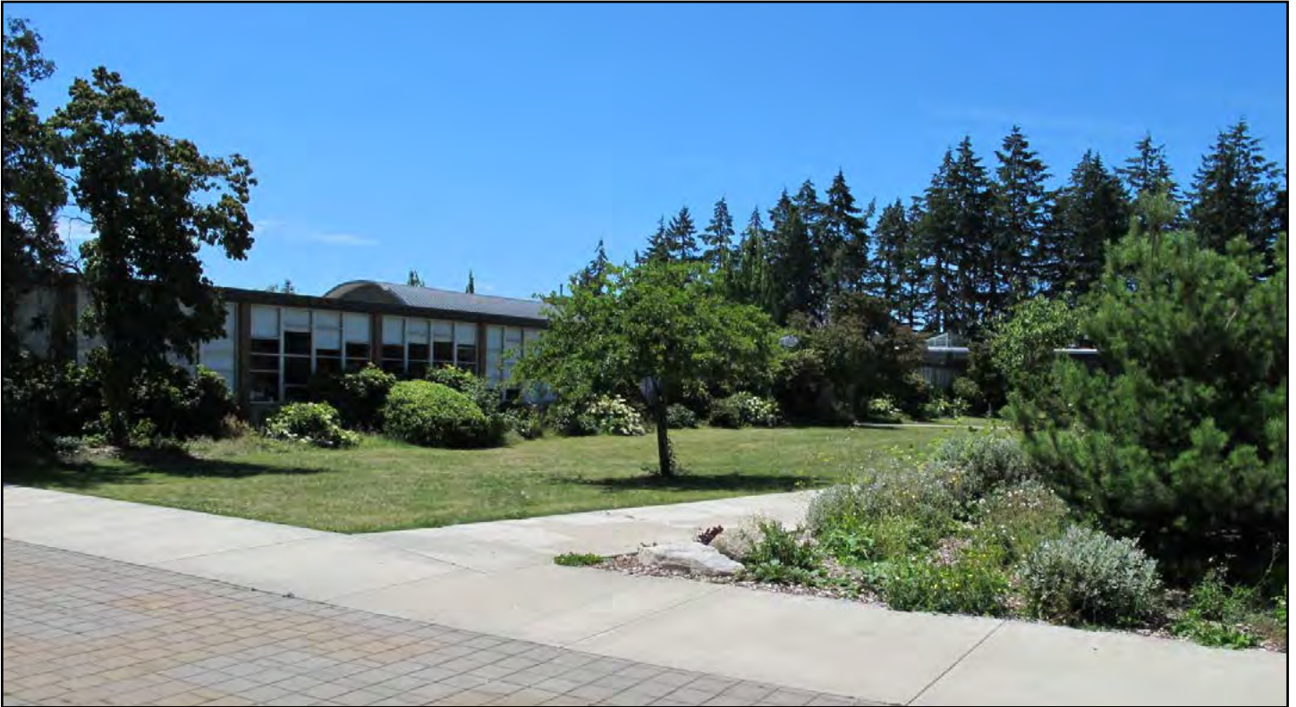
Figure 15. Ingraham High School, Main Building, northern façade
