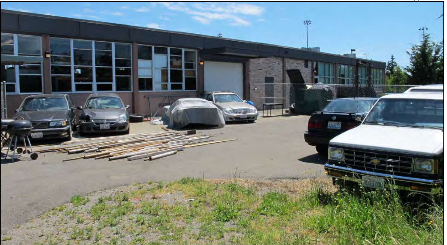
Figure 28. Ingraham High School, Building 300, western façade
