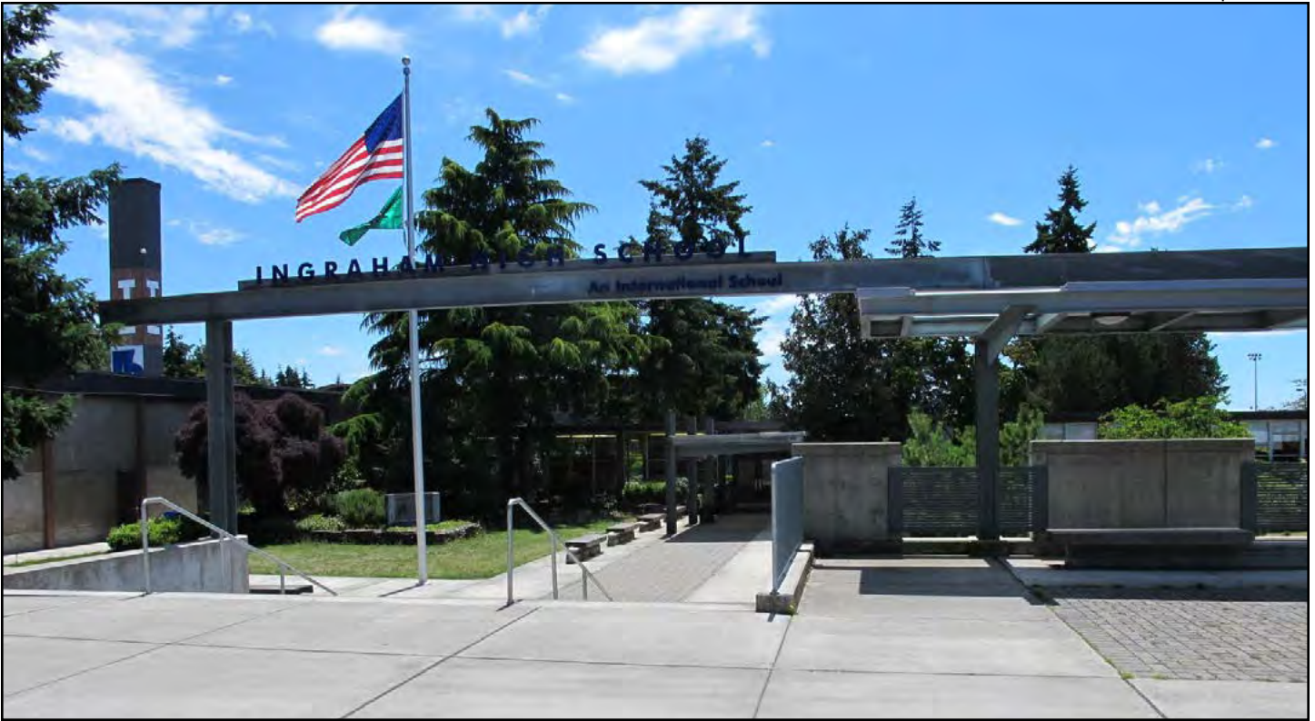
Figure 13. Ingraham High School, Main Building, entry
