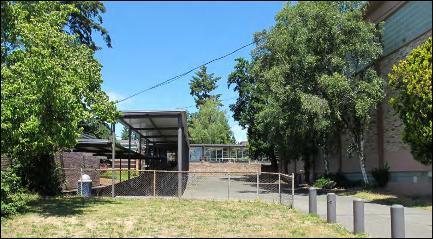
Figure 17. Ingraham High School, Main Building, southern façade/entry
