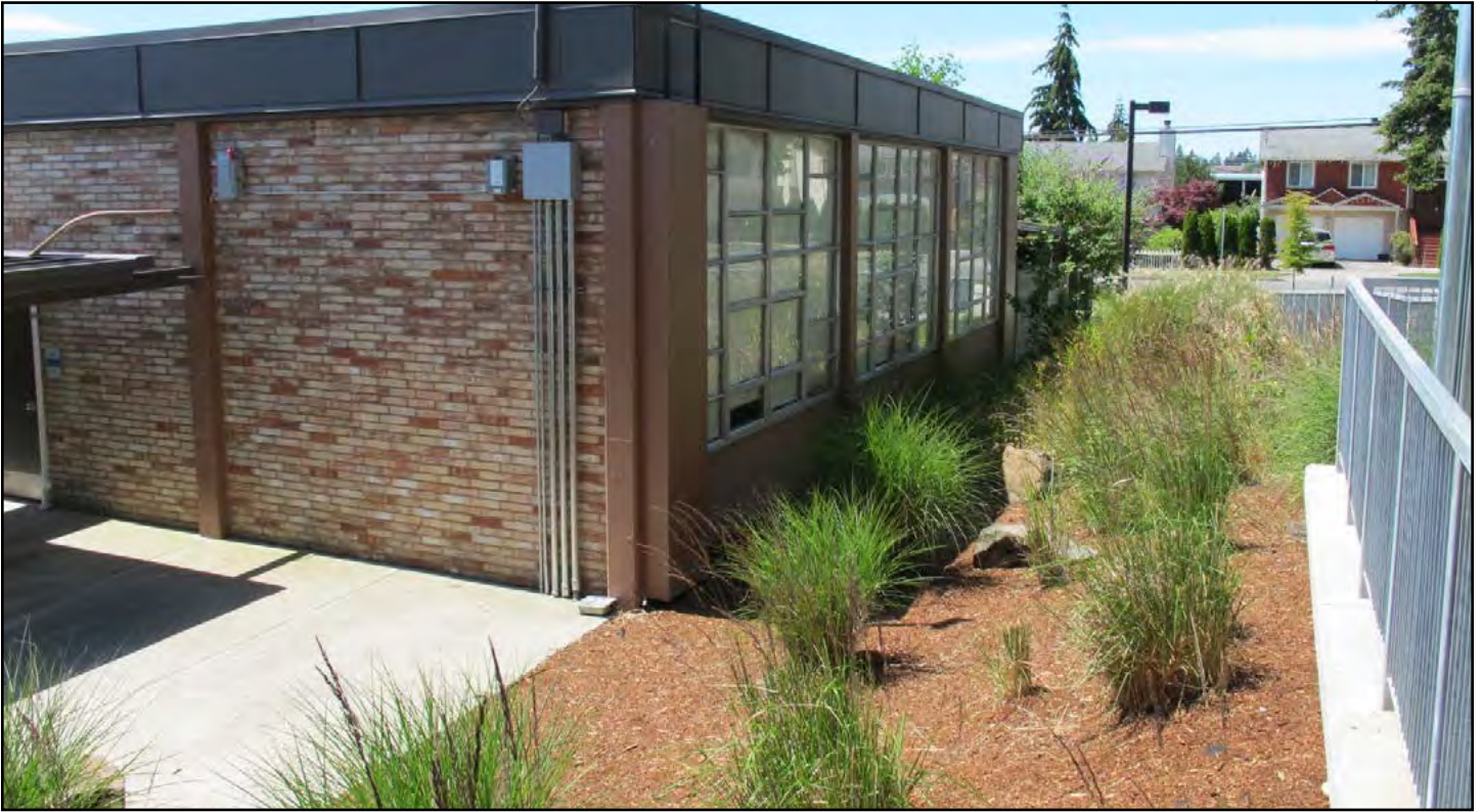
Figure 27. Ingraham High School, Building 300, northern façade
