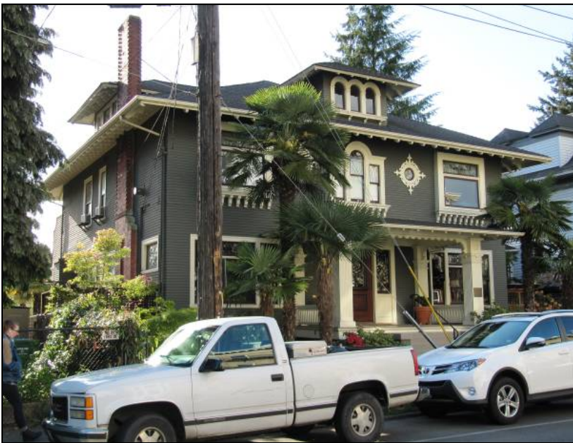
Figure 42. Below, looking northwest at the east and south facades.
