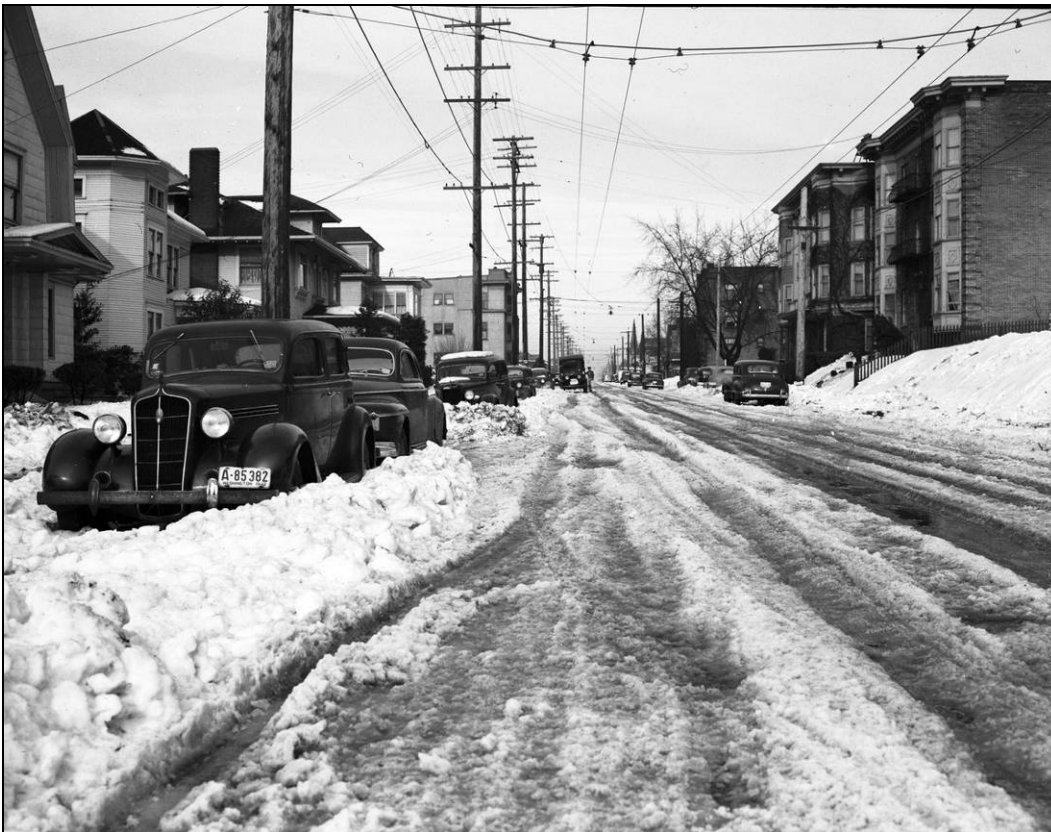
Figure 10. Below, a view looking north on 15 th Avenue E from E Olive Street on January 26, 1943. The Singerman residence is partially visible on the left in mid-frame, distinguished by its tall brick chimney (SMA 40083).
