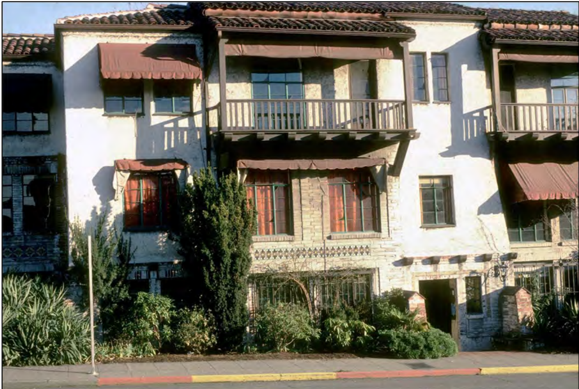
Fig. 55 – 1975 photo of the subject building, center part of west elevation. (SMA #180227)
