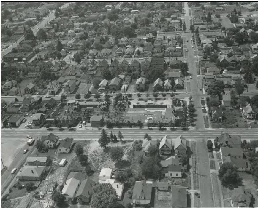
Figure 74. Below, another aerial view from 1975, showing residential development to the west and slightly north of the substation (center) and 23 rd Avenue in the lower half (SCL Collection).
