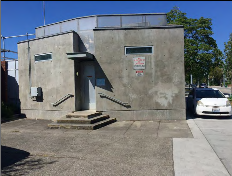
Figure 34. Above, detail view looking north at the main entry to the control building and the south facade of the addition. The element above the concrete facade is a perforated metal screen for rooftop equipment. 23 rd Avenue is to the right.
