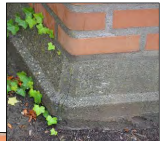
Figure 54. Below left and inset, detail views of the original masonry perimeter wall and typical cast-in-place base and footing with some curved brick (lower left photo, Rebecca Ossa, SCL October 2017). Lower right corner, a newer section of the 2003 masonry wall.
