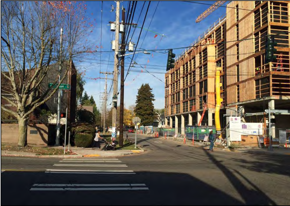
Figure 21. Above, context view looking north on 22 nd Avenue from the intersection of E Union Street, with a new mixed-use development under construction to the right, a 1956 church to the left, and EPS in the distance (center).
