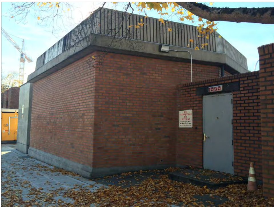
Figure 35. Below, detail view looking southwest at the north and east facades of the control building. Note the original corrugated patterned concrete roof “cap.”
