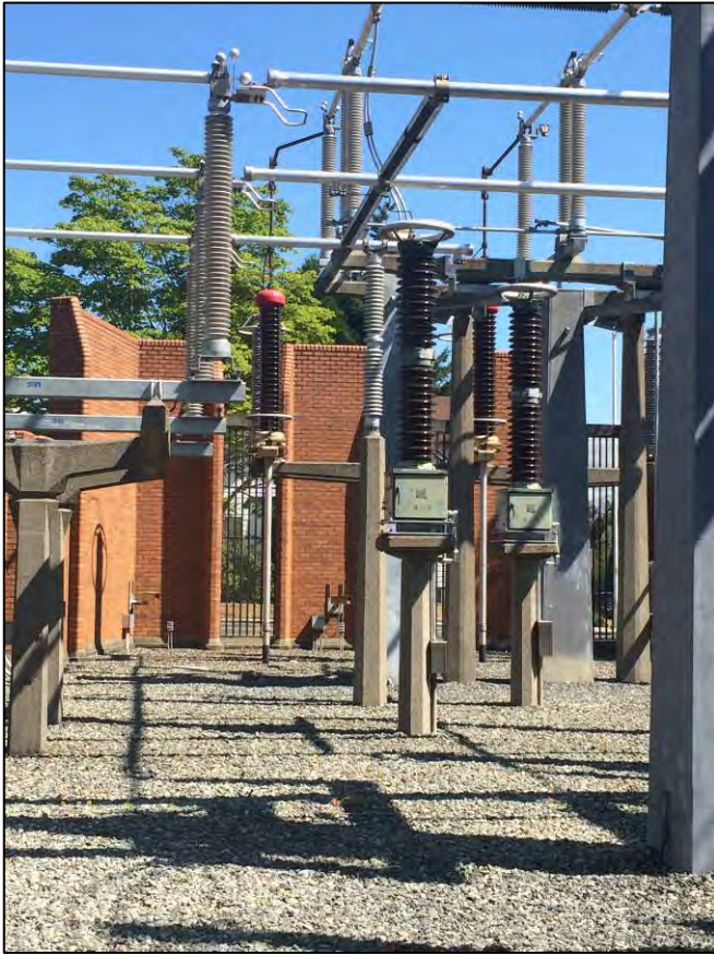
Figures 55 and 56. Above, detail views of some of the original pre-cast concrete equipment supports, and the northeast corner of the switchyard.
