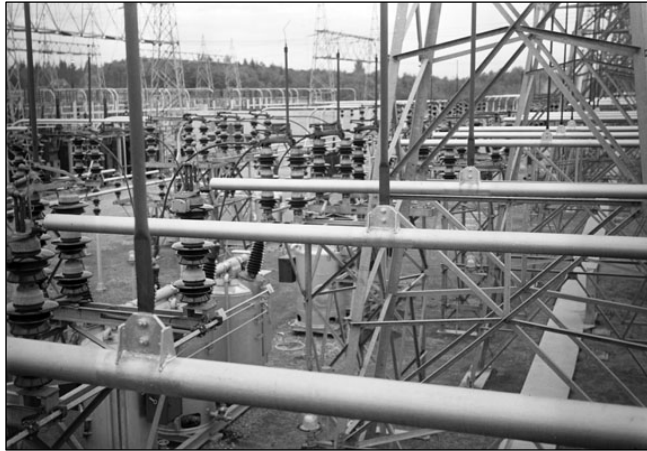
Figures 94 and 95. Photos of other substations illustrate the relative consistency in design as switchyard layouts became more based on manufactured components than customized or shop-built equipment. Above left, the bus fork at the Bothell Substation, 1964 (SMA 168190). Above right, larger lattice type supports at the Duwamish Substation, 1955 (SMA 172931).
