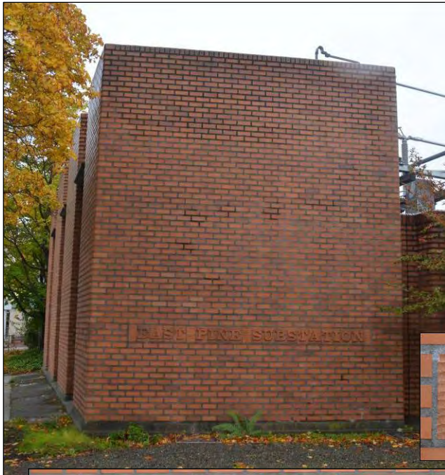
Figure 28. Left, looking south at the north facade of the high yard wall section near the control building, which contains the name of the substation in sculpted brick letters. 23 rd Avenue is to the left off camera (Rebecca Ossa, SCL, October 2017).
