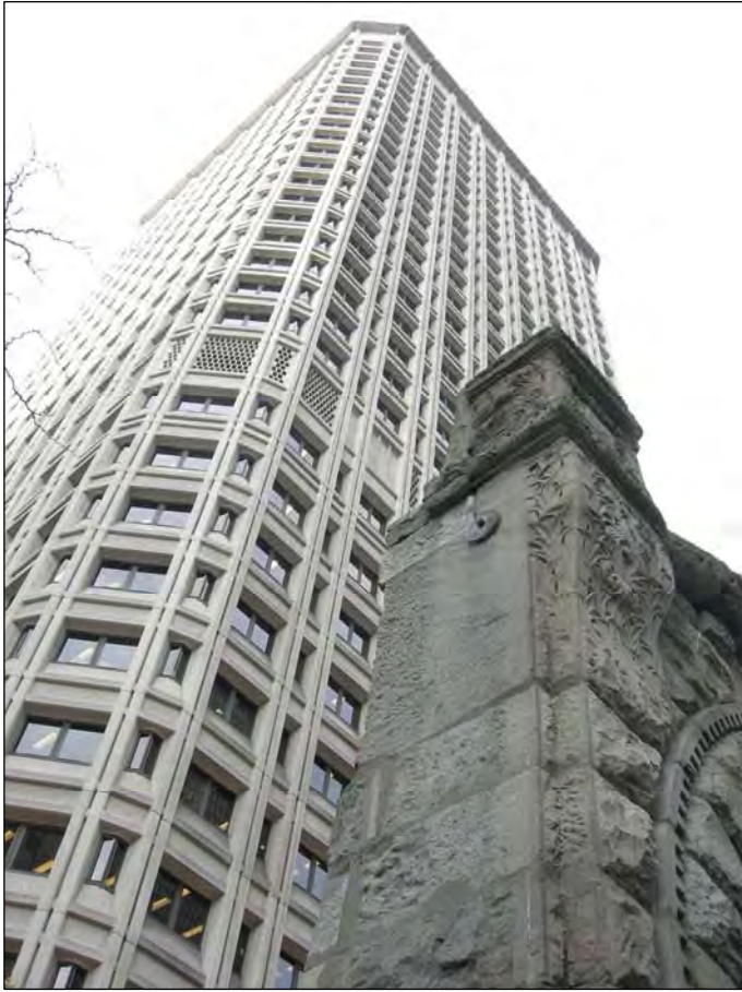
Figure 85. ABOVE, the 37-story reinforced concrete Henry M. Jackson Federal Office Building at 915 2 nd Avenue, Seattle, 1964-1971 (Joe Mabel, Wikimedia).
