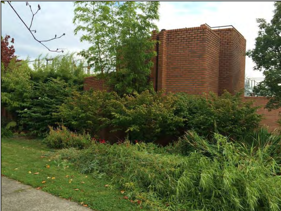
Figure 114. Left, a view looking generally south at the outer walls of the children's viewing tower on November 26, 2001. By this date, new landscaping had been planted around its base to obscure the former steps (SCL Collection).
