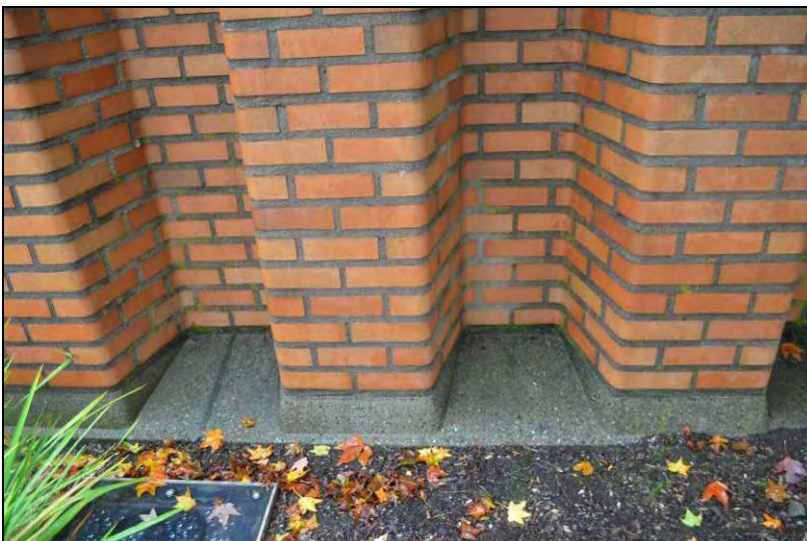
Figure 54. Below left and inset, detail views of the original masonry perimeter wall and typical cast-in-place base and footing with some curved brick (lower left photo, Rebecca Ossa, SCL October 2017). Lower right corner, a newer section of the 2003 masonry wall.
