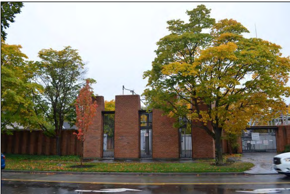
Figure 24. Below, Frontal view of the high yard wall along 23 rd Avenue perimeter. Note the grilles between the wall sections, designed for viewing into the substation switchyard (Rebecca Ossa, SCL, October 2017).
