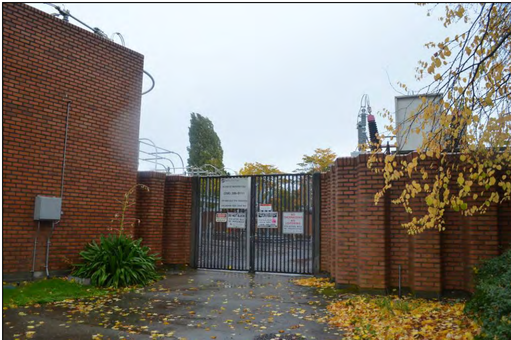
Figures 46 and 47. Above and below, detail views of two of the four vehicle gates in the west wall showing details of concrete posts and adjacent wall conditions. (See figure 106 for comparable original view to the photo below.)
