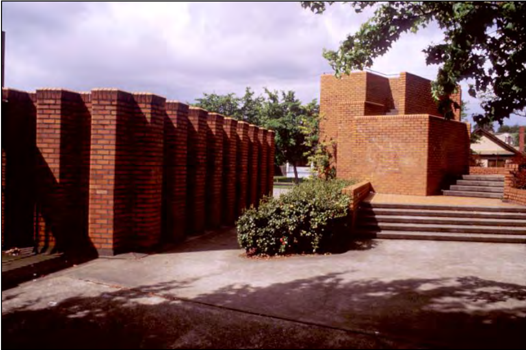
Figure 104. Above, looking west at the children’s viewing tower after completion, taken in 1969 (SMA 123758).
