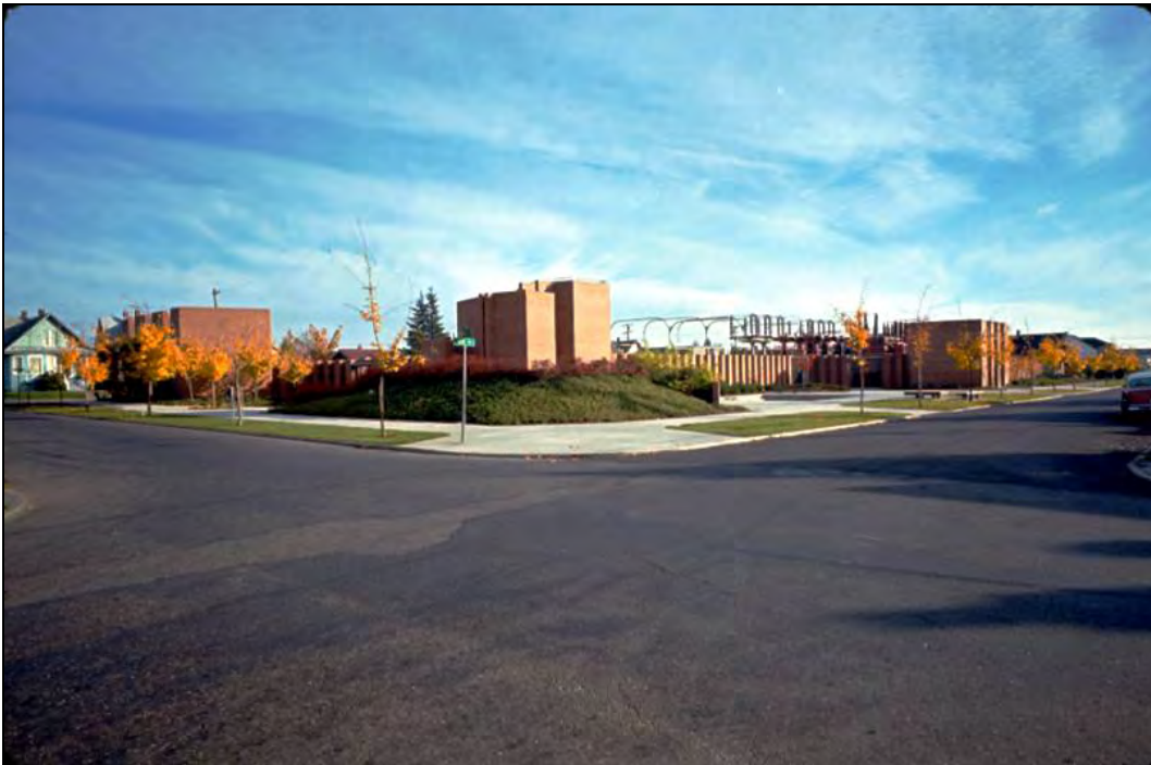
Figure 105. Below, looking southeast at the substation after completion, taken in 1969 (SMA 123757).
