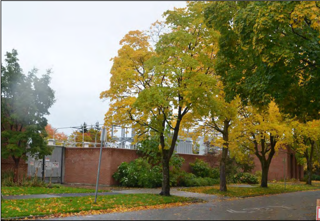
Figure 44. Above, looking southeast toward the west perimeter contemporary brick wall. The tower is to the left, and the high yard wall is to the right, behind the mature trees.
