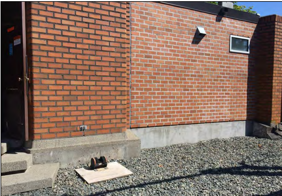
Figure 63. Below, detail view of the original west facade, left, and the later addition, right. Note the lighter brick and mortar differences.
