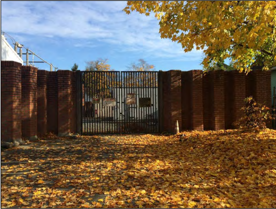
Figure 50. Above, looking east at corrugated walls and fourth set of vehicle entry gates near the south end of the west wall.
