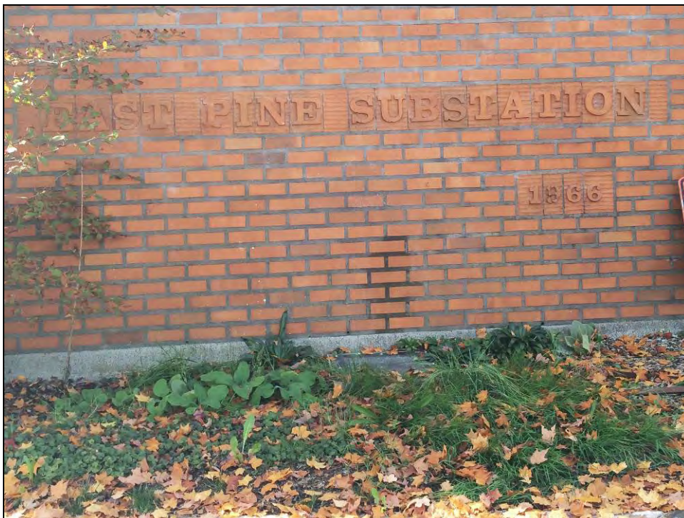
Figure 39. Below, detail view of the signature brick on the northeast high yard wall noting the facility's name and year of design/construction.
