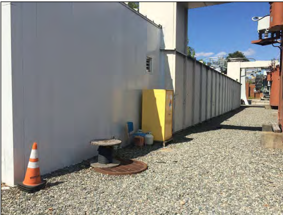
Figure 59. Below, looking northwest at a recently installed steel clad workshop and covered switchgear equipment, located along the southern portion of the west wall, parallel to 22 nd Avenue (out of frame to the left).
