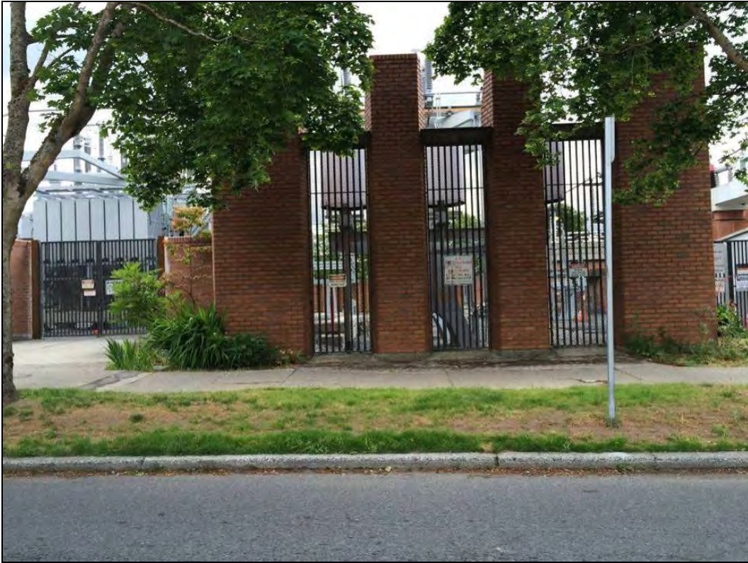
Figure 48. Above, additional view looking east at the west perimeter high yard wall. Note the slender pylons in the center.
