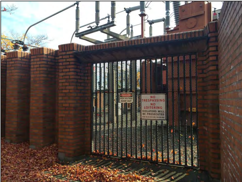
Figure 41. Below, looking south through a square viewing grille in the set-back section of the north perimeter wall. Contemporary brick wall to the right.
