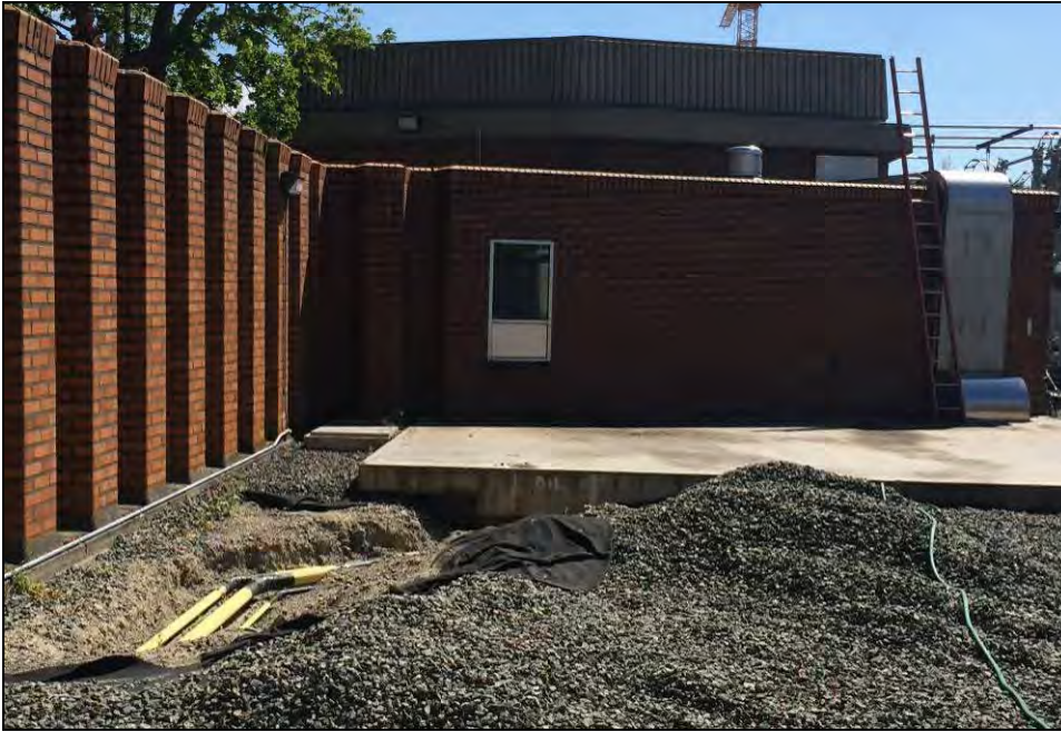
Figure 64. Above, looking south at the original north facade of with a newer single window. The slab in the foreground is part of a basement addition, dating from 2011.
