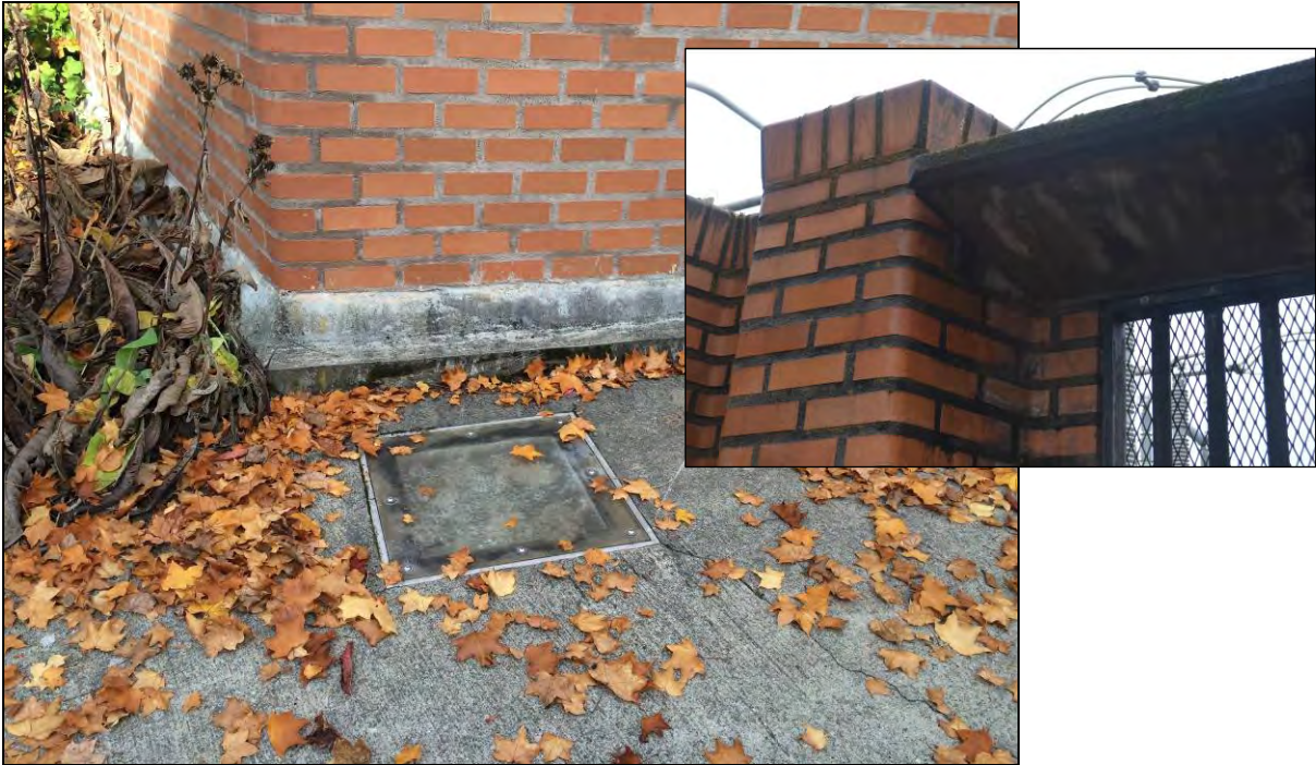
Figures 52 and 53. Above right and left, detail views of the original masonry wall sections, with straight and curved pieces, and precise precast concrete lintels and base sections, constructed above the cast-in-place concrete footings. These photos also show a portion of a newer exterior light fixture, set flush into the grade, which provides dramatic up-lighting on the brick walls.
