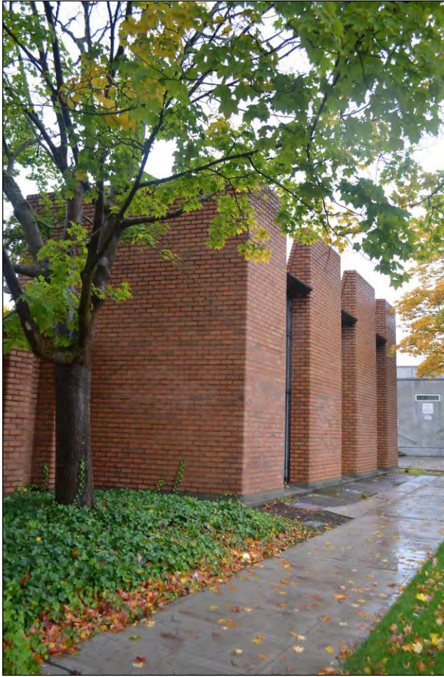
Figure 23. Left, view toward the high yard wall section, unaltered, along 23 rd Avenue. This section is nearest the substation's southeast corner. The control building is located to the center (left in the background) (Rebecca Ossa, SCL, October 2017).
