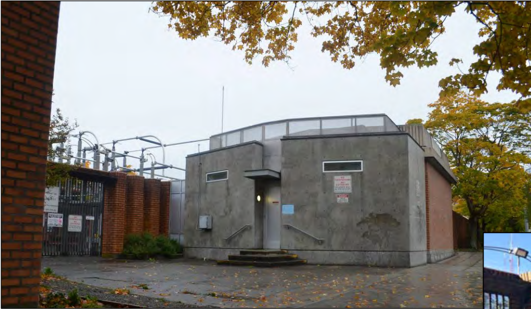
Figures 31 and 32. Above, looking northwest at the ca. 2003 south facade of the control building expansion. Right, detail view of the link between it and the original corrugated wall.
