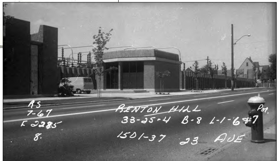
Figure 115 and 116. The 1966 Assessor's record card, above. Right, the property record card photo depicts a view looking northwest on 23 rd Avenue at the original south and east facades of the control building (King County Assessor's property record card photo, July, 1967).
