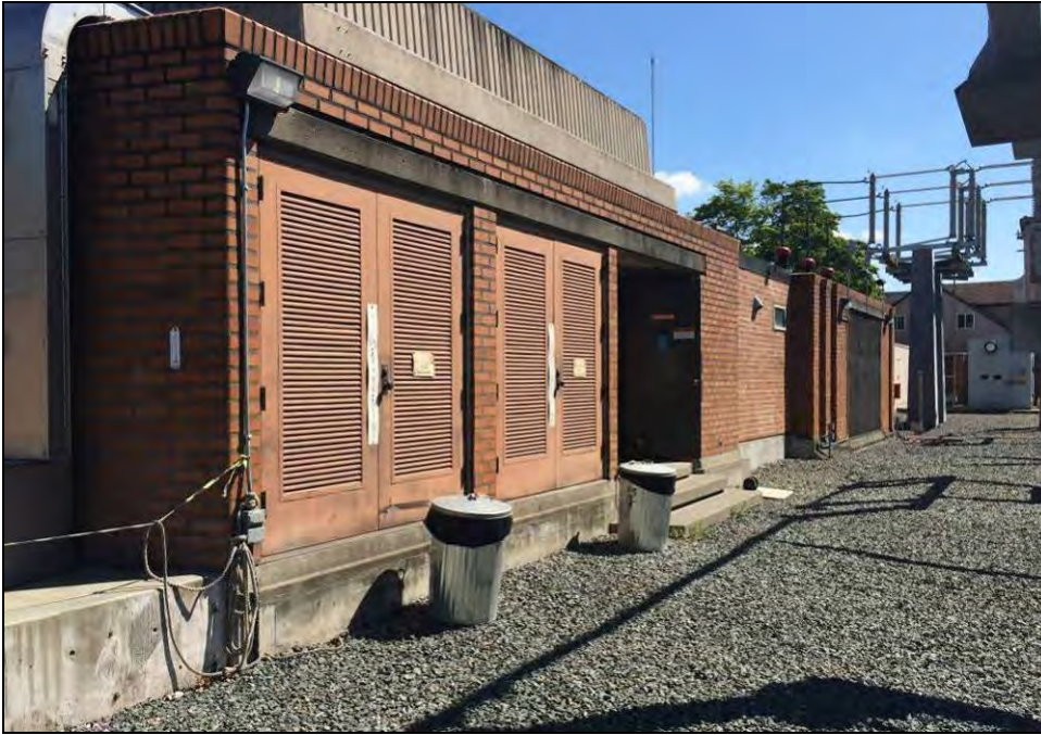
Figure 62. Above, oblique view looking southeast at the west facade of the control building. The metal louvered doors access a transformer room; the entry doors are adjacent and recessed. Note the original cast control roof cap.
