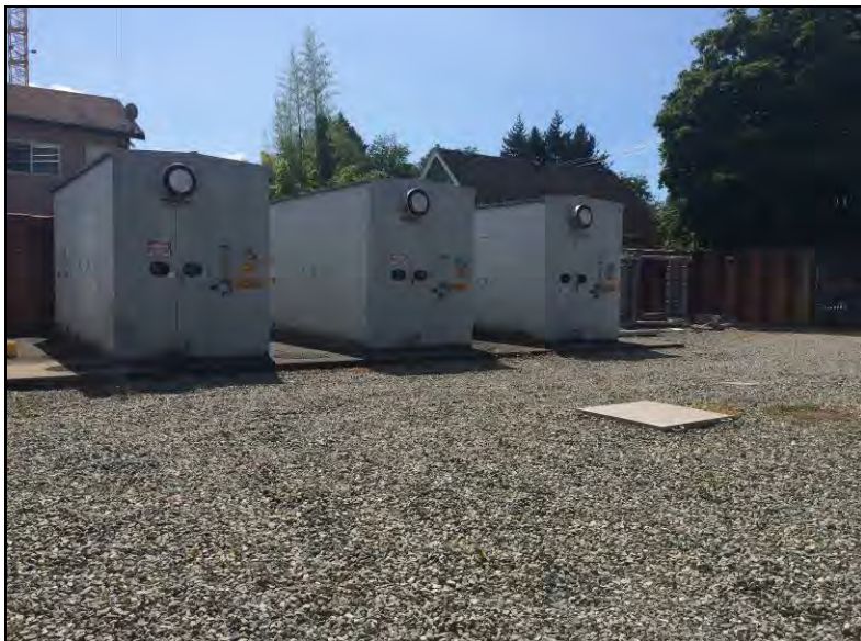
Figure 57. Below, typical equipment on concrete pads in the southern, lower section of the switchyard.
