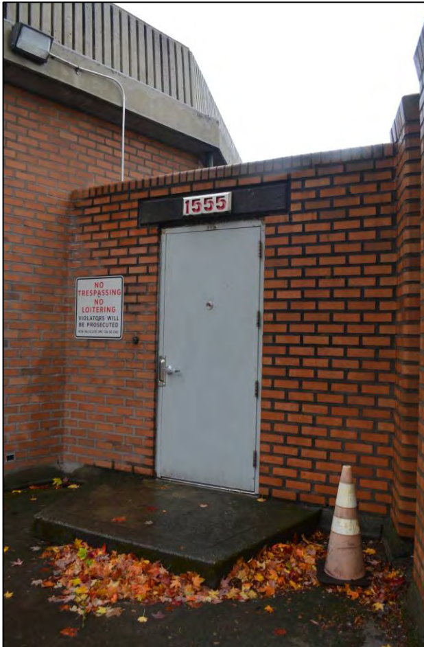
Figure 36. Left, detail view of the original entry, currently a secondary entry at the north end, east facade of the control building (Rebecca Ossa, SCL, October 2017).
