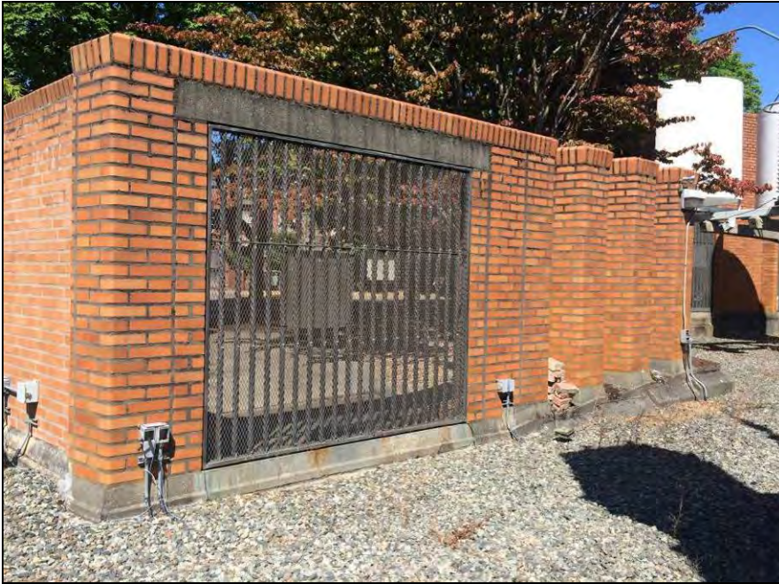
Figure 60. Above, looking northeast from within the switchyard at the square viewing grille with concrete lintel and custom cast brick soldier course cap. The viewing grilles are distinguished from the vehicle gates by the continuous pre-cast bases visible in this interior view.
