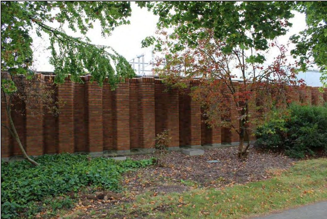
Figure 49. Below, looking east at the west perimeter corrugated wall (22 nd Avenue is behind the photographer).
