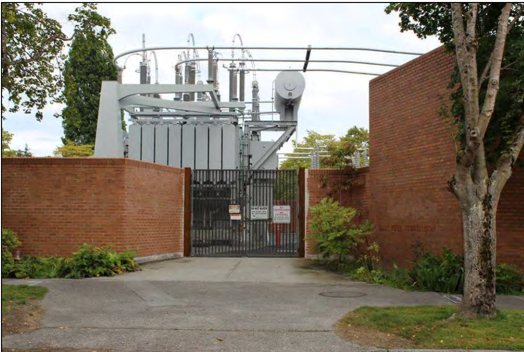
Figure 45. Below, looking east at a second vehicle entry gate (from the north) along 22 nd Avenue and adjoining the high yard wall to the right.
