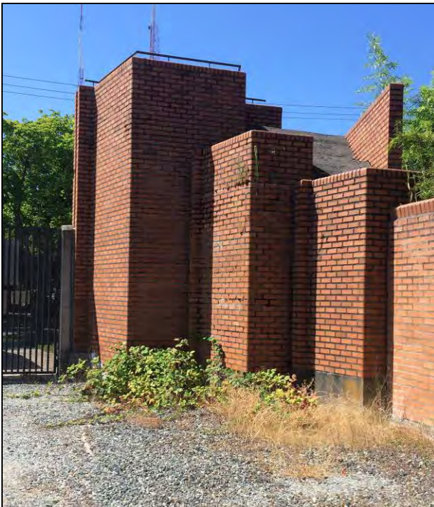
Figure 61. Below, looking northwest at the former viewing tower from within the switchyard showing the original northeast corner of this element. A portion of the vehicle gate in the west wall is visible on the left.
