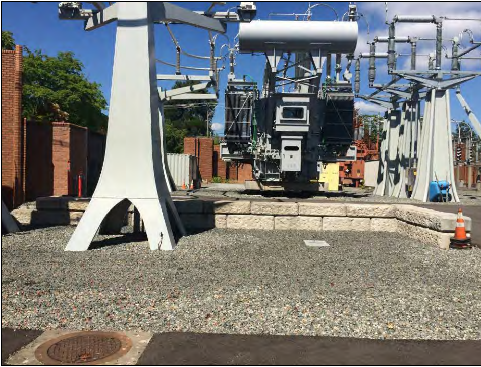
Figure 58. Above, looking north at the newer installed steel equipment supports, concrete block retaining wall in the middle of the switchyard and gravel groundcover.
