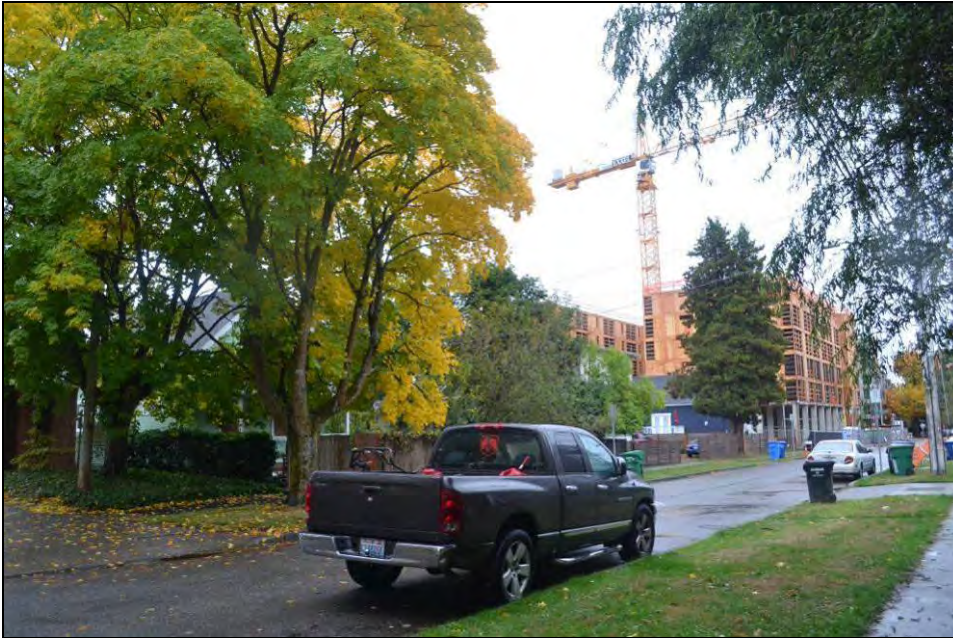
Figure 15. Above, looking southeast from mid-block on 22 nd Avenue with southwest corner of the EPS to the extreme left. A new mixed-use development at the corner of 23 rd Avenue and Union Street is in the background (Rebecca Ossa, SCL, October 2017).
