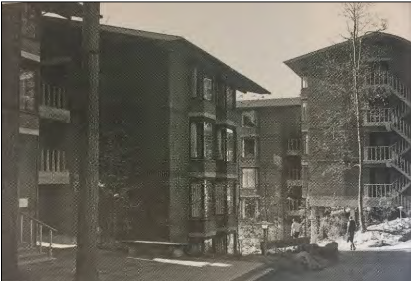
Figure 82. Below, Phase 2 of the Ridgeway Dormitories at Western Washington University in Bellingham, built 1963-1970 (Ochsner, p. 336). These buildings featured heavy timber, concrete slabs, and wood and brick cladding.
