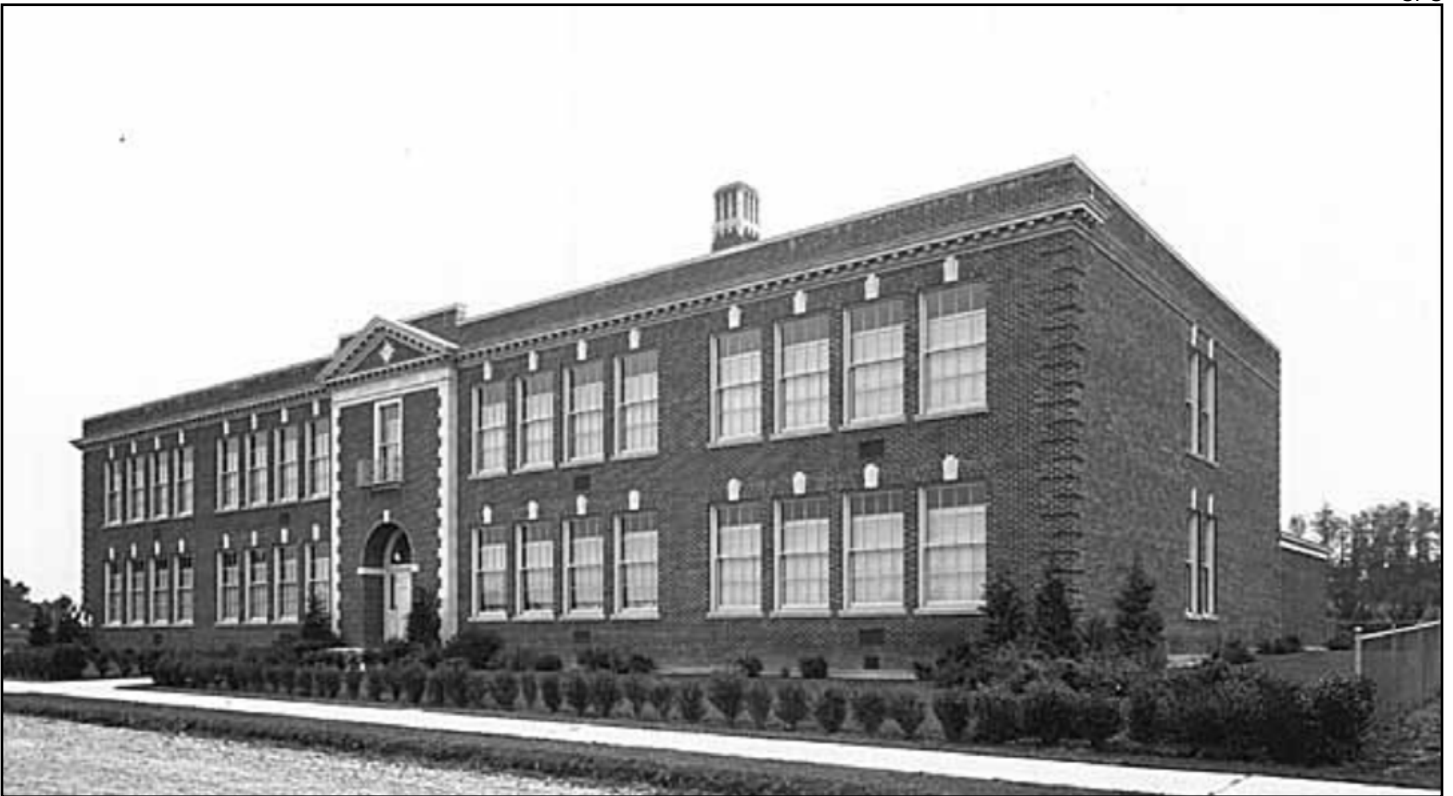
Figure 69. Laurelhurst School, 4530 46th Avenue NE (1928, Floyd A. Naramore, altered)
