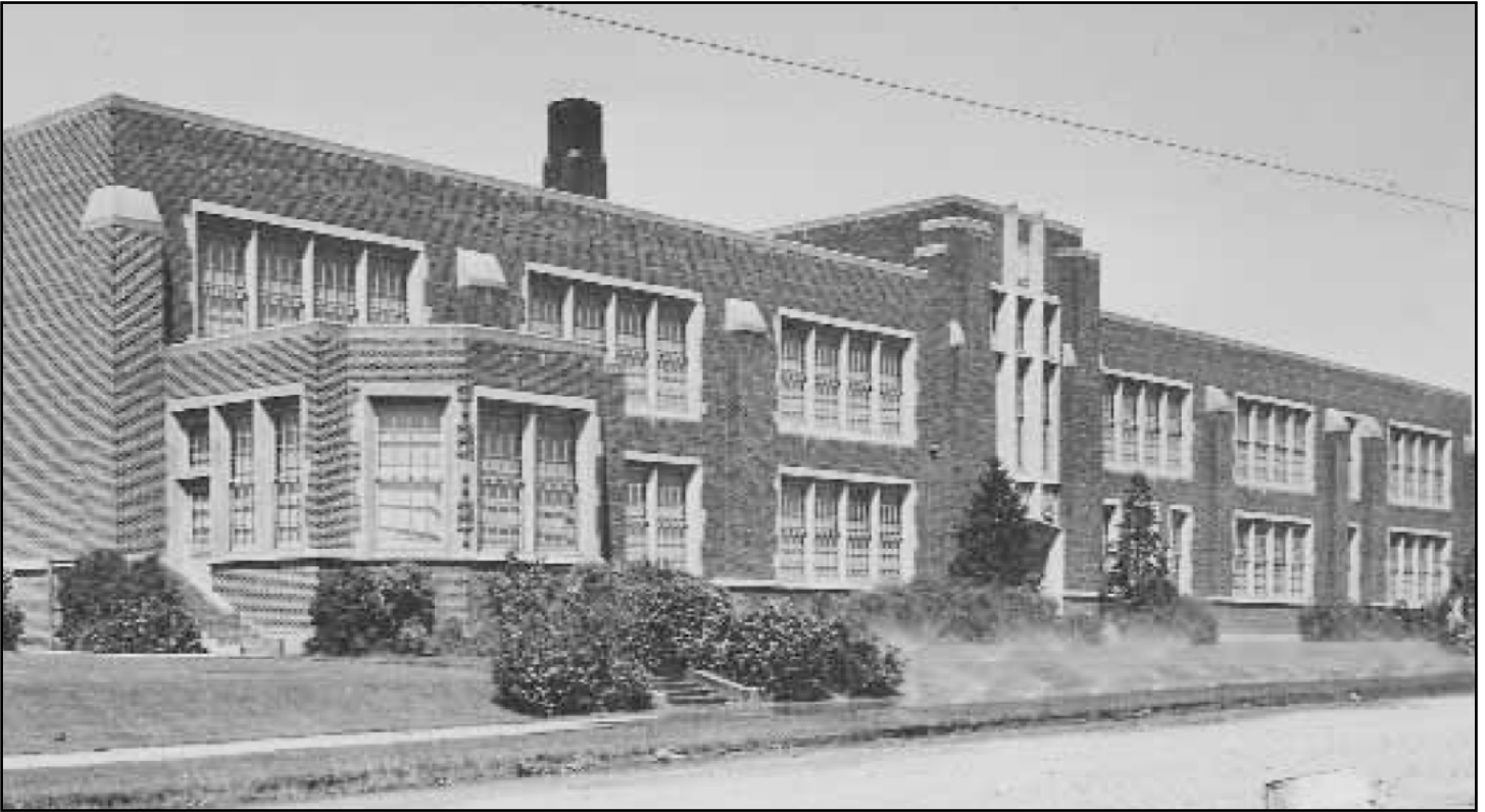
Figure 70. Daniel Bagley School, 7821 Stone Avenue N (1930, Floyd A. Naramore)
