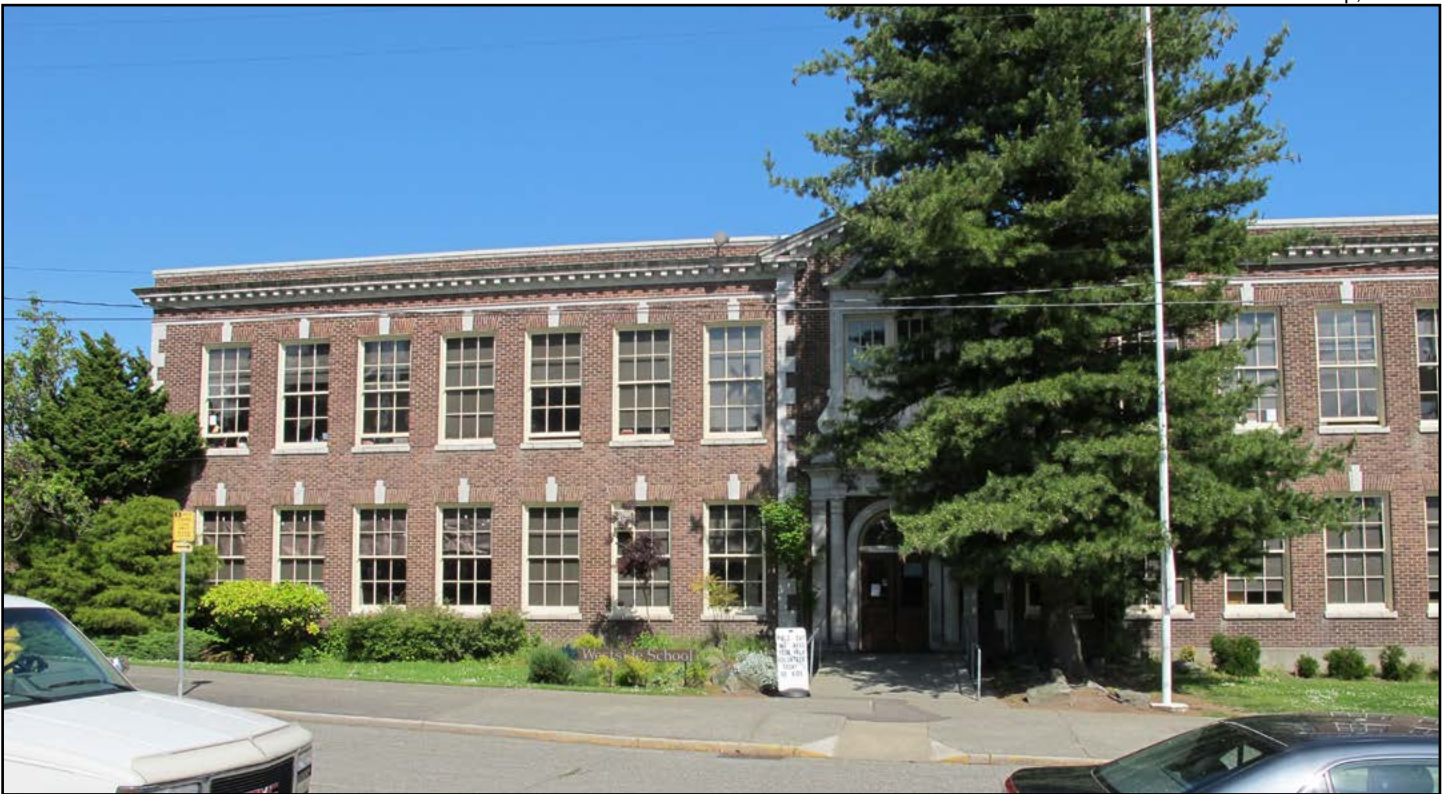
Figure 13. E.C. Hughes School, western façade, northern side
