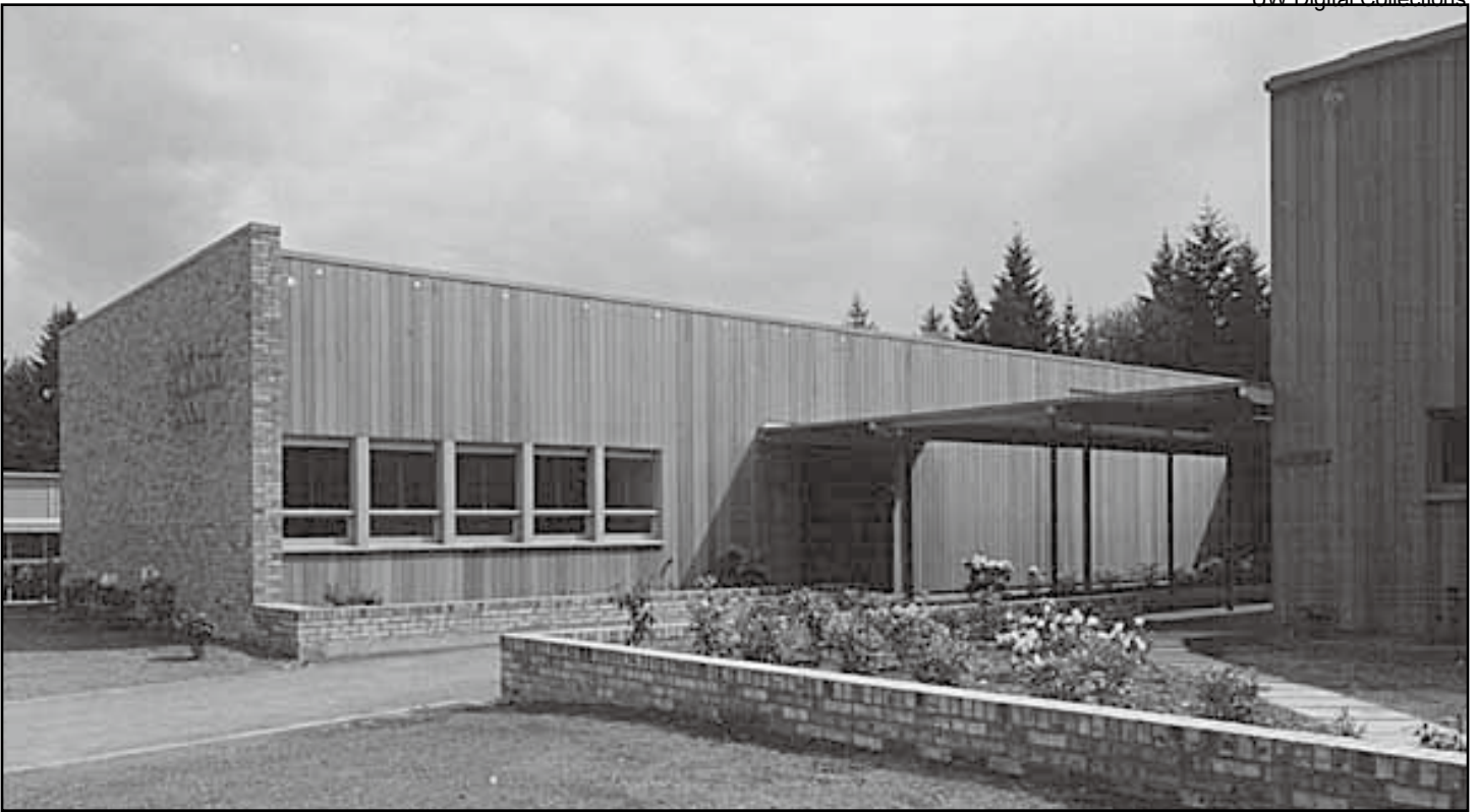
Figure 85. Clyde Hill Elementary School (1953, NBBJ)
