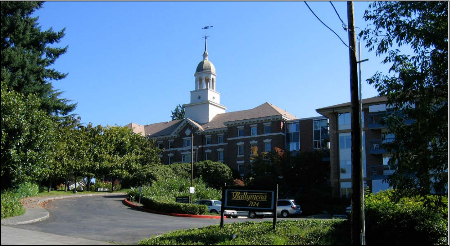
Figure 54. Seaview Building at The Kenney West Seattle (1908, Graham & Meyers)
