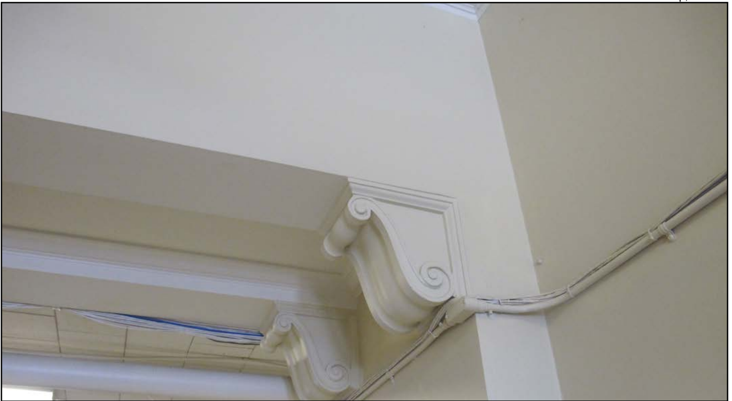
Figure 24. E.C. Hughes School, detail at entry interior
