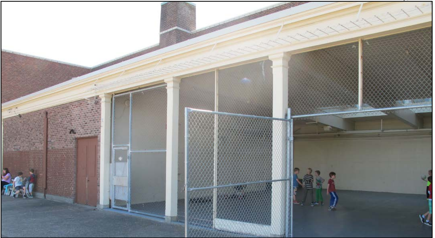
Figure 18. E.C. Hughes School, eastern façade, detail at covered playcourts
