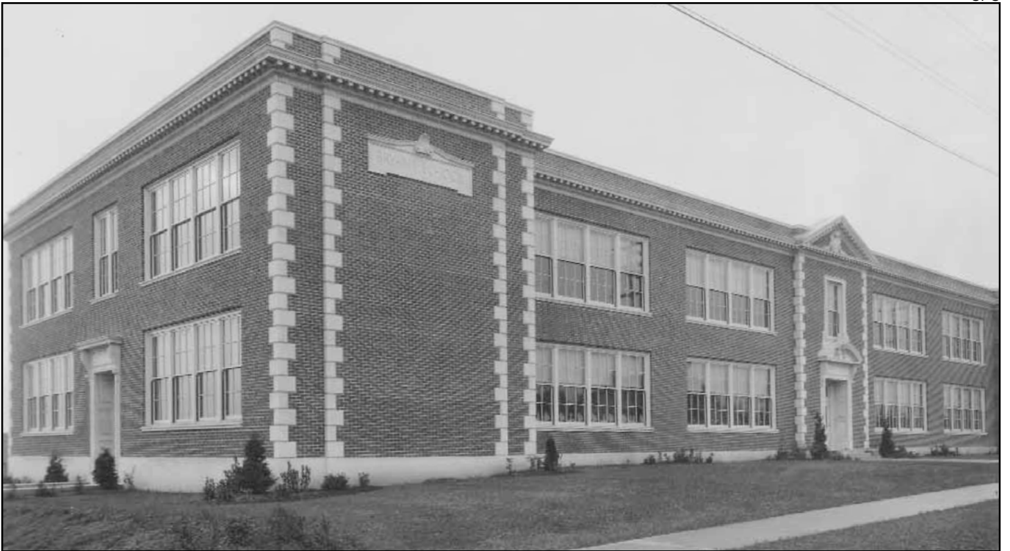
Figure 67. William Cullen Bryant School, 3311 NE 60th Street (1926, Floyd A. Naramore, altered, Seattle Landmark)
