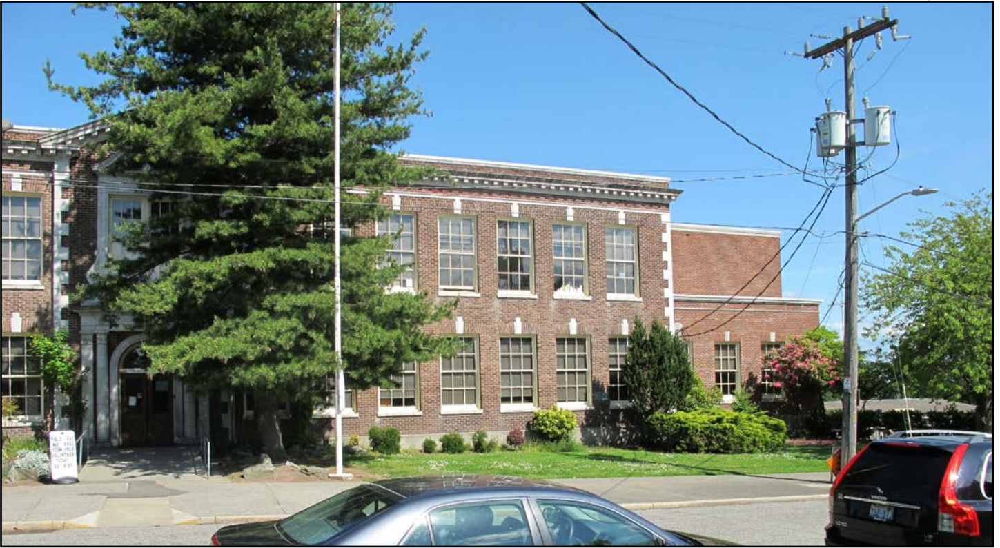
Figure 15. E.C. Hughes School, western façade, southern section
