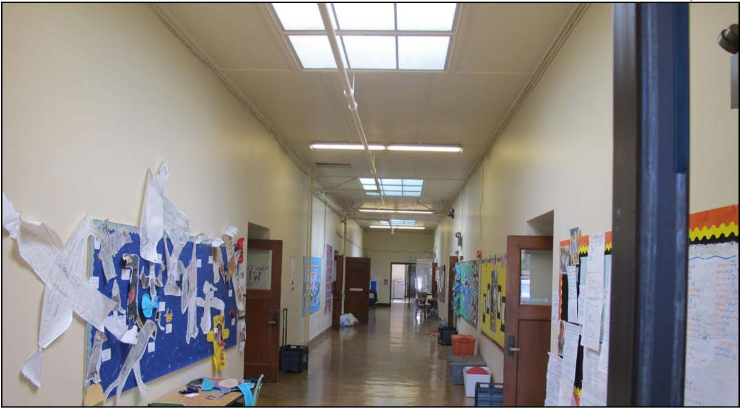
Figure 33. E.C. Hughes School, interior at upper floor hallway
