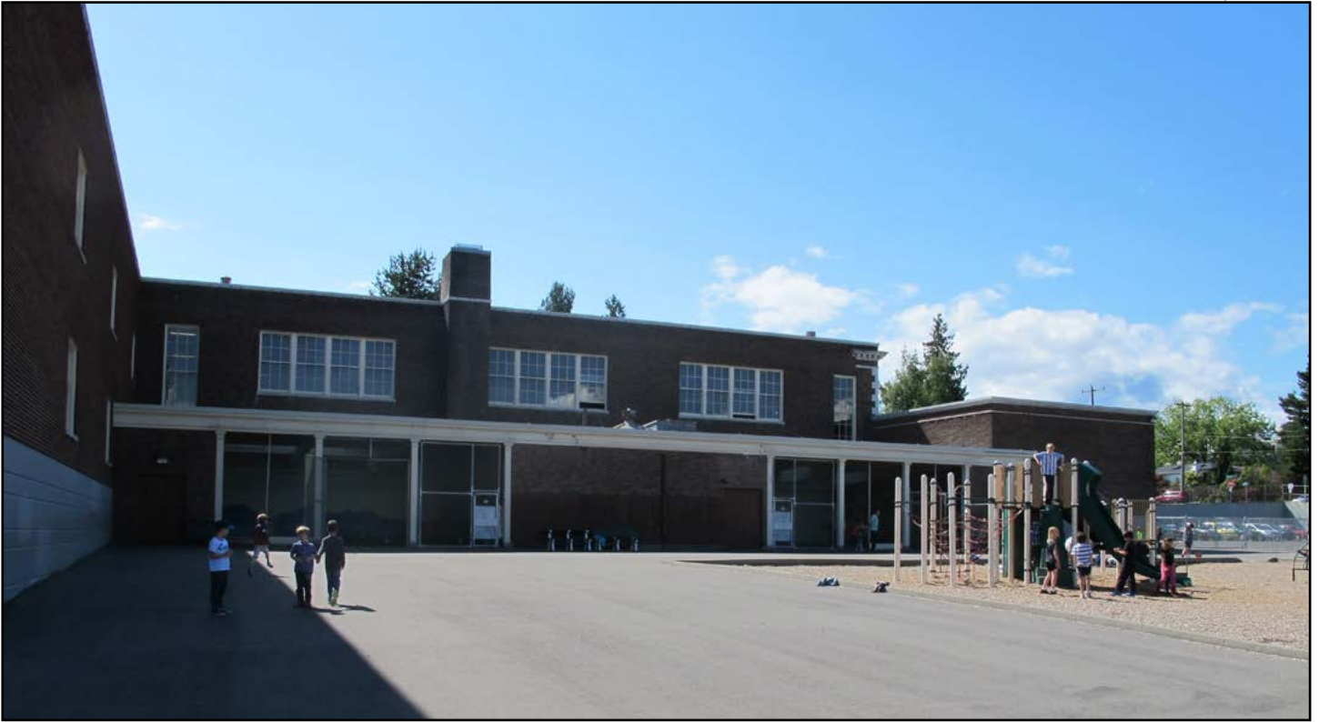
Figure 17. E.C. Hughes School, eastern façade at playcourts
