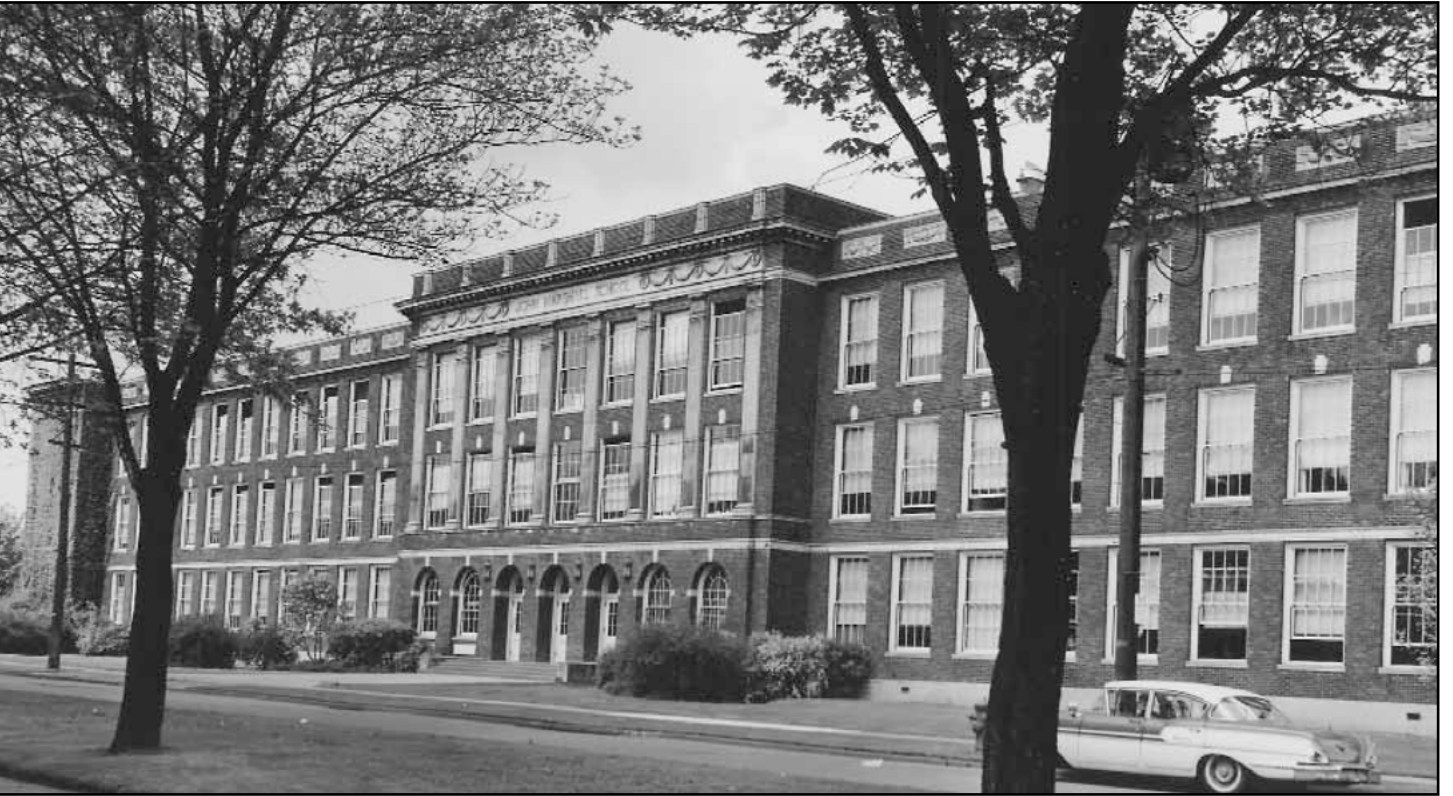
Figure 73. John Marshall Jr. High School, 520 NE Ravenna Boulevard (1927, Floyd A. Naramore)
