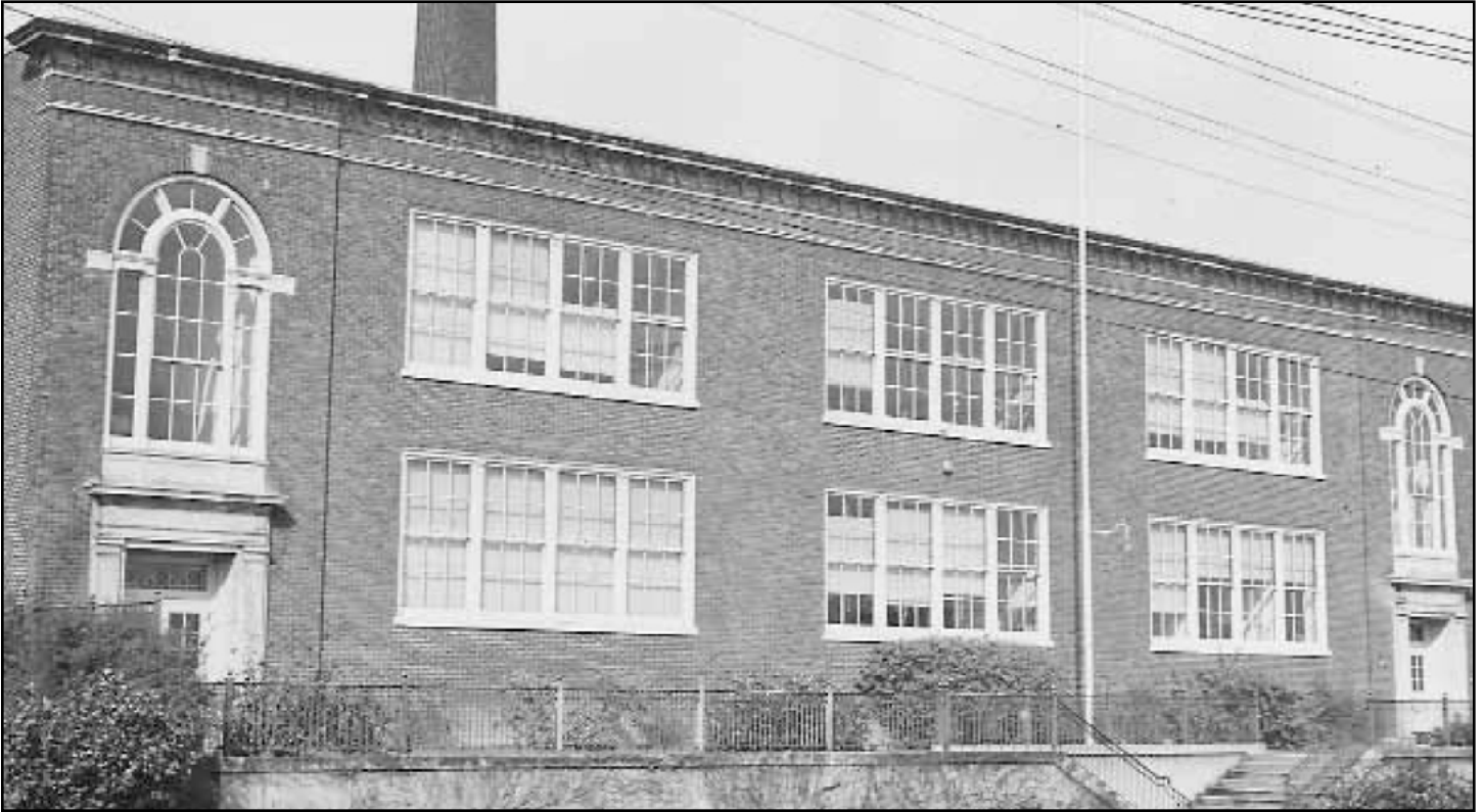
Figure 66. Montlake School, 2409 22nd Avenue E (1924, Floyd A. Naramore, Seattle Landmark)
