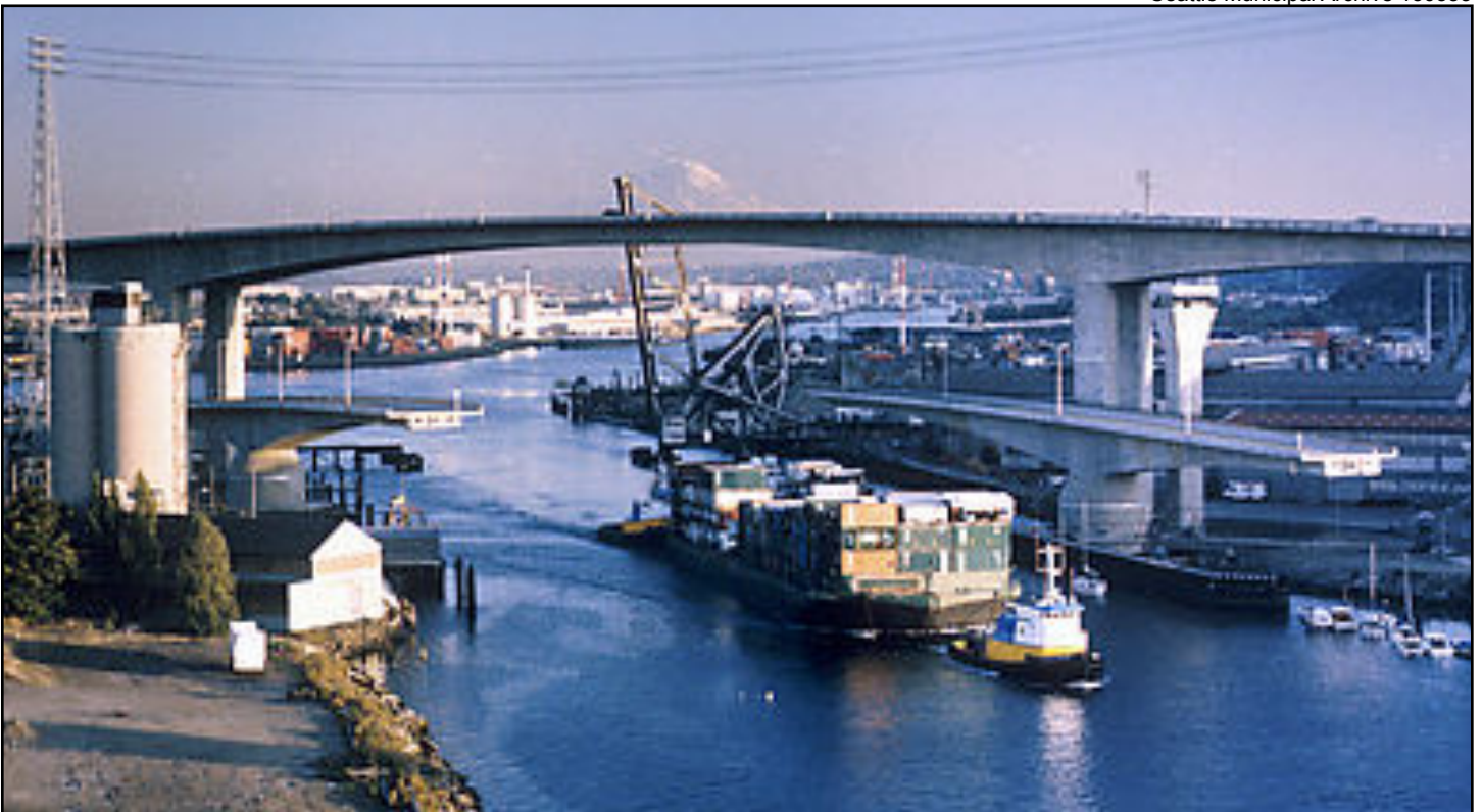
Figure 45. West Seattle Bridge, ca. 1984
