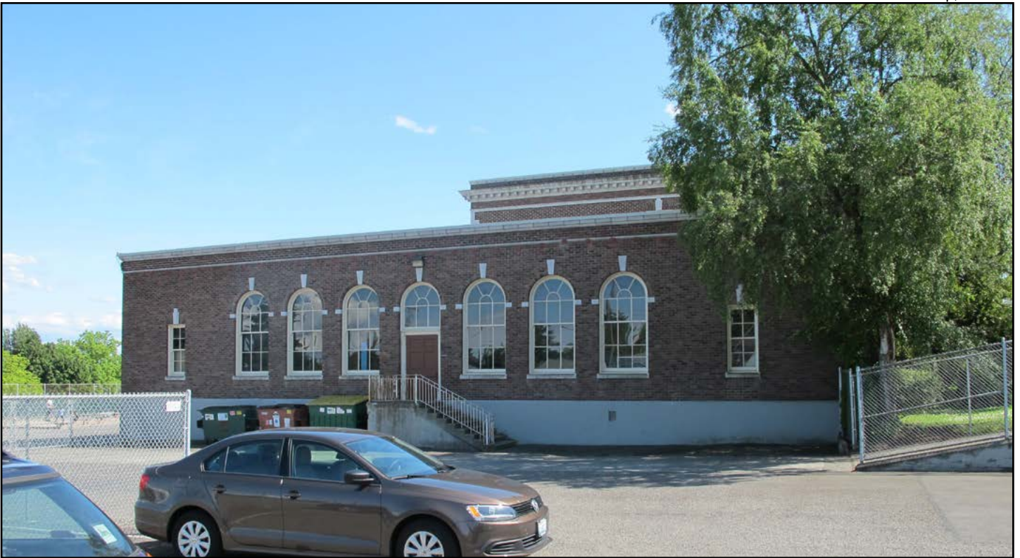
Figure 16. E.C. Hughes School, northern façade at auditorium
