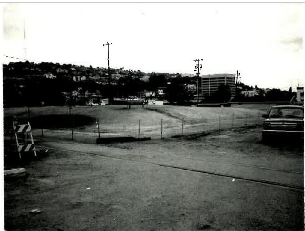
B25. Site of the former Belknap Glass building shortly after demolition, 1990. Source: King County Assessor.
