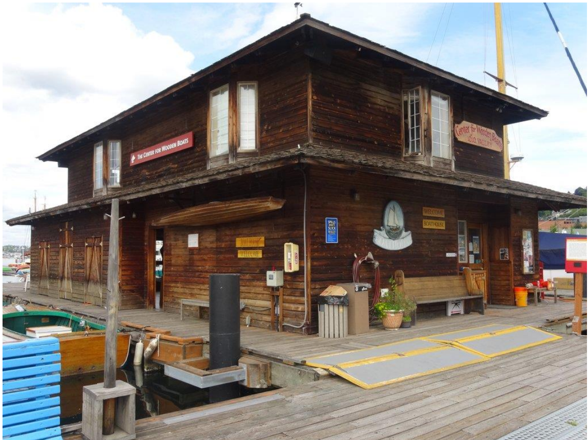
C19. Boathouse view of southwest corner; note the black steel piling in foreground, June 4, 2020
