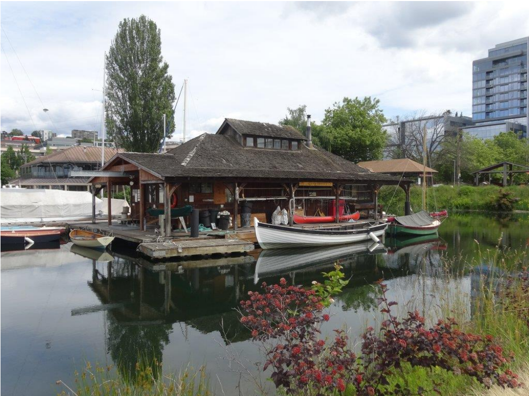
C13. View of north side of boat shop, showing gantry and sliding doors, view south, June 4, 2020
