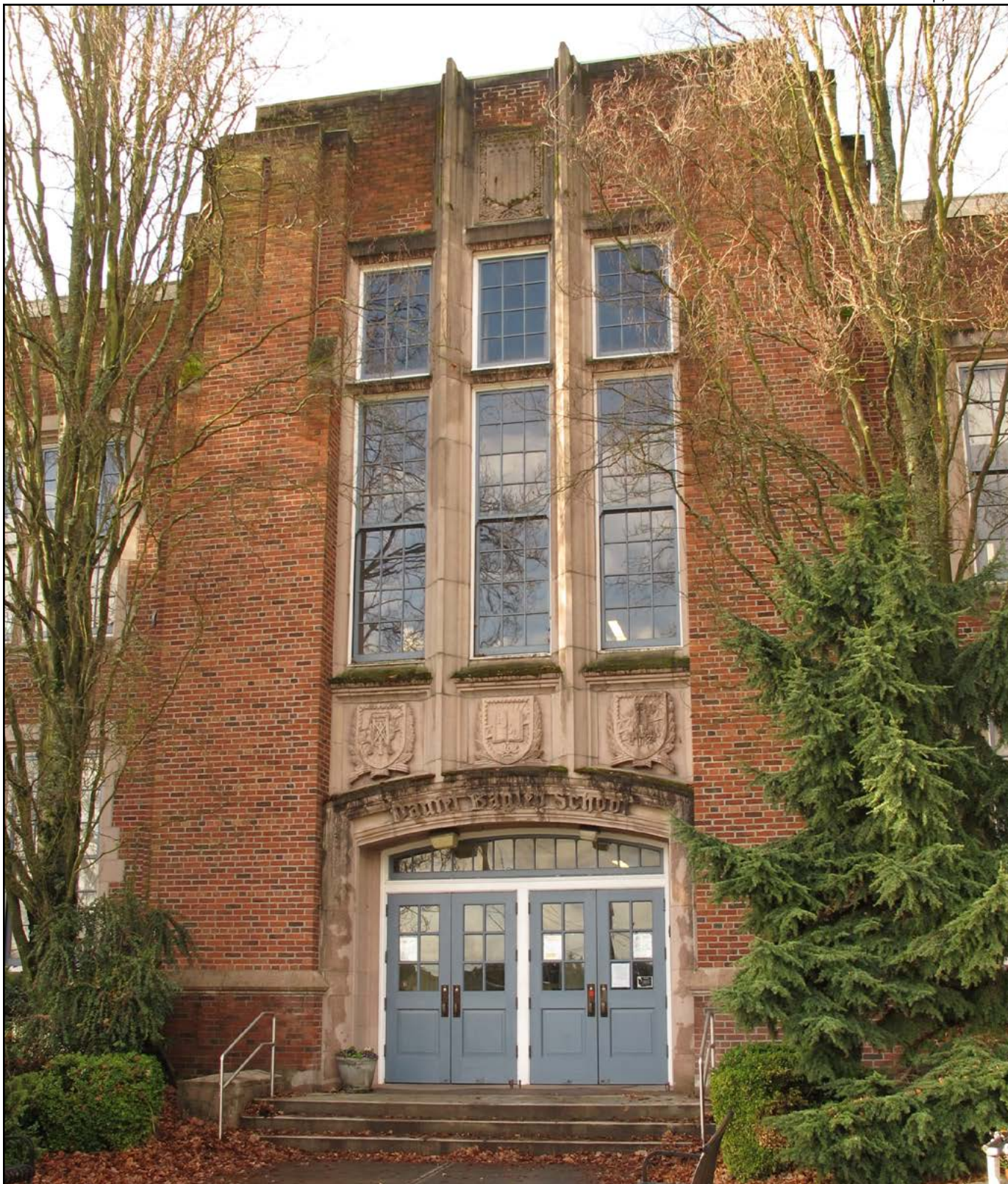
Figure 11. Daniel Bagley School, entry bay, eastern façade
