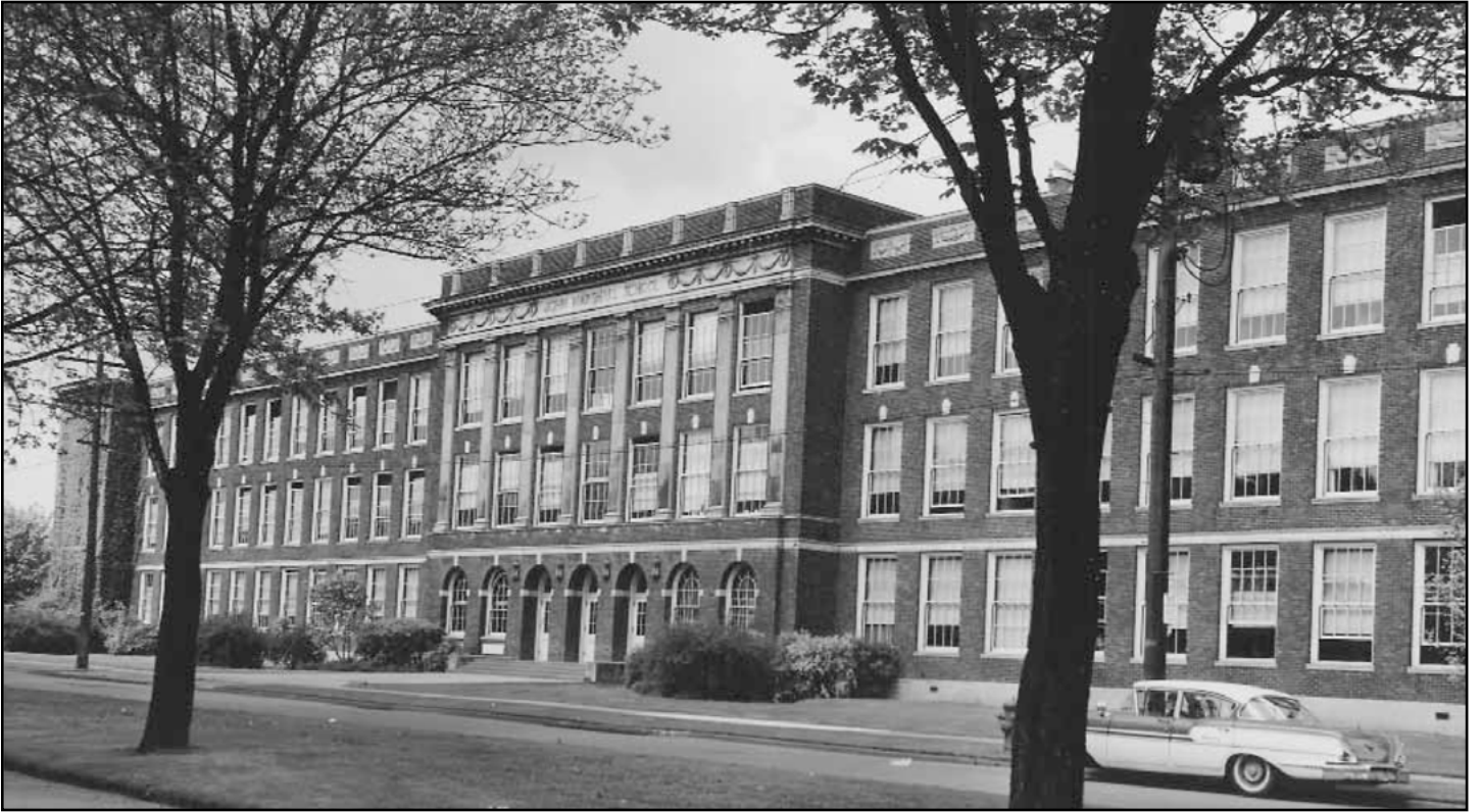
Figure 93. John Marshall Jr. High School, 520 NE Ravenna Boulevard (1927, Floyd A. Naramore)
