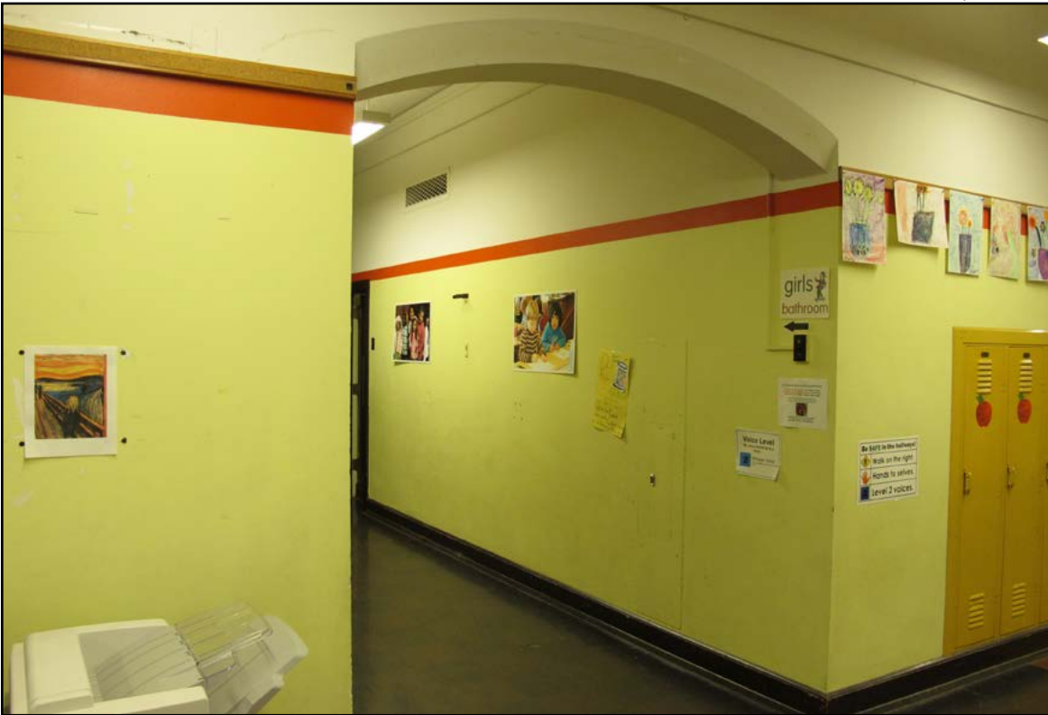
Figure 28. Arched opening at intersection of hallways
