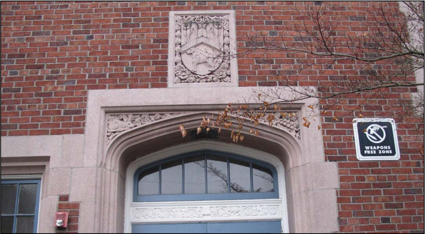
Figure 16. Daniel Bagley School, northern façade entry details
