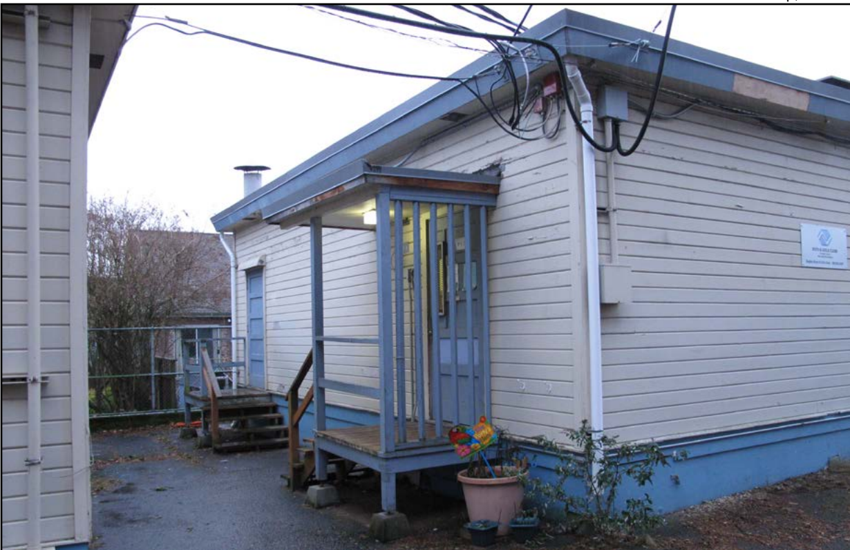
Figure 37. Temporary building entrance
