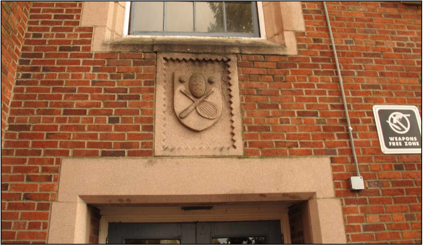
Figure 22. Daniel Bagley School, detail of western façade entrance
