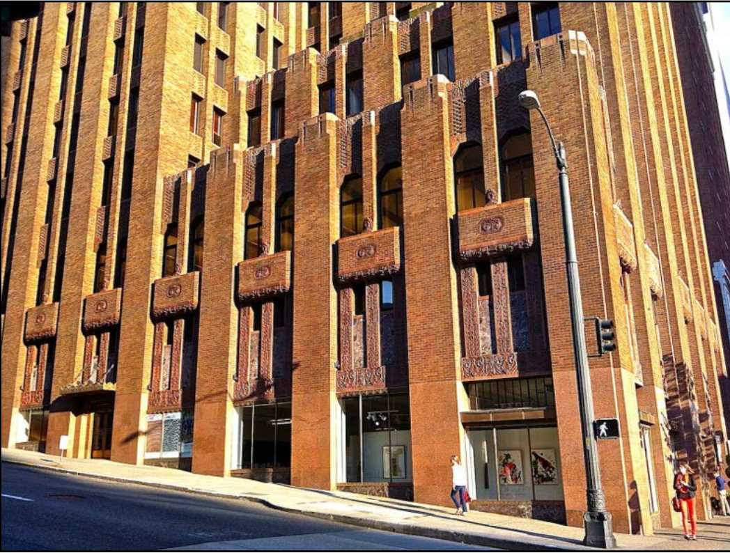
Figure 77. The Seattle Tower, Seattle (1928, Albertson, Wilson & Richardson, City of Seattle Landmark)
