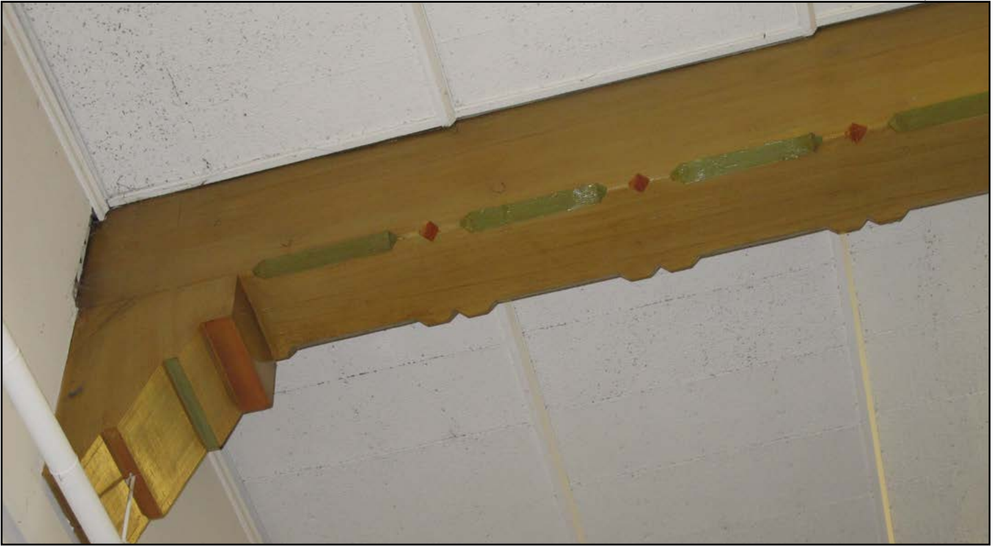
Figure 30. Detail of beams in meeting room
