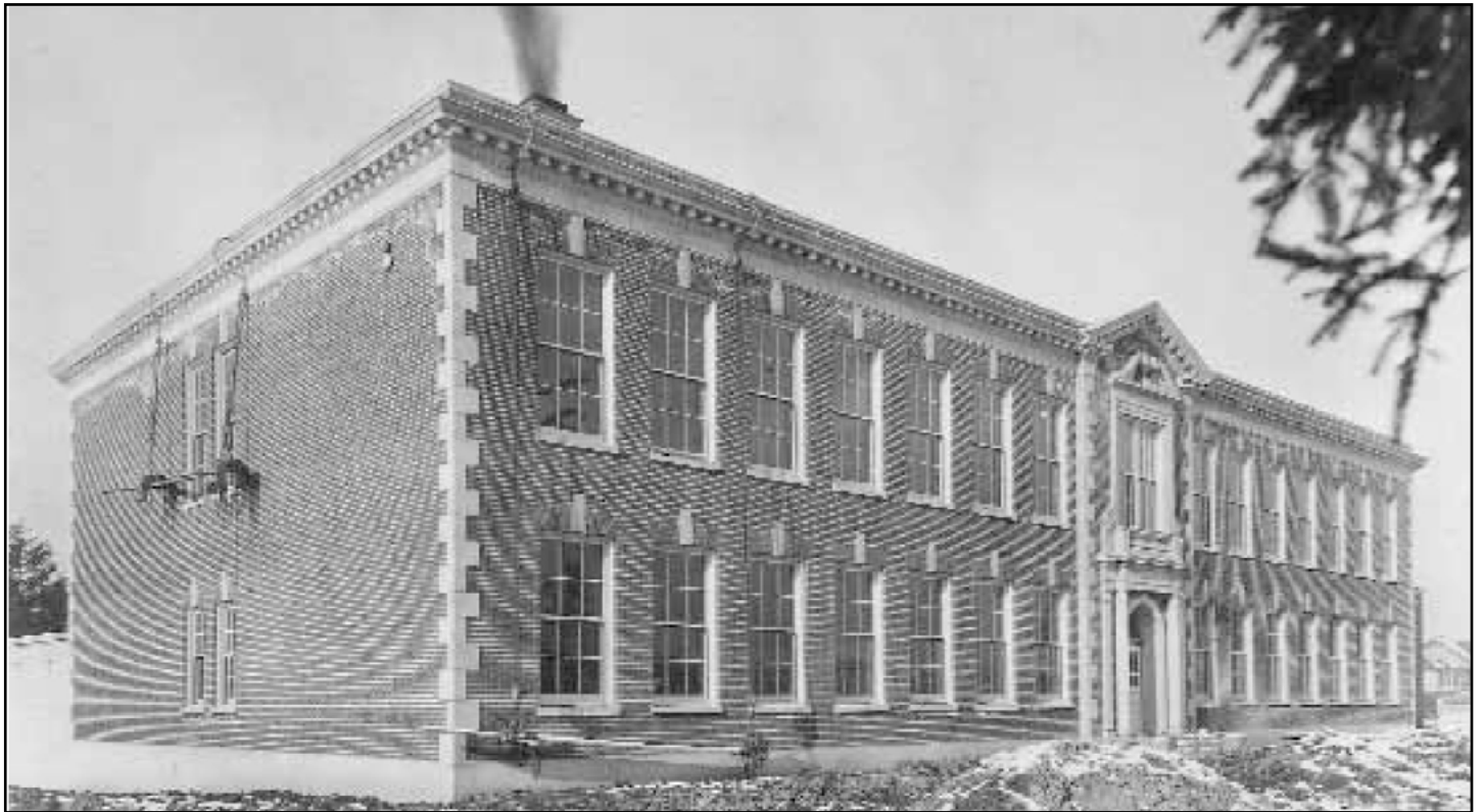
Figure 86. Dunlap School, 8621 46th Avenue S (1924, Floyd A. Naramore, Seattle Landmark)
