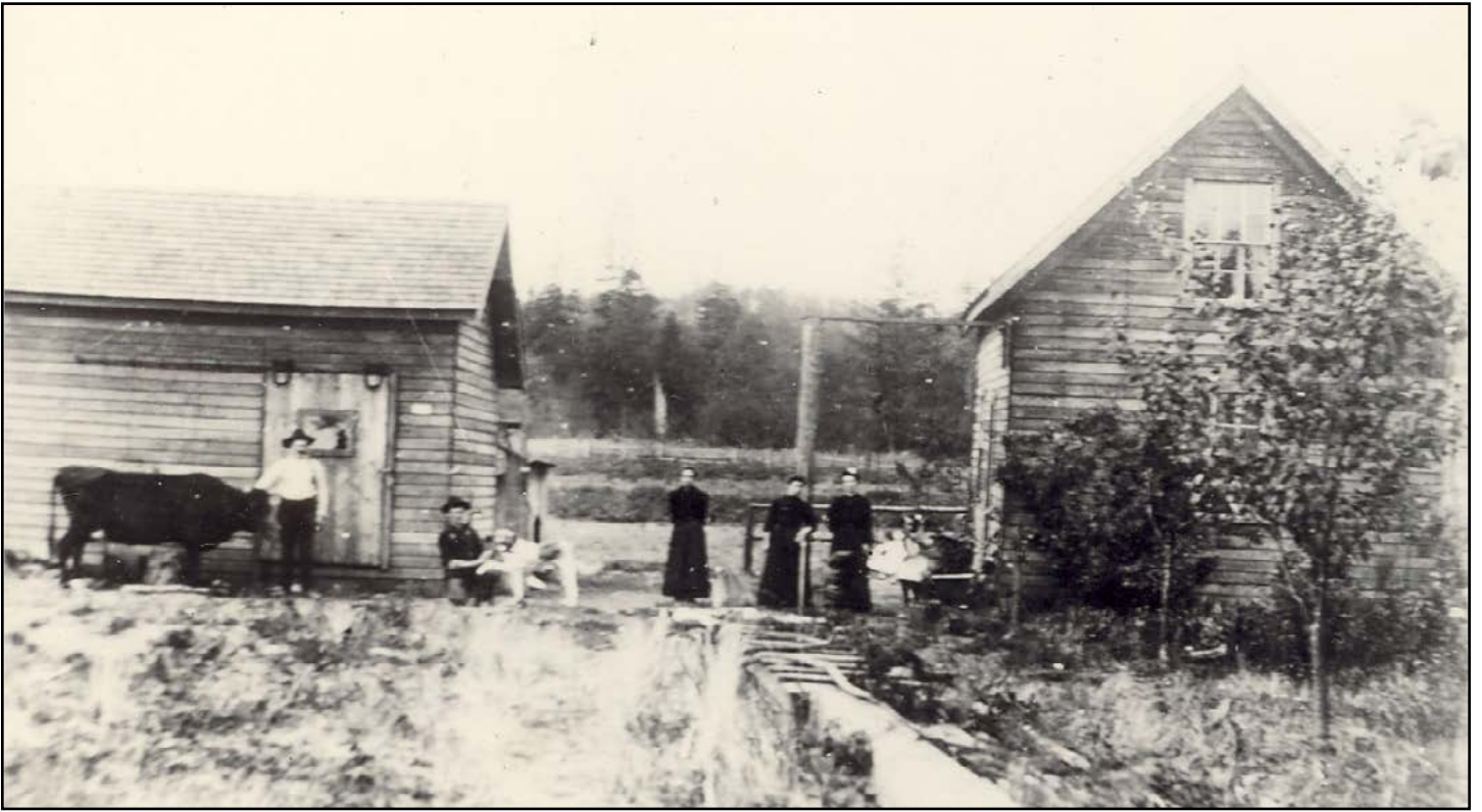
Figure 60. Allen Annex, ca. 1900
