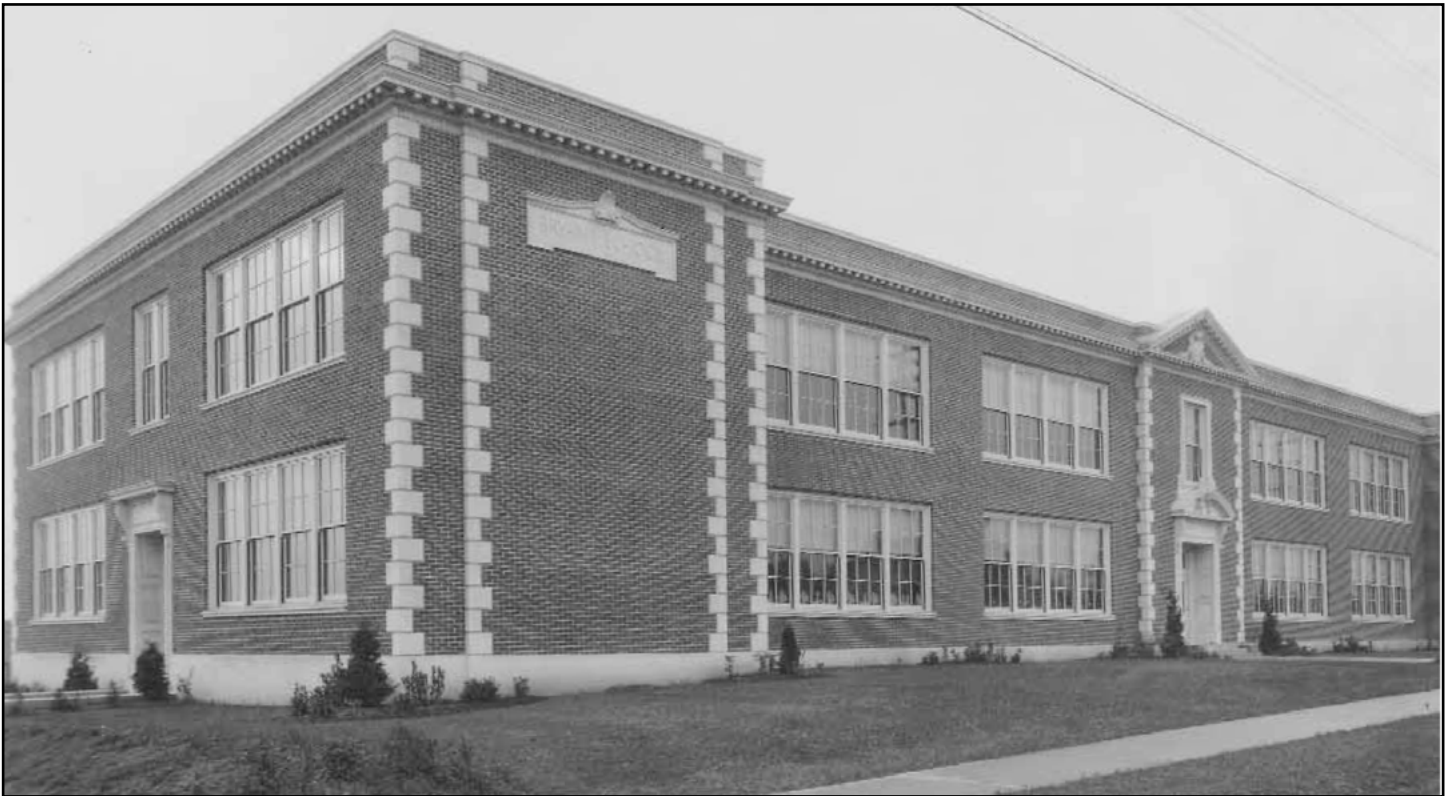
Figure 88. William Cullen Bryant School, 3311 NE 60th Street (1926, Floyd A. Naramore, altered, Seattle Landmark)
