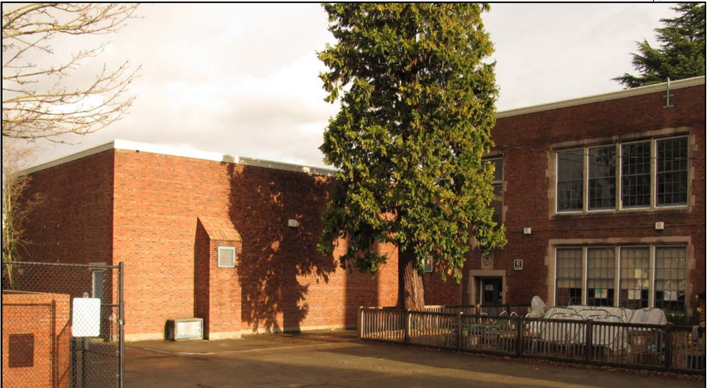
Figure 21. Daniel Bagley School, southern façade of northern wing
