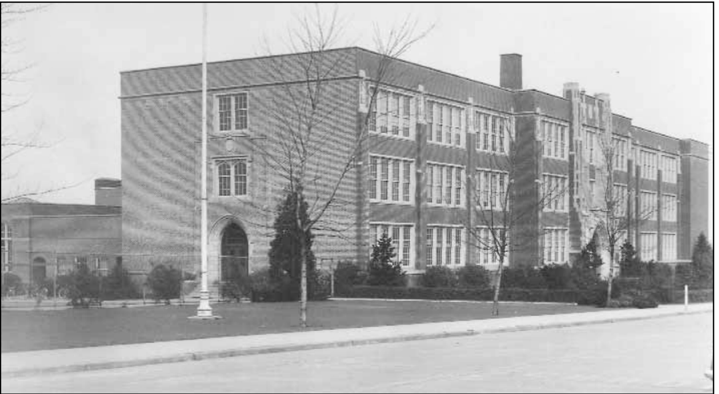
Figure 94. Madison Jr. High School, 3429 45th Avenue SW (1929 Floyd A. Naramore, Seattle Landmark)
