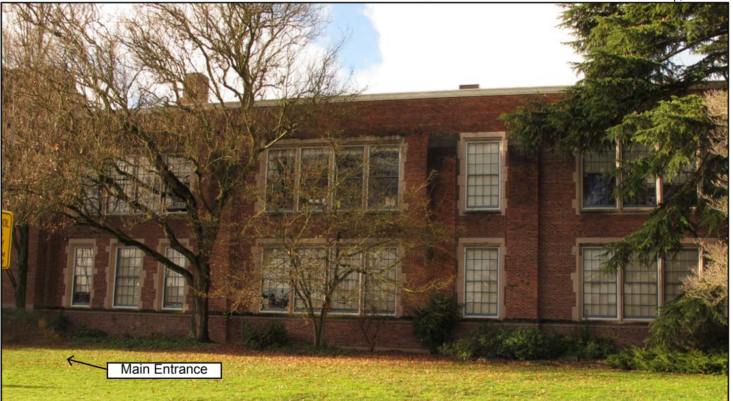
Figure 10. Daniel Bagley School, eastern façade
