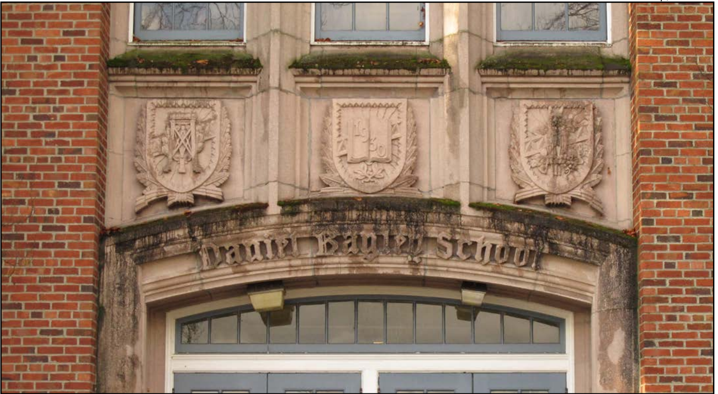
Figure 12. Daniel Bagley School, detail of transom, casing, and spandrel at main entry
