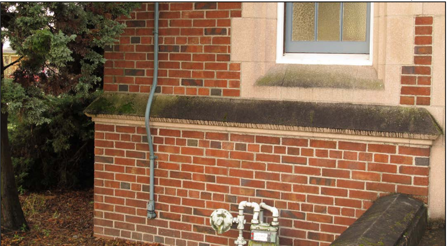
Figure 17. Daniel Bagley School, water table on northeastern corner
