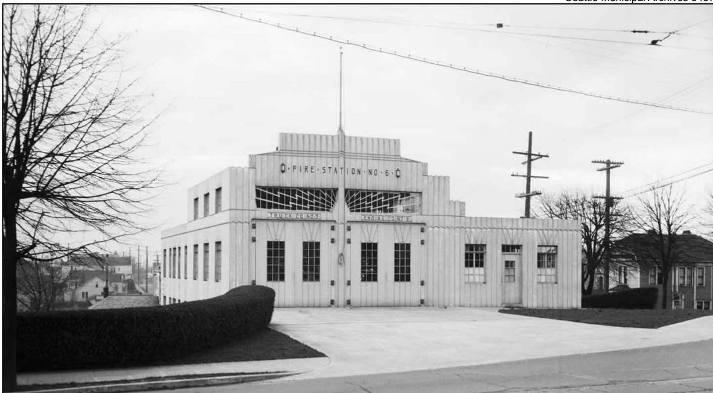
Figure 76. Fire Station #6, Seattle (1931, George Stewart, City of Seattle Landmark)
