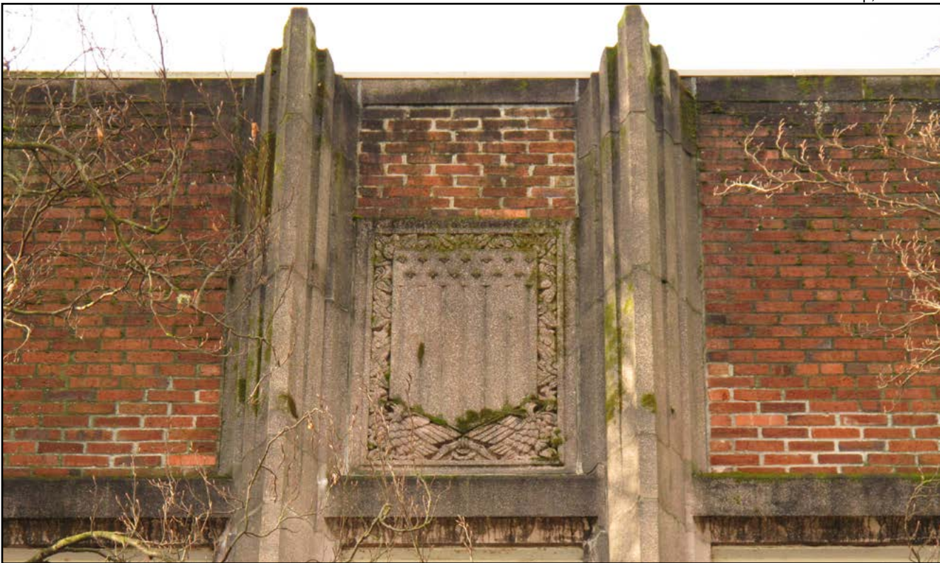
Figure 13. Daniel Bagley School, cast stone shield and parapet
