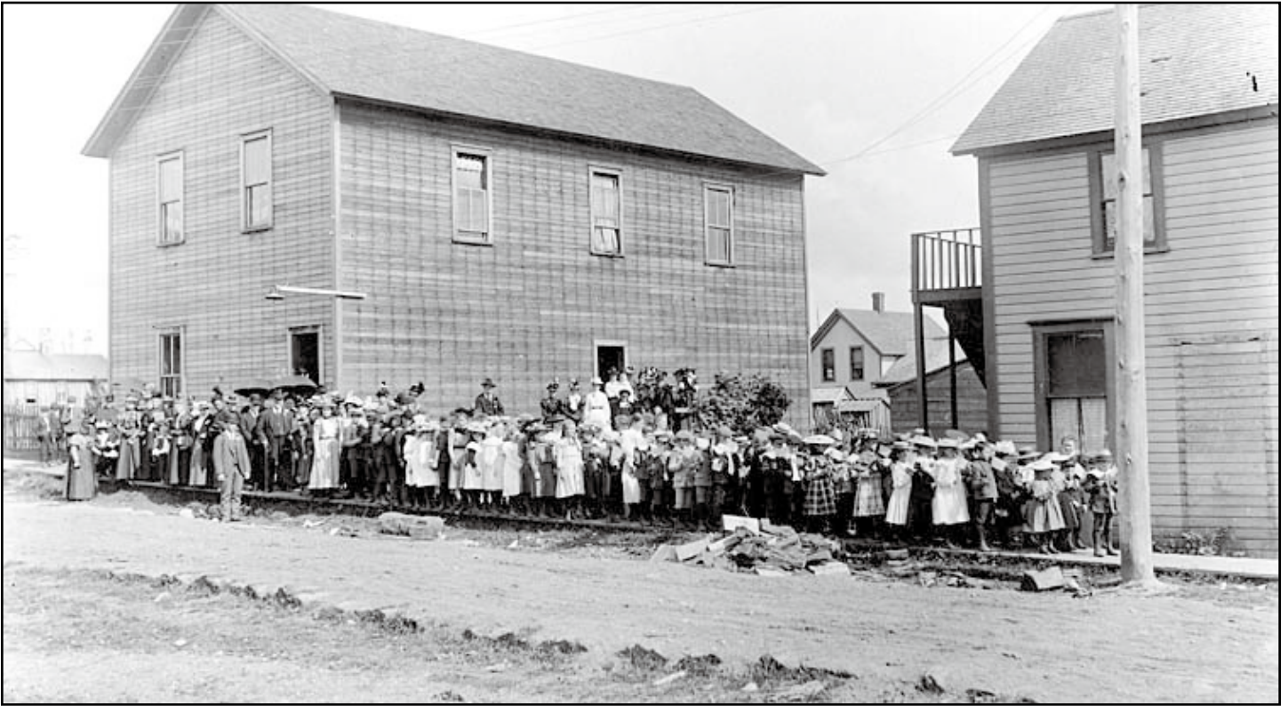
Figure 47. Green Lake School annex in the Independent Order of Good Templars Hall, 1897
