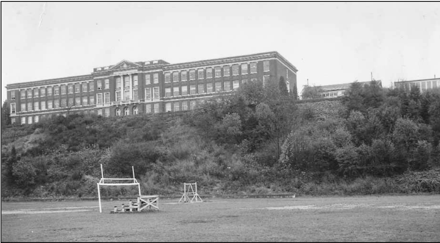
Figure 98. Cleveland High School, 5511 15th Avenue S (1927 Floyd A. Naramore, altered, Seattle Landmark)
