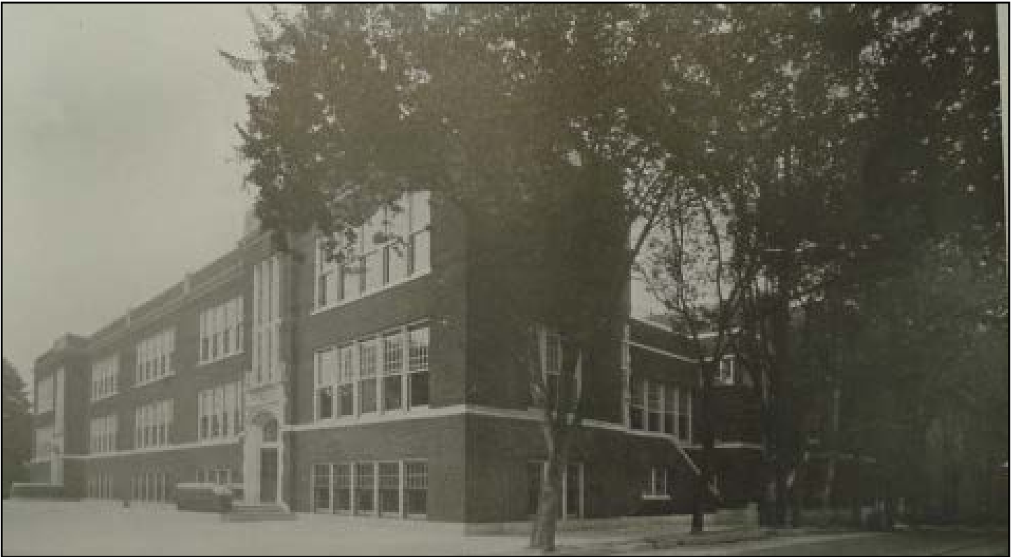
Figure 100. Couch Elementary School, Portland Oregon (1914-1915 Floyd Naramore, altered)
