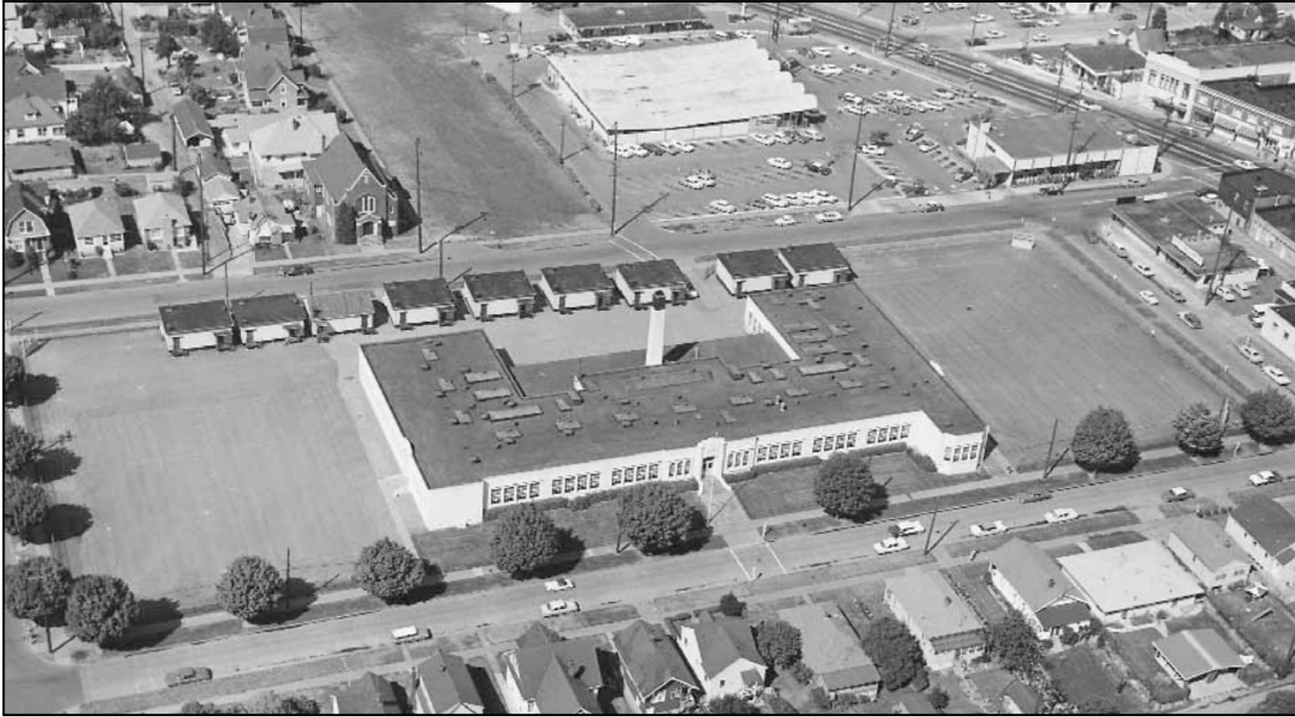
Figure 84. Columbia School, 3528 S Ferdinand Street (1922, Floyd A. Naramore)
