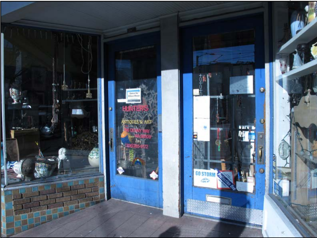
Figure 18. 104 Denny Way building, southern façade, entrance at 106 Denny Way
