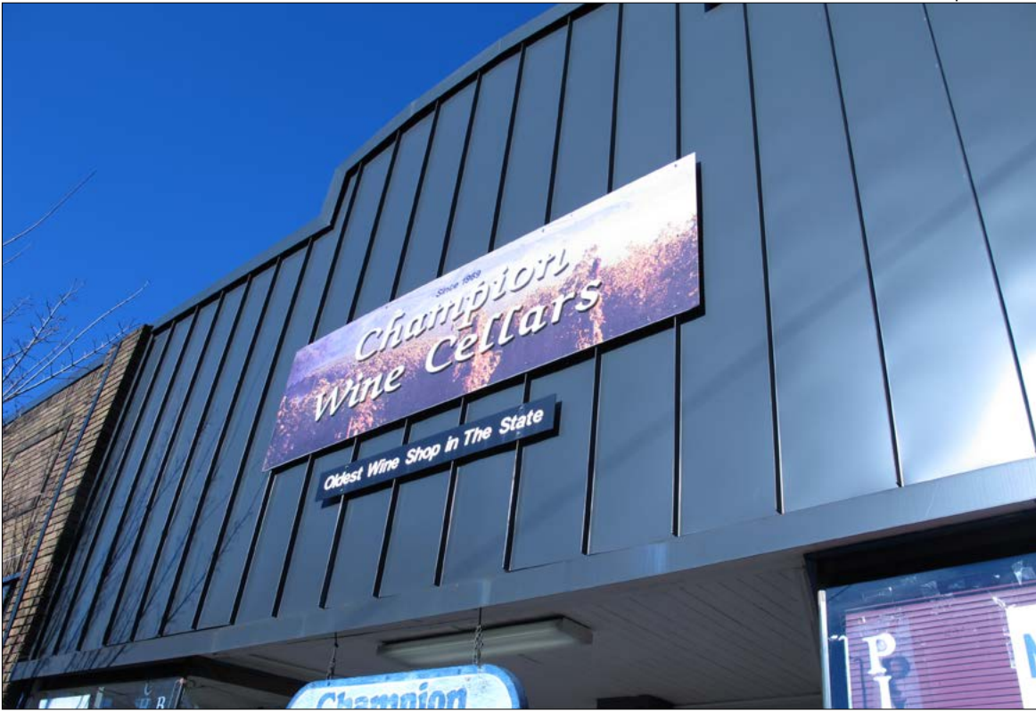
Figure 21. 104 Denny Way building, southern façade, aluminum parapet at 108 Denny Way
