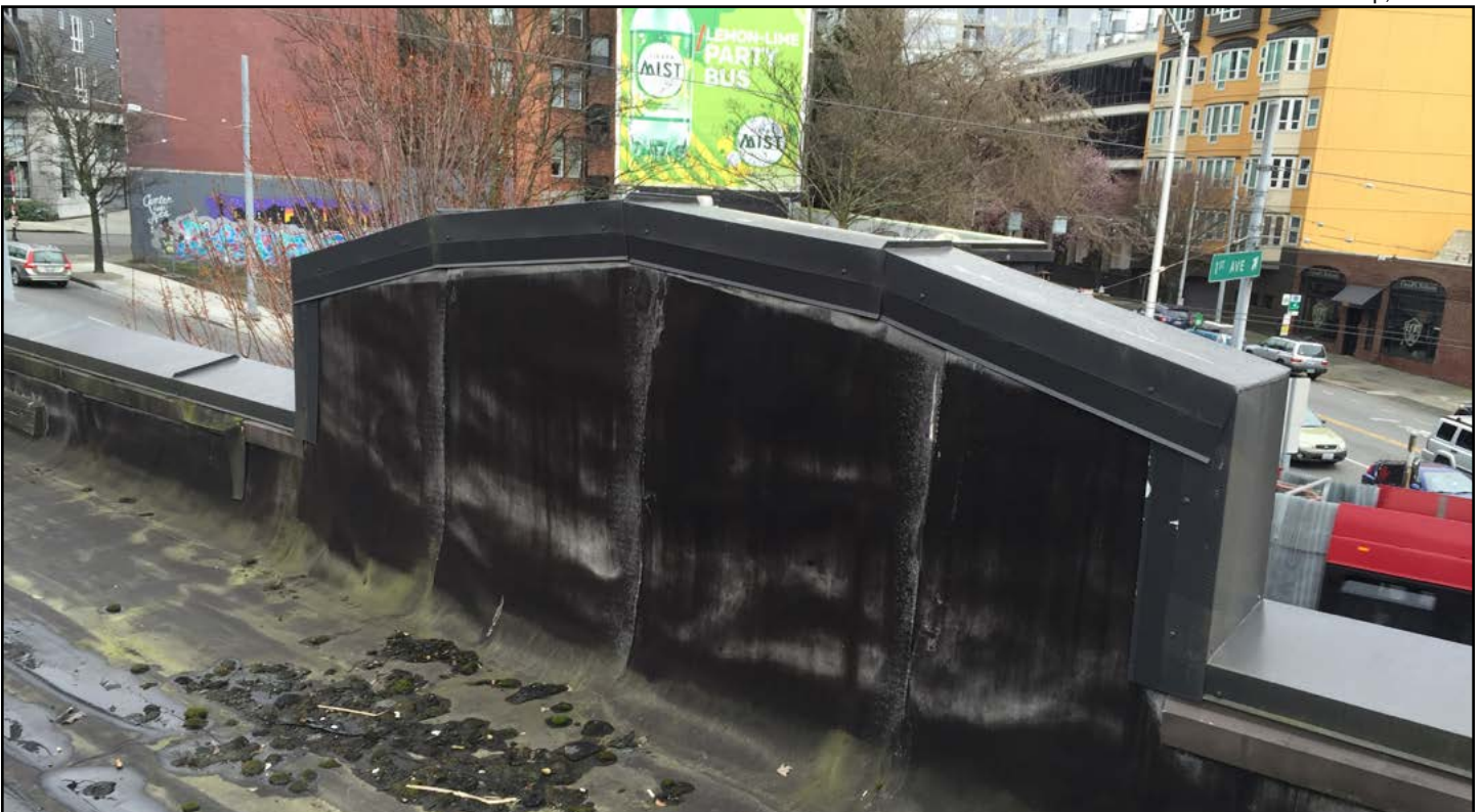
Figure 34. 104 Denny Way building, detail at parapet above 108 Denny Way
