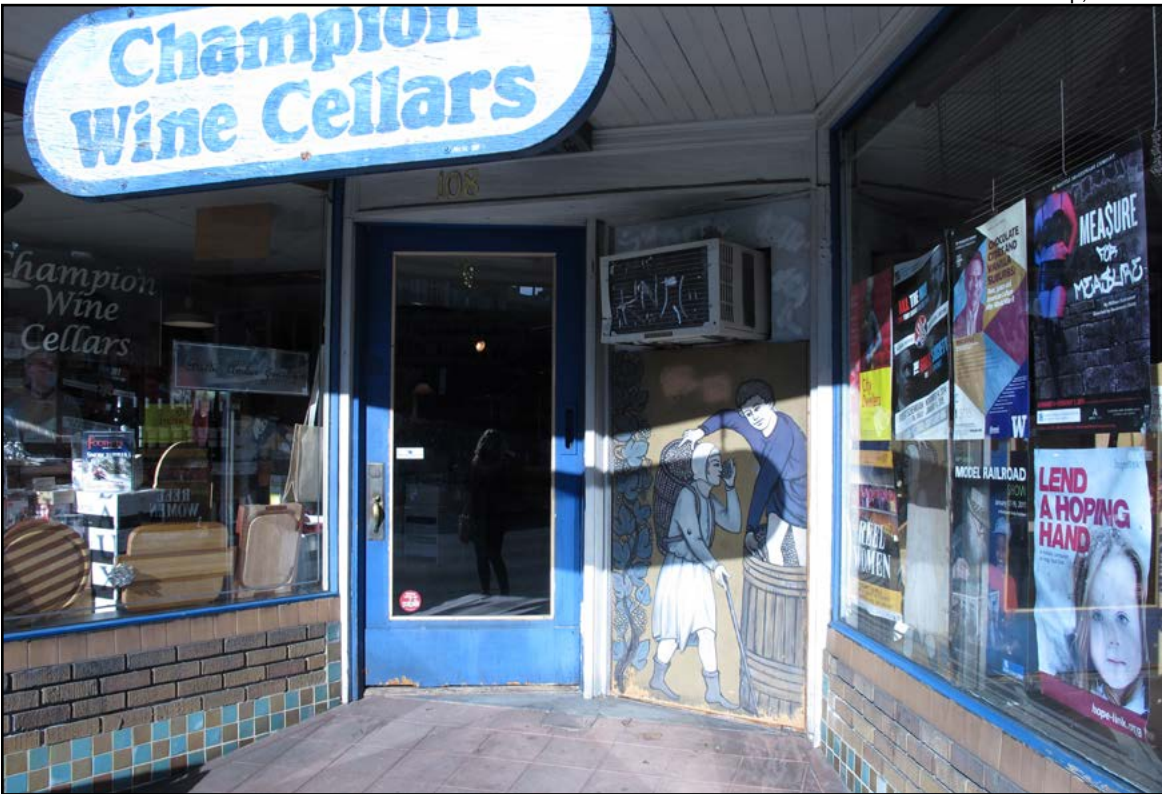
Figure 20. 104 Denny Way building, southern façade, entrance at 108 Denny Way
