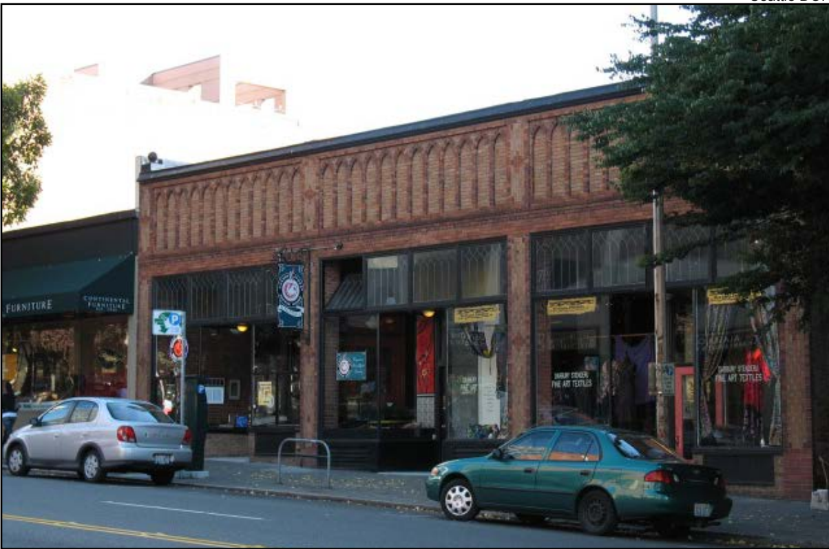
Figure 50. The Colsky Building, 2121 First Avenue (1926, James E. Blackwell)
