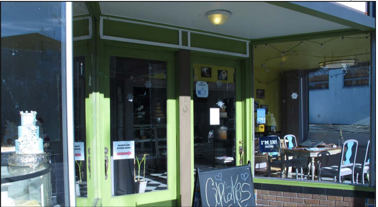
Figure 22. 104 Denny Way building, southern façade, entrance at 110 Denny Way
