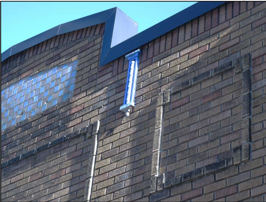
Figure 12. 104 Denny Way building, western façade, detail at parapet
