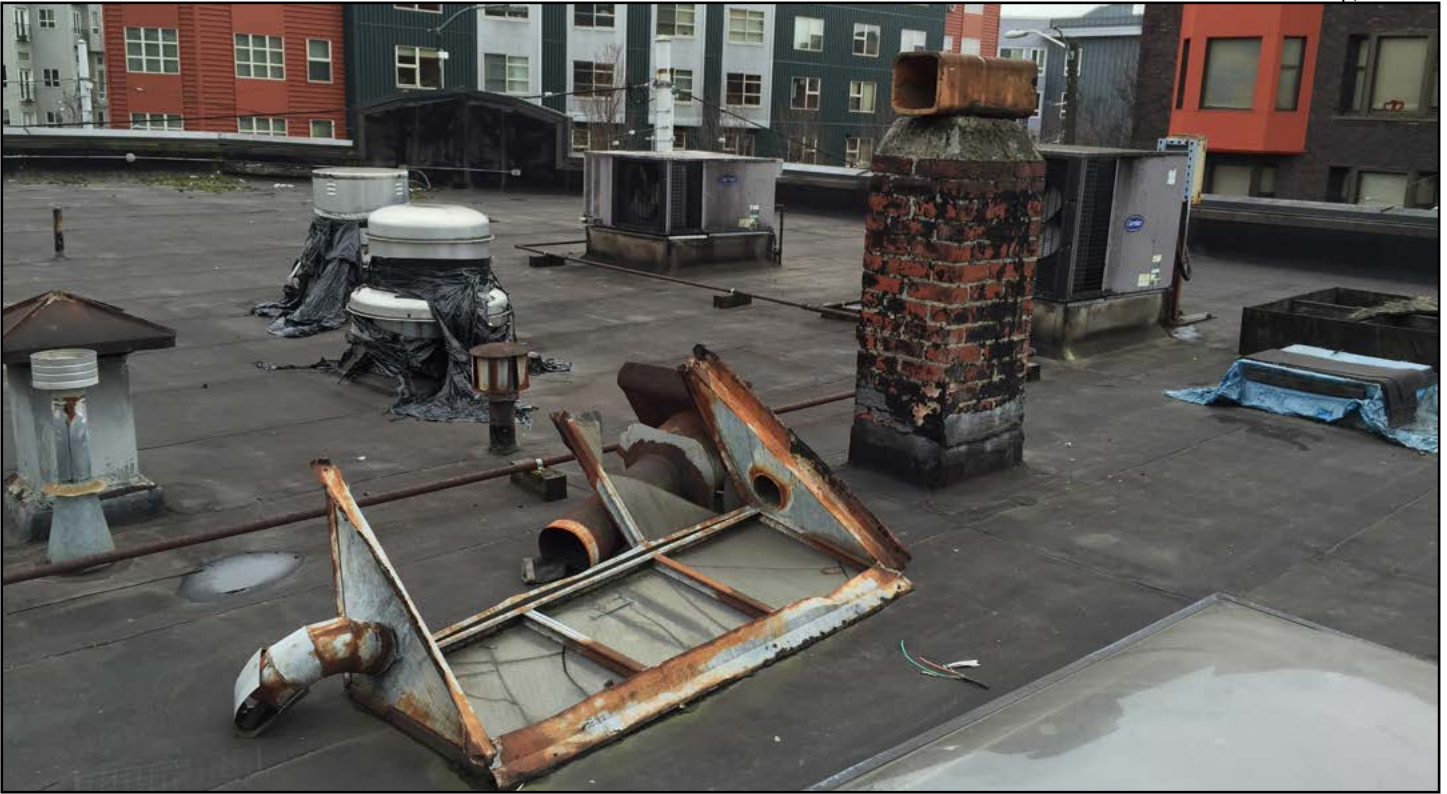
Figure 33. 104 Denny Way building, roof viewing southwest
