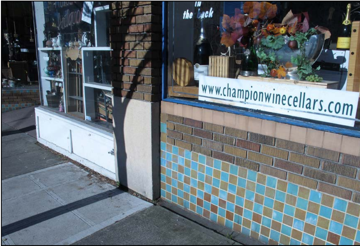
Figure 19. 104 Denny Way building, southern façade, tile and panel detail
