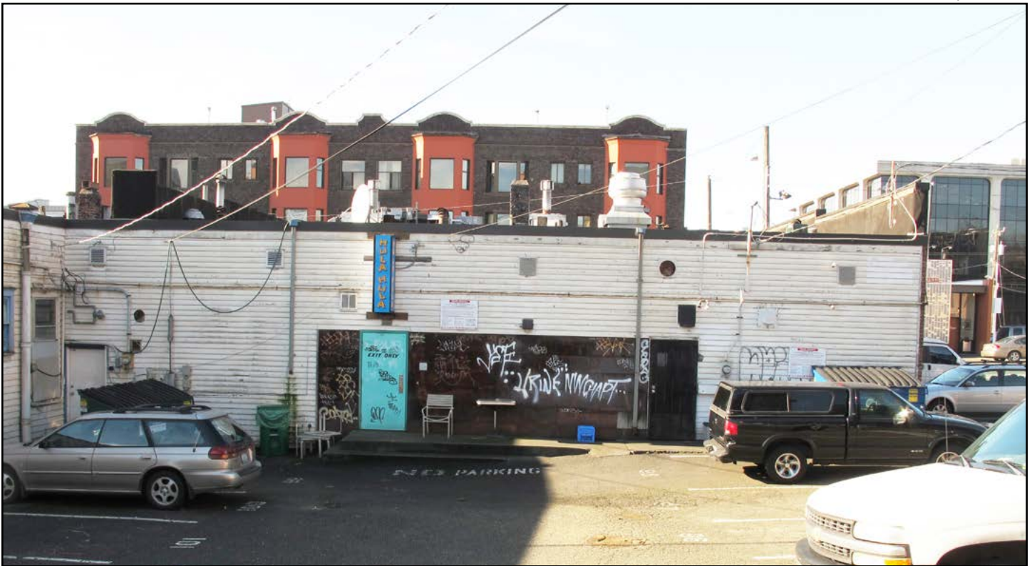
Figure 24. 104 Denny Way building, northern façade at parking lot
