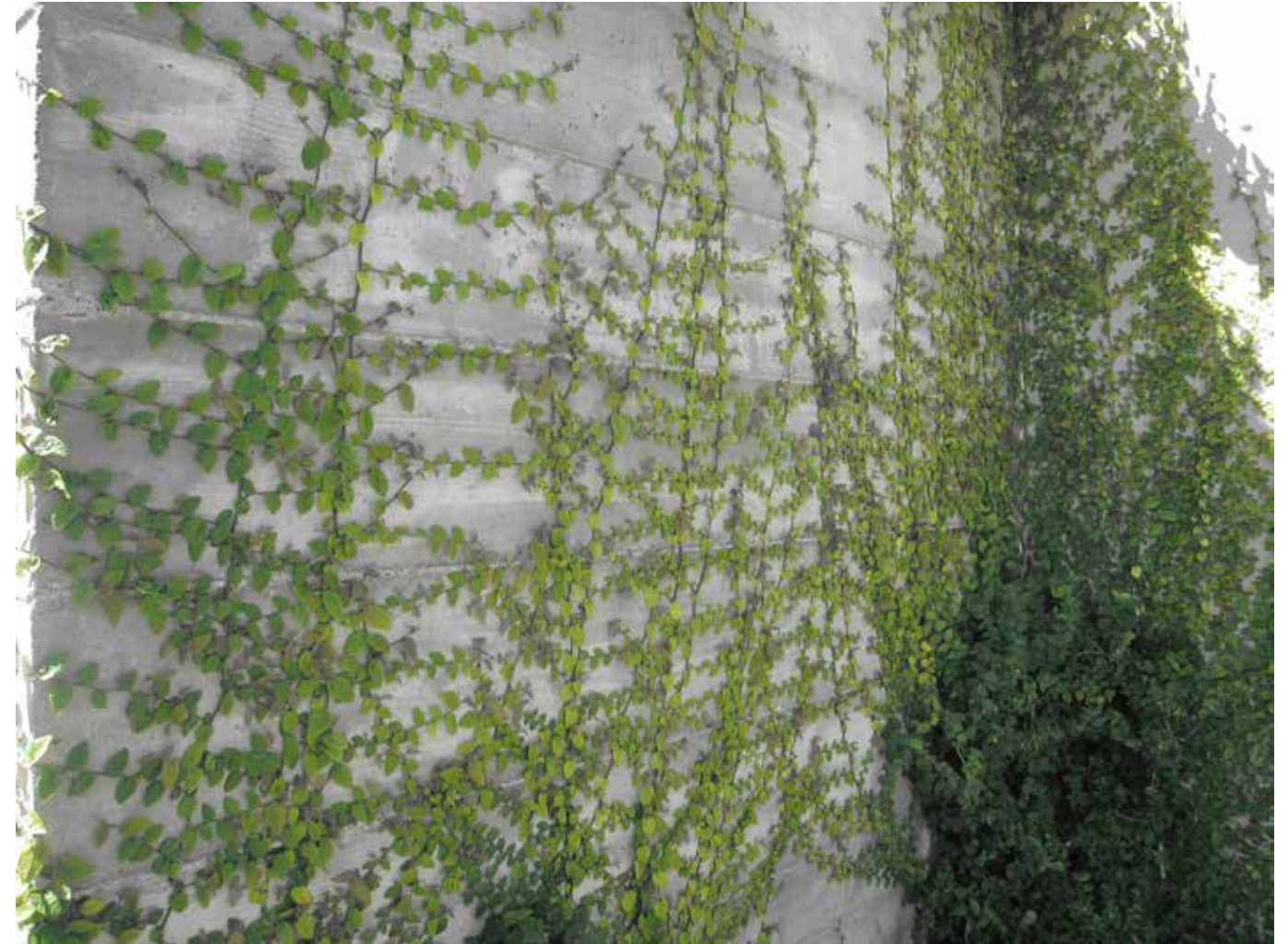
OVER TIME NORTH FACE GREEN TRELLIS PLANTS ARE ANTICIPATED TO GROW OVER TO SOUTH FACE OF WALL.
