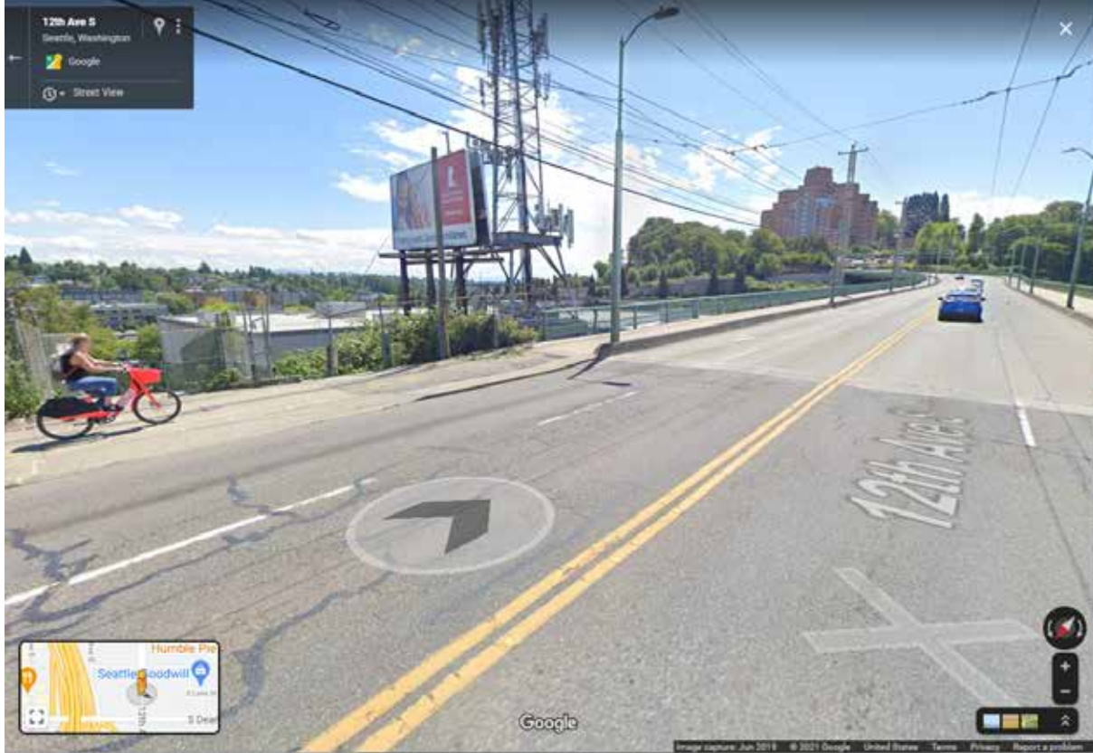
CONCRETE FENCES VISIBLE ACROSS BRIDGE.
