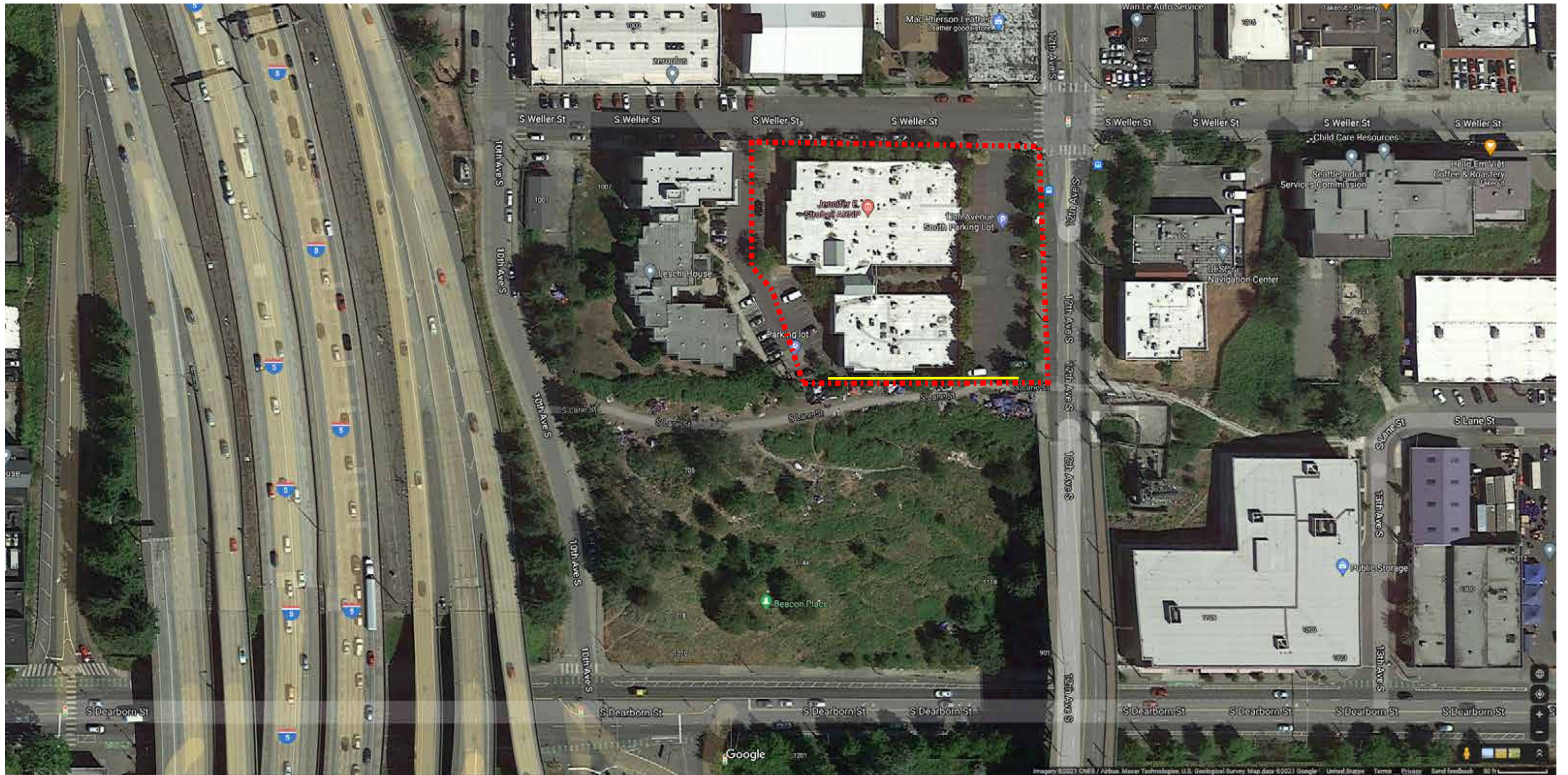
AERIAL SITE VIEW
