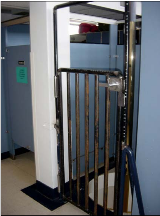
Above left, detail of the security gate at the top of the fire pole. Above right, detail of Second Floor Locker Room flooring. Black concrete delineates the edge of an original open well to the Apparatus Room below, which has been infilled with concrete slab to create a larger Locker Room.
