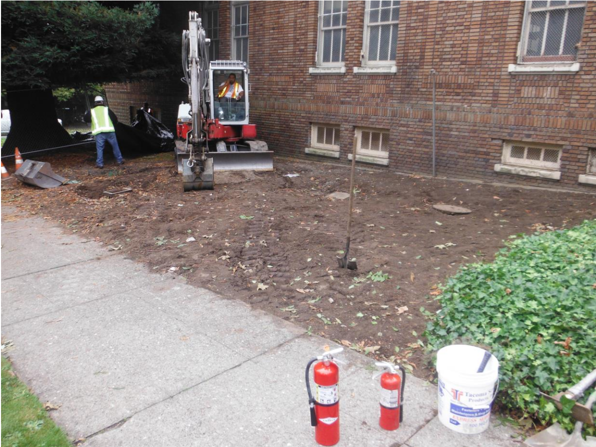
Location of 2 USTs along north exterior of building.
